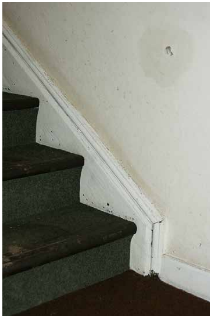
Plate 116: Roll beaded skirting on staircase
