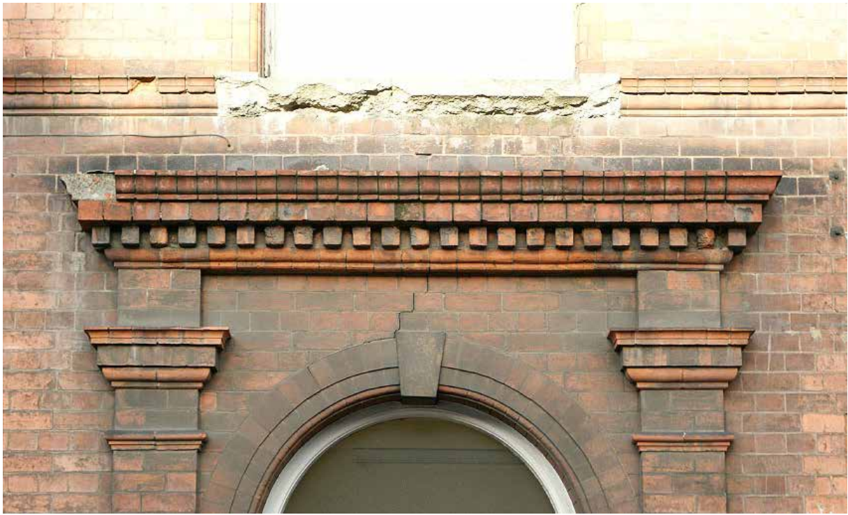
Plate 104: Dentilated cornice and terracotta pediment to front entrance
