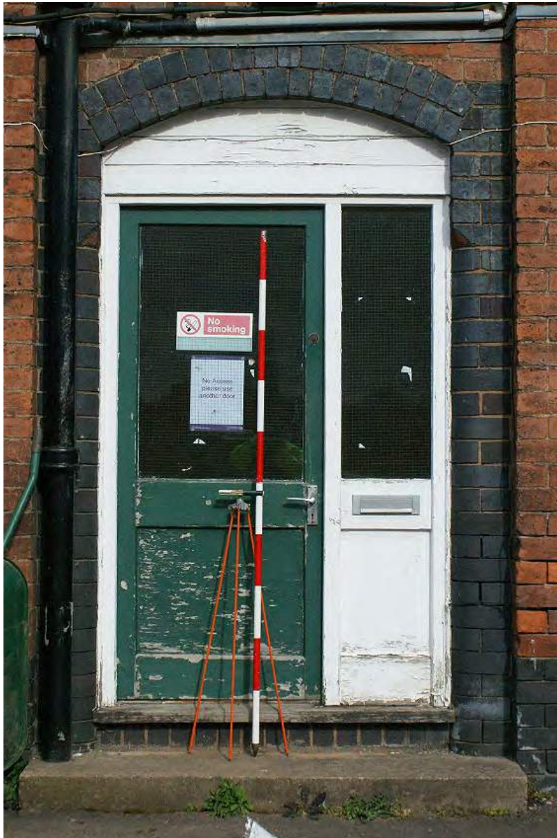
Plate 100: Blue brick door surround of two-storey range
