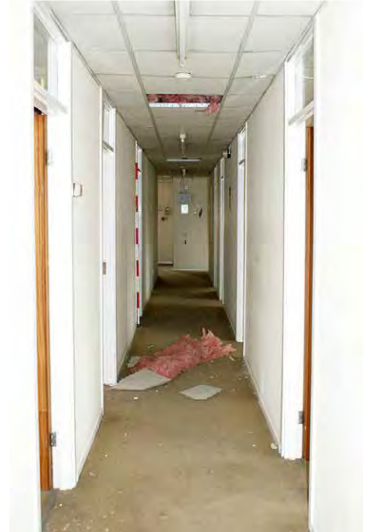
Plate 176: Corridor on sawmill building first floor
