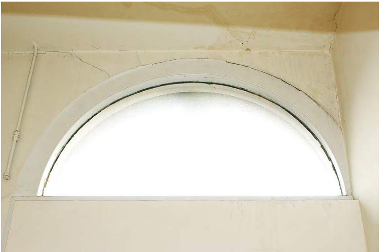
Plate 113: Plain fanlight above front door, Room G5
