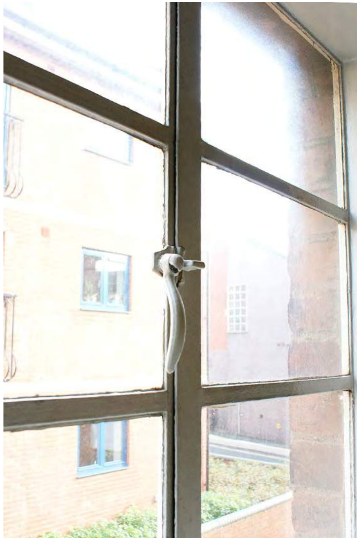
Plate 132: Curved turnbuckle window catch
