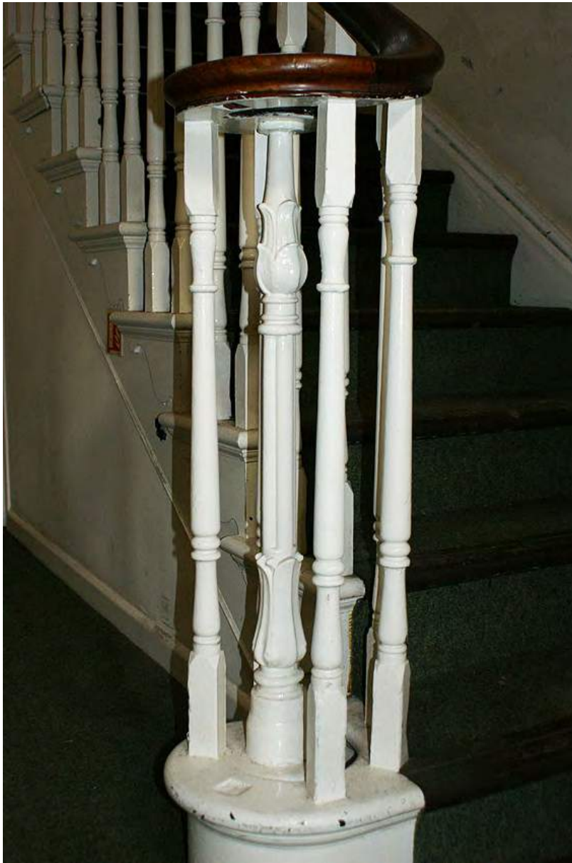
Plate 117: Curtail step with foliate carved central post and tapered column balusters
