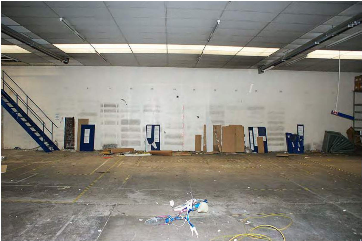
Plate28: New stud wall hiding city wall from the north
