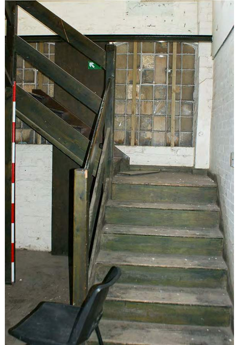
Plate 174: Staircase added into building and cut across windows
