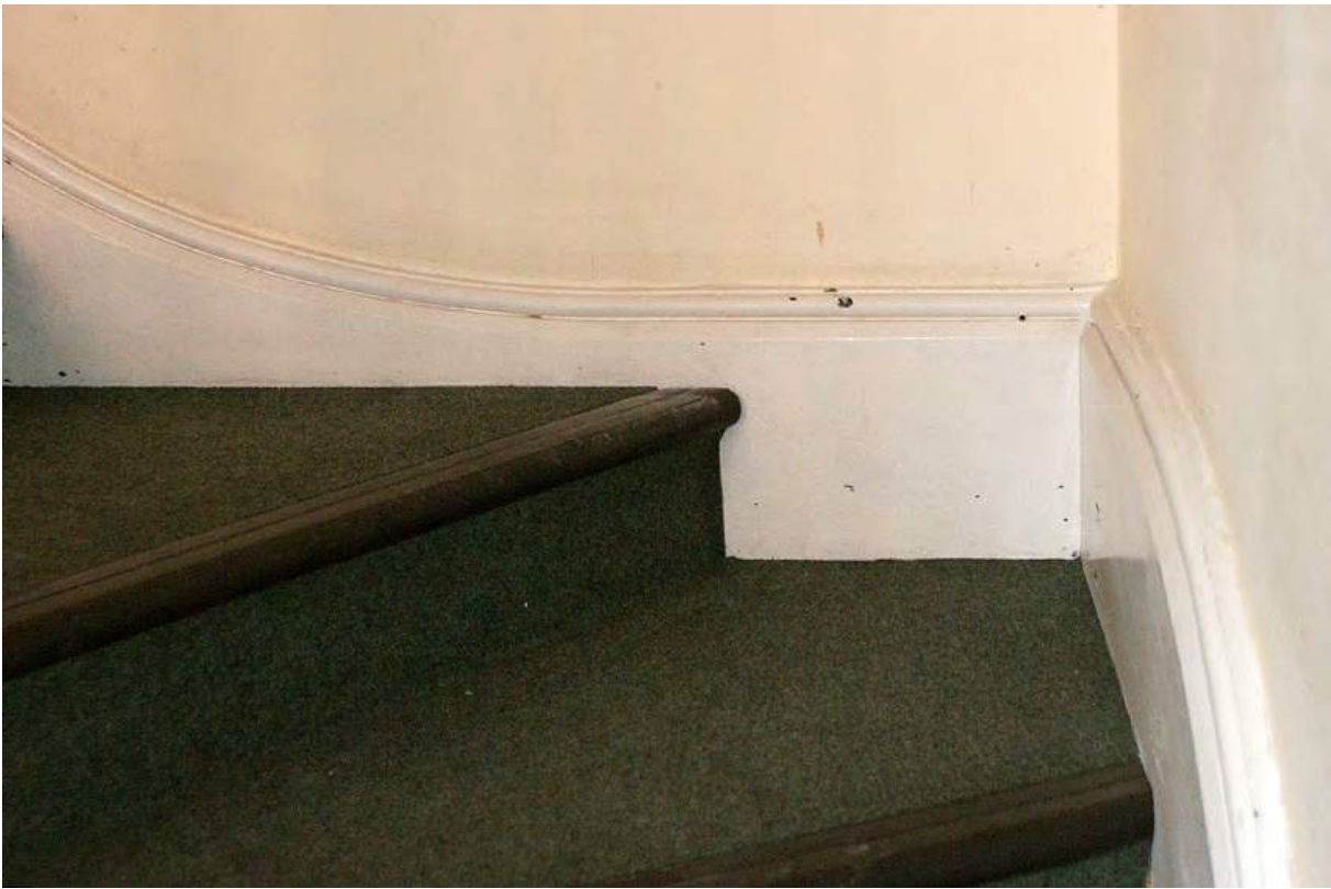
Plate 129: Roll beaded skirting on staircase, Room F3
