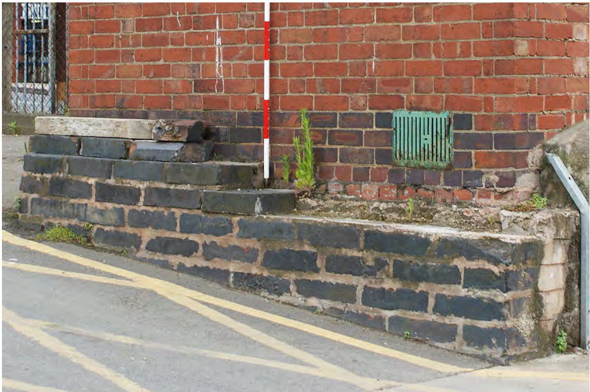
Plate 84: Air vent at base of wall of air raid shelter
