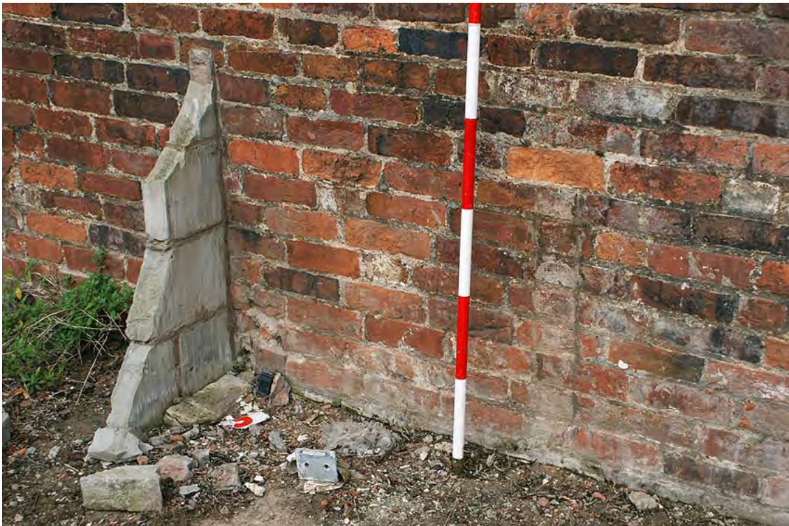
Plate 68: Breeze block stub-wall and scar from similar wall
