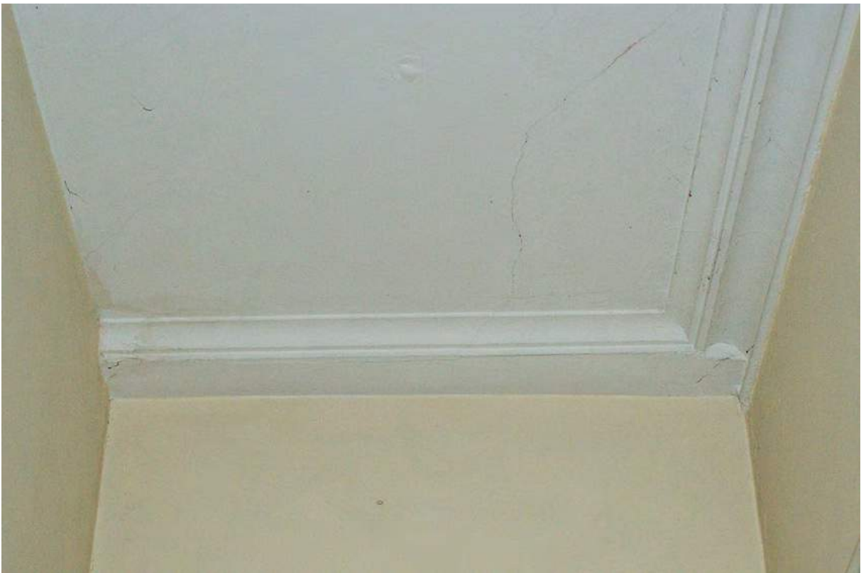
Plate 109: Moulded plaster corncicing, Room G3
