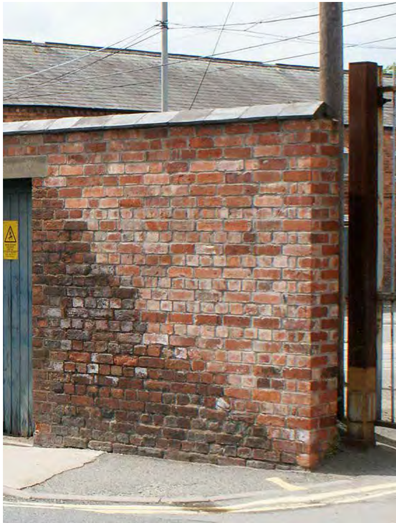
Plate 44: The Butts boundary wall rebuilt east section
