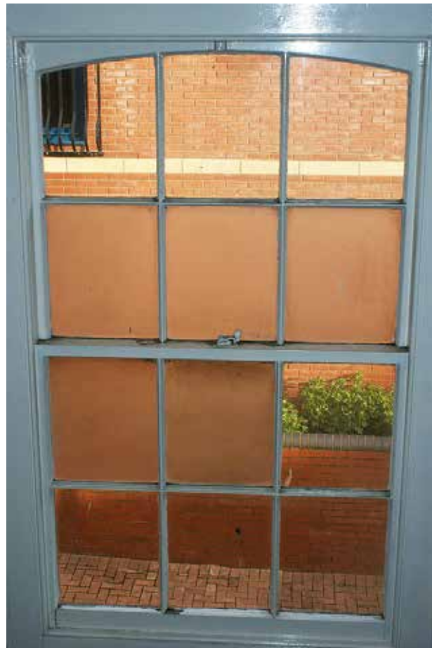
Plate 125: Staircase window, Room F3
