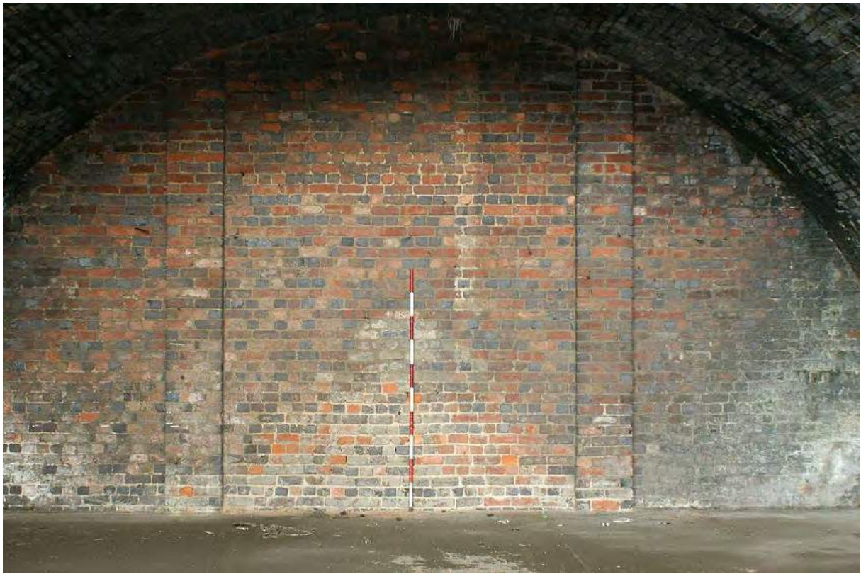
Plate 202: Blocking of The Butts siding arch
