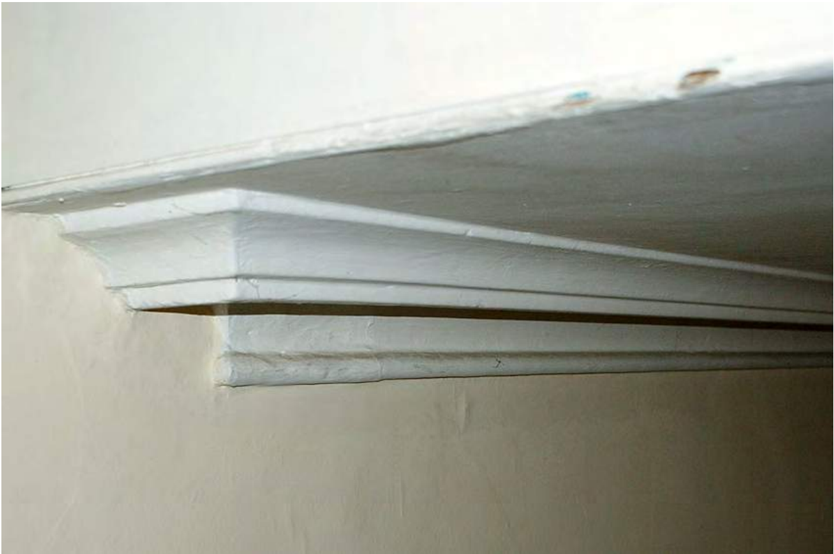
Plate 119: Example of plaster moulded cornice on staircase
