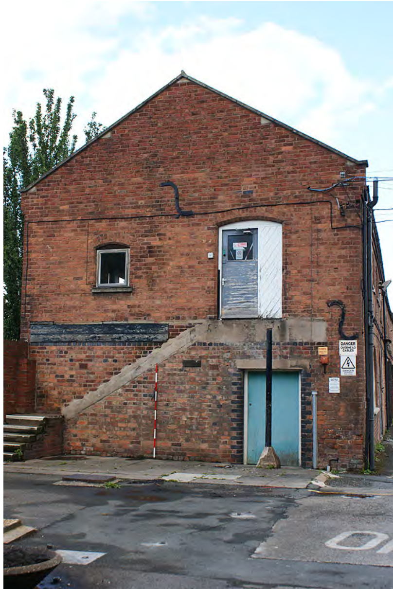
Plate 164: South elevation of sawmill building from south
