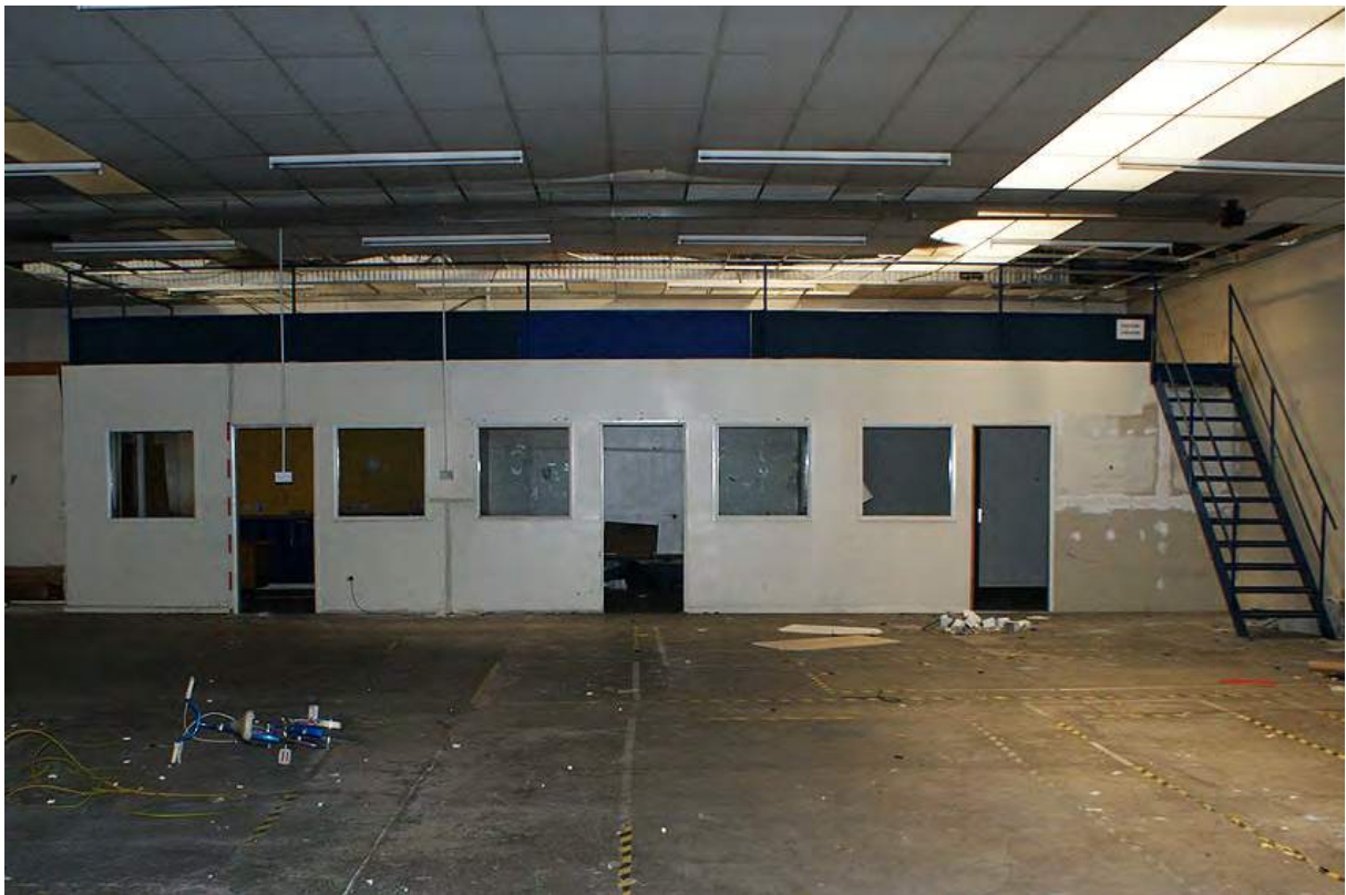
Plate 29: New offices from the west
