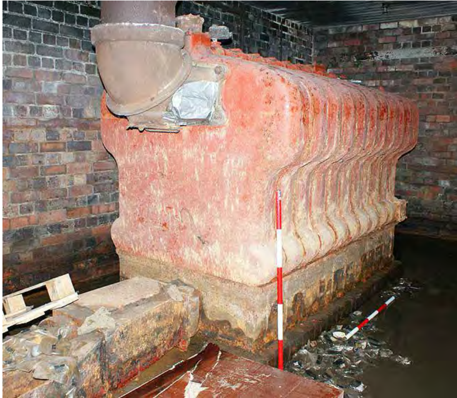
Plate 13: Cast iron boiler with Transwipers cellar, from the north
