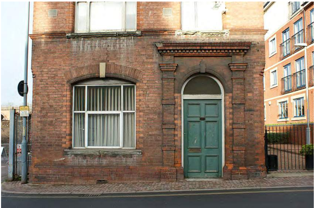
Plate 105: Ground floor, south elevation of the 'office building' fronting The Butts, showing door surround, window surround and string course
