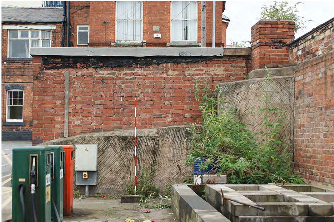
Plate 81: West elevation of air raid shelter
