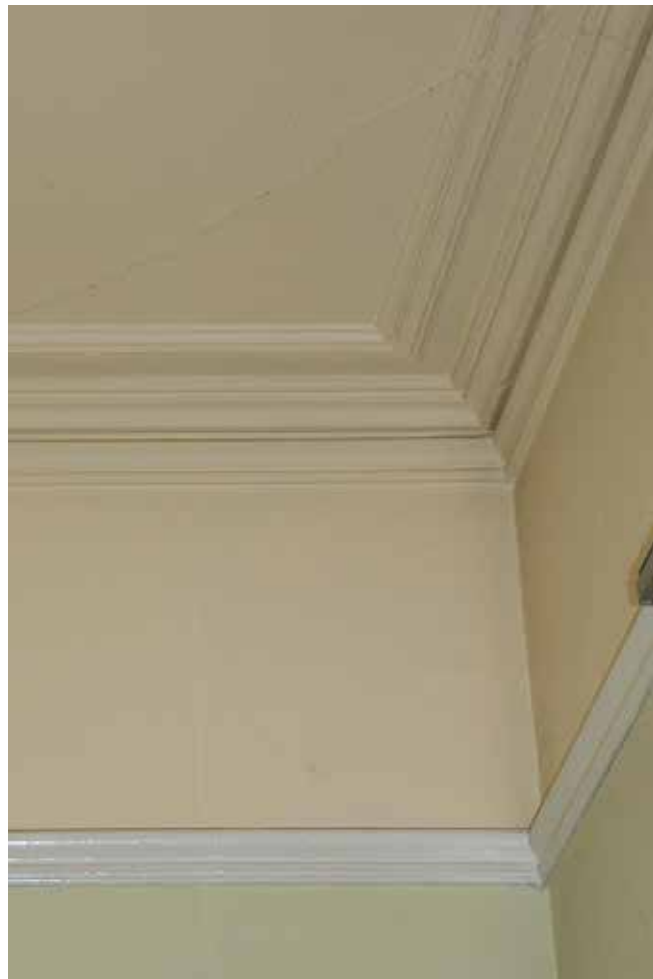
Plate 121: Cornice and picture rail, Room F1
