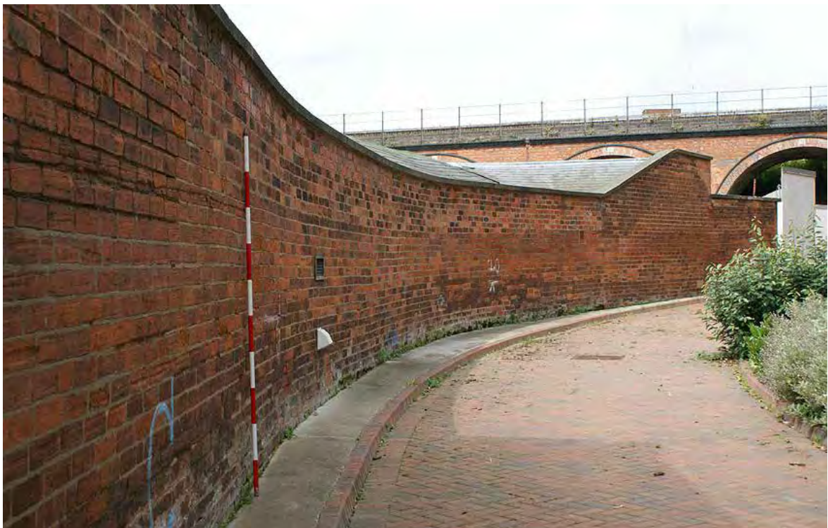
Plate 49: Netherton Lane boundary wall from the south
