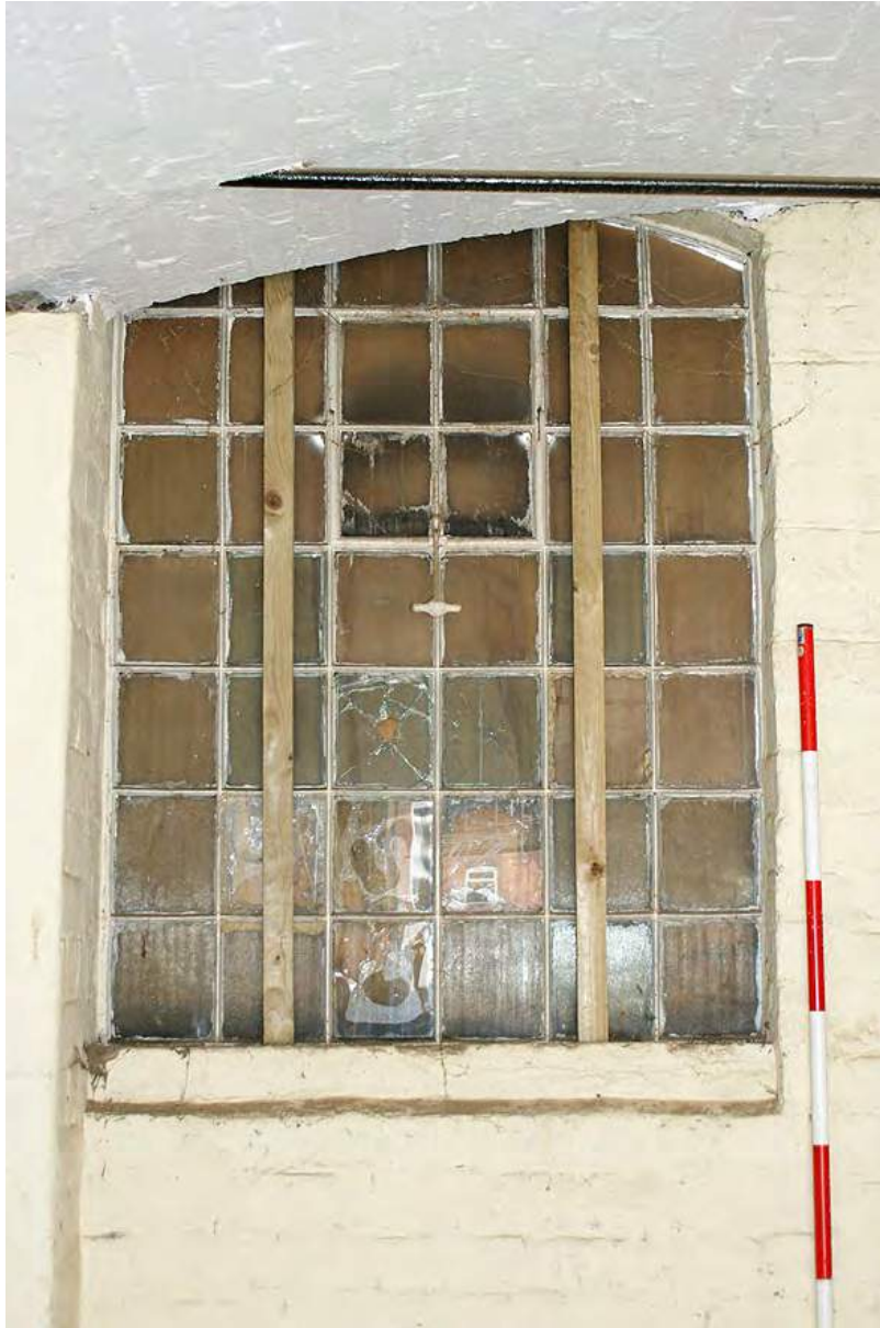
Plate 173: Windows cut across by ceiling vault
