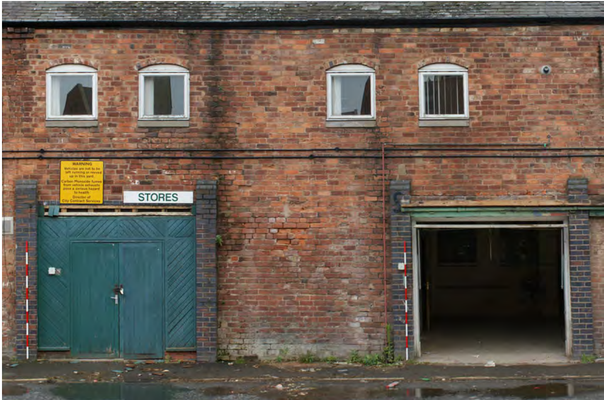
Plate 166: Buttresses formed from remains of structures built against the elevation
