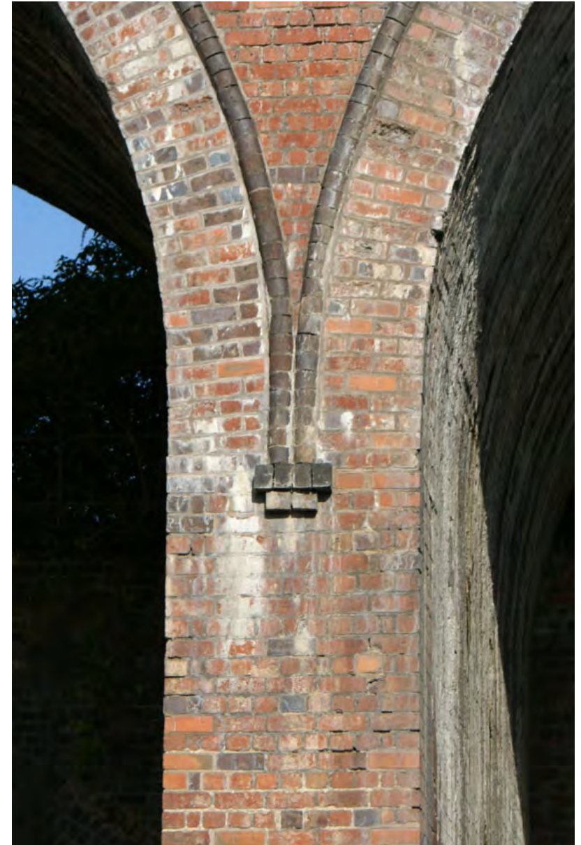
Plate 196: Viaduct arch hoodmould and stop of brick
