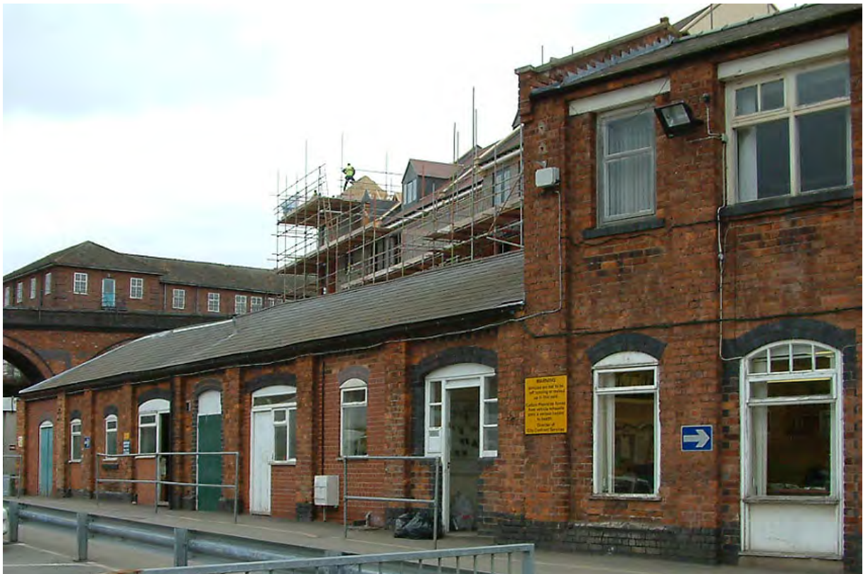
Plate 94: West elevation of single-storey range of Joseph Wood building
