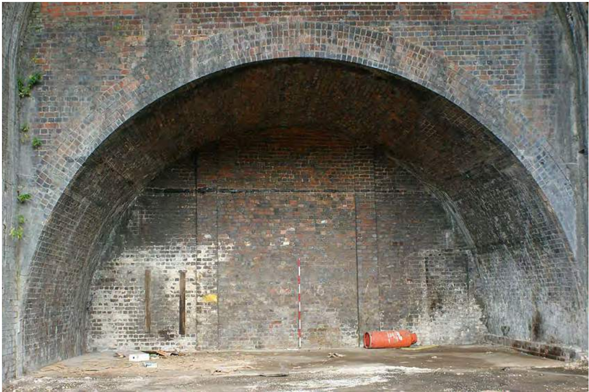
Plate 200: Vitrified bricks of The Butts siding wall
