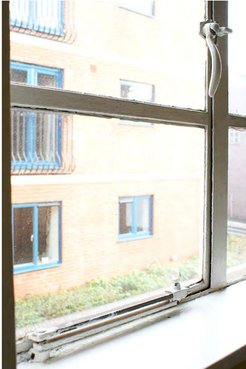
Plate 133: Slider Quadrant bar and curved turnbuckle window catch
