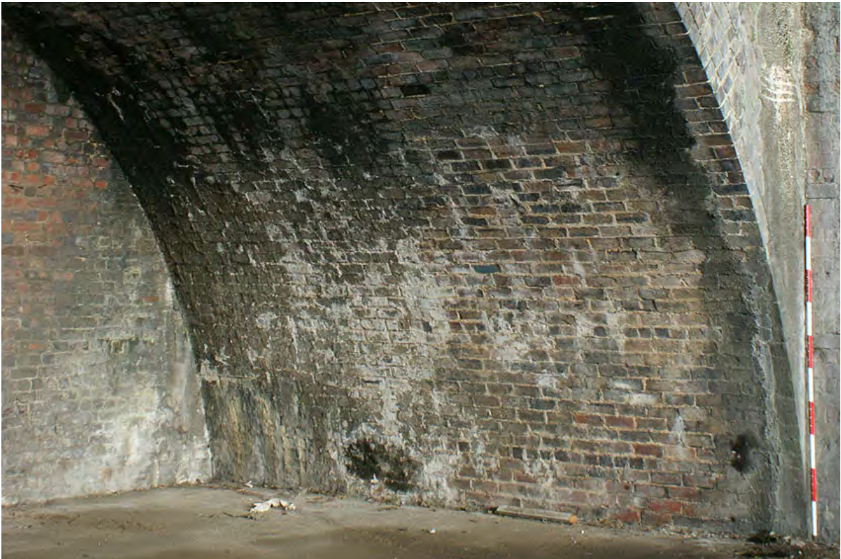
Plate 199: Brickwork of The Butts siding arch
