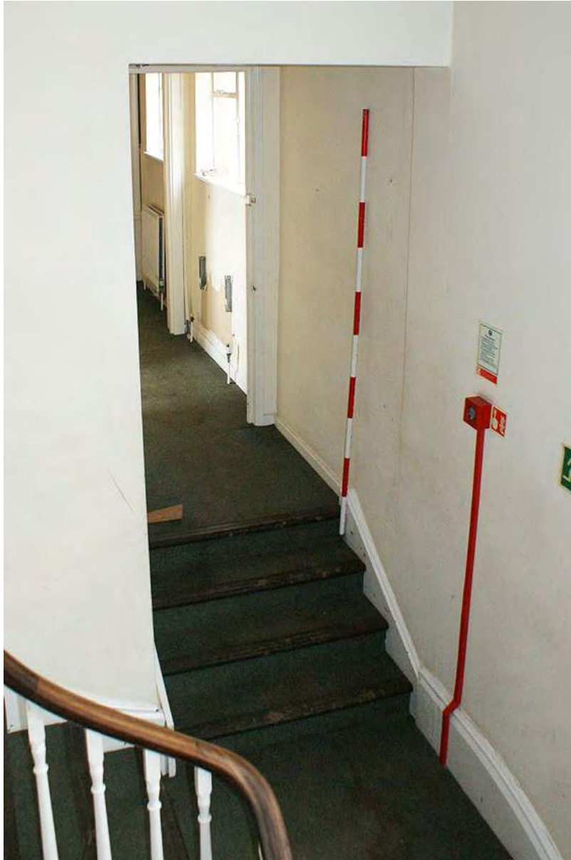
Plate 148: 1980s access to middle section first floor
