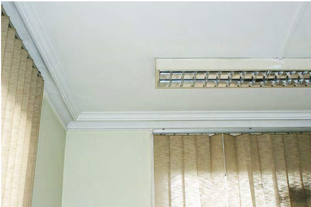
Plate 111: Moulded plaster corncing within the main building
