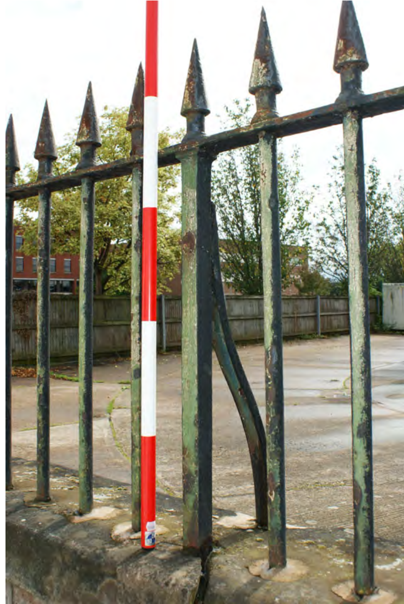
Plate 74: Square post and bracket of railings
