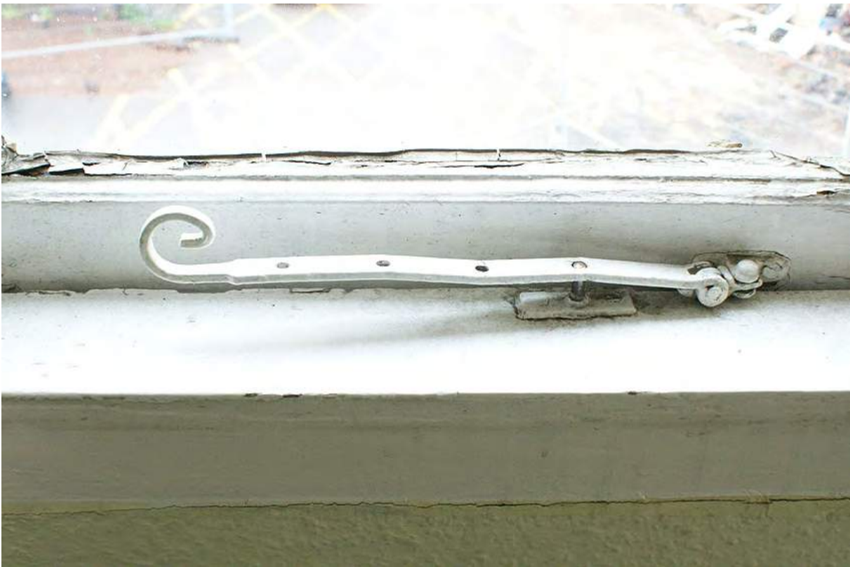
Plate 135: Spiral window stay and handle
