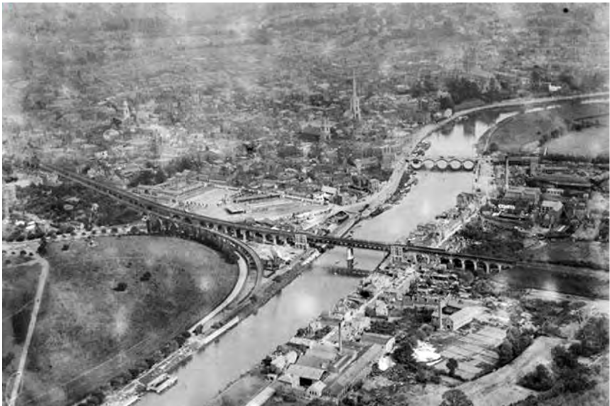
Plate 201: 1920s aerial photograph showing railway viaduct and siding (© English Heritage http://www.britainfromabove.org.uk/image/EPW005383 )
