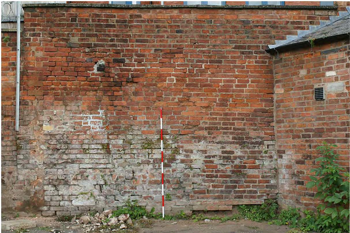
Plate 58: Wall section 3, depot side of Netherton Lane wall
