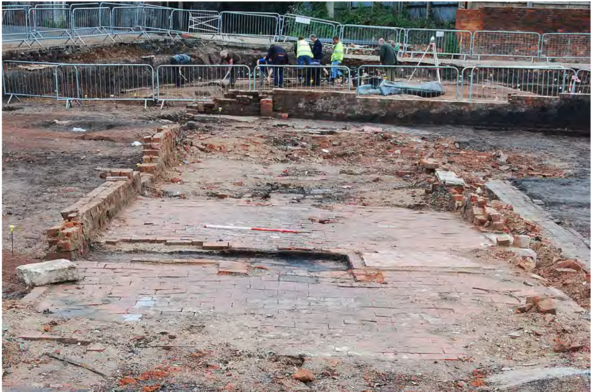
Plate 189: Almshouses foundations, from the west
