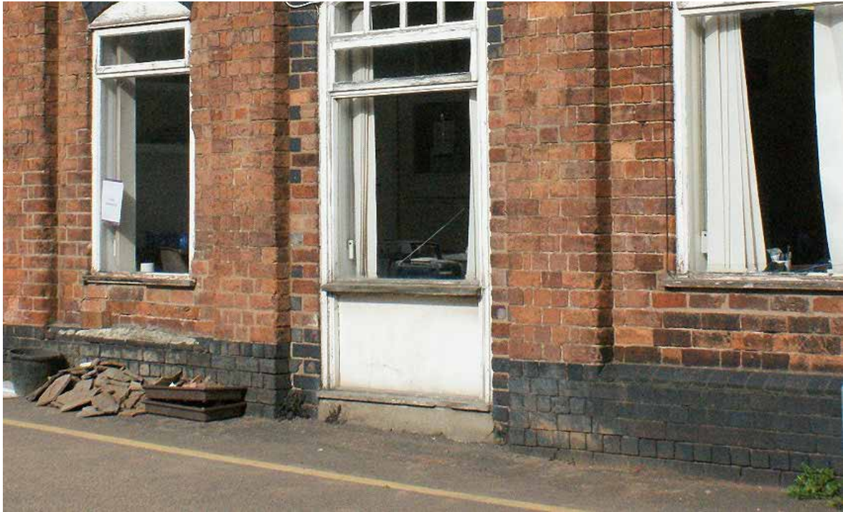
Plate 102: Plinth of two-storey range
