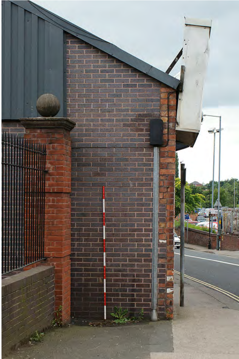
Plate 22 East elevation of Transwipers
