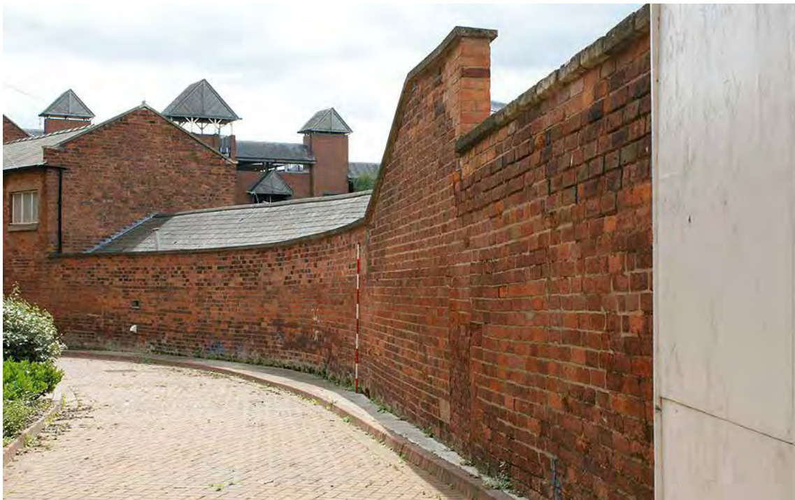
Plate 51: Netherton Lane boundary wall from the north
