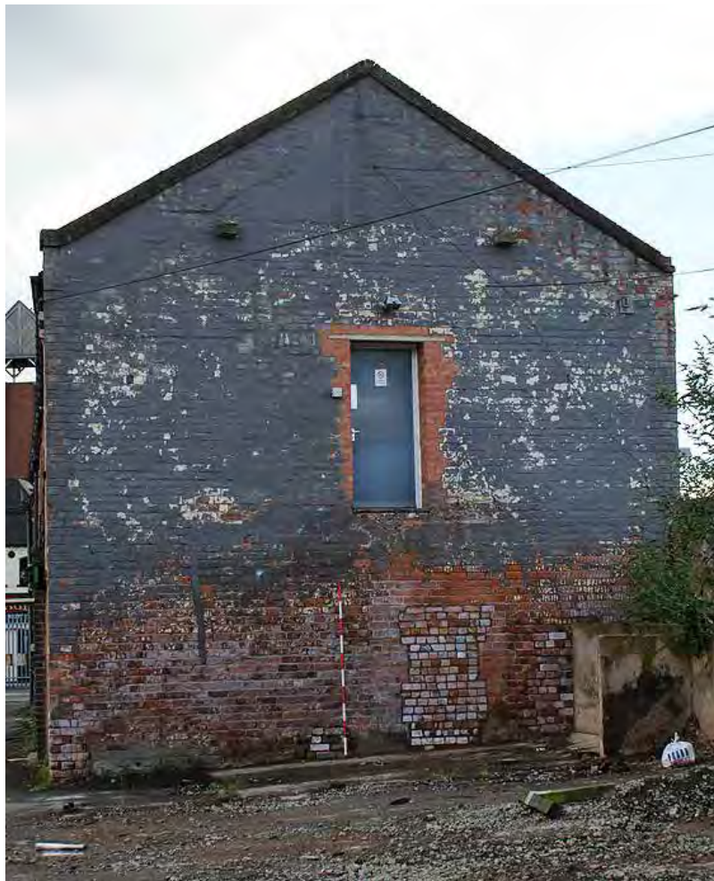
Plate 163: North elevation of sawmill building from north
