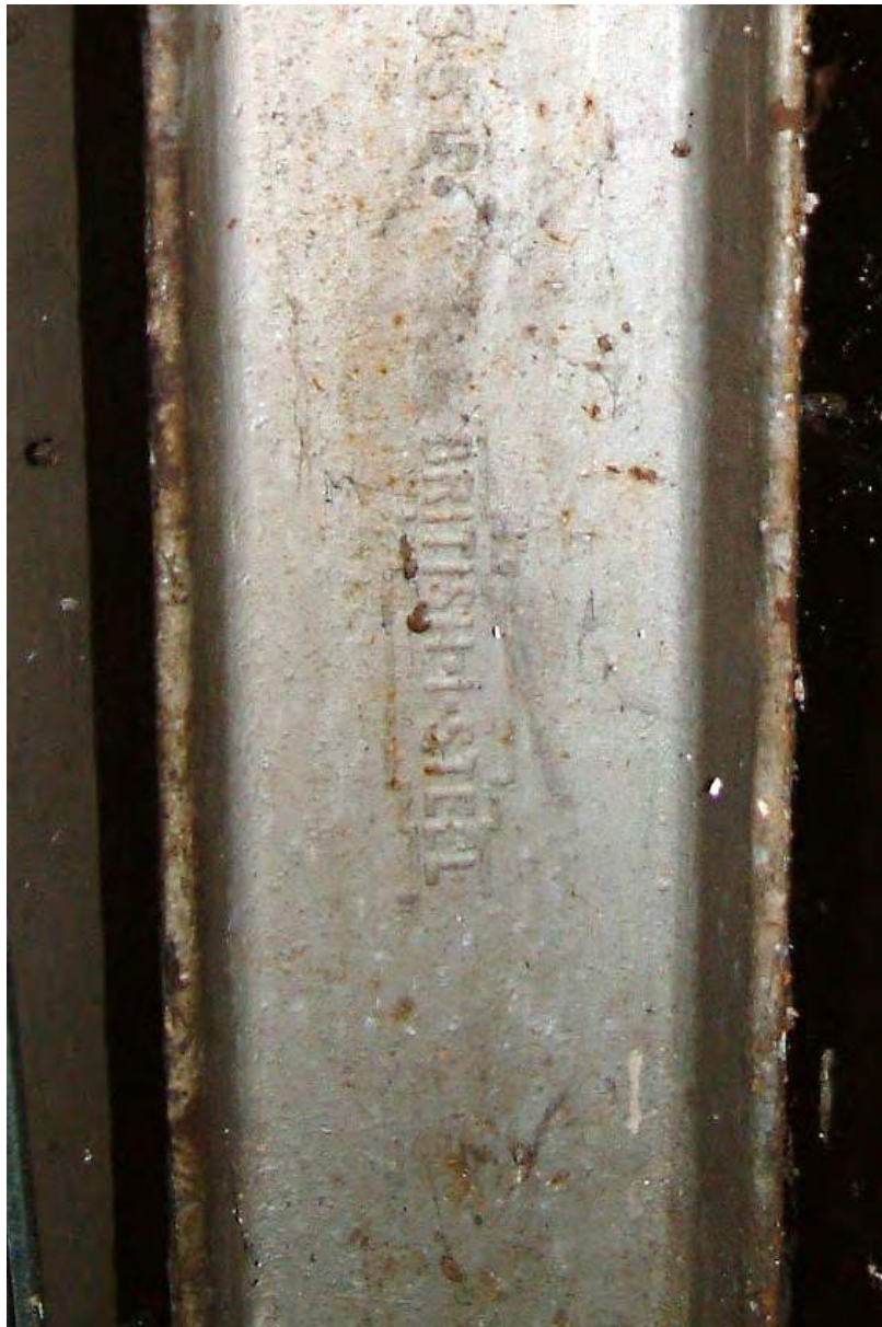
Plate 25: British Steel stanchion
