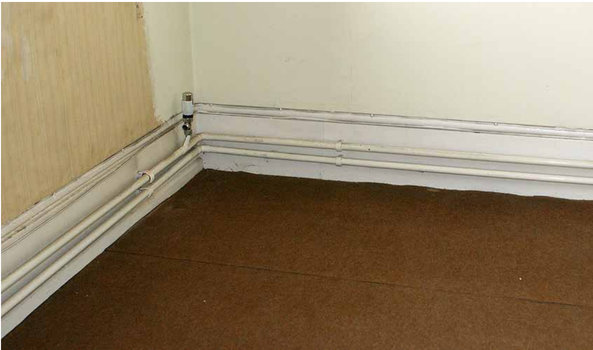
Plate 123: Example of roll beaded skirting, Room F1
