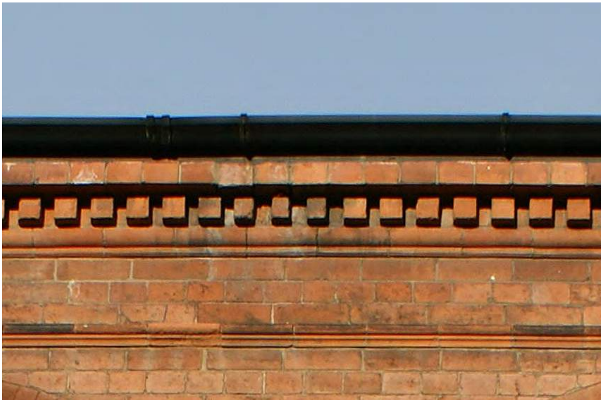
Plate 99: Moulded terracotta and brick eaves cornice
