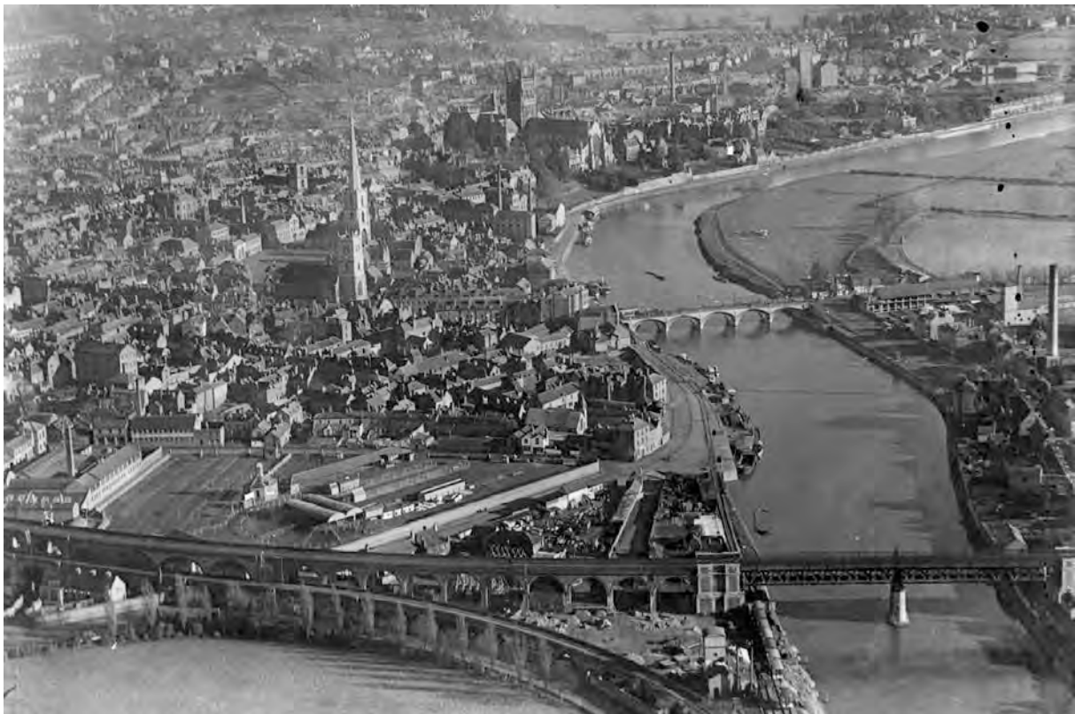
Plate 167: 1920s aerial photograph with Joseph Wood site on left middle, note tall chimney (© English Heritage http://www.britainfromabove.org.uk/image/EPW005383 )
