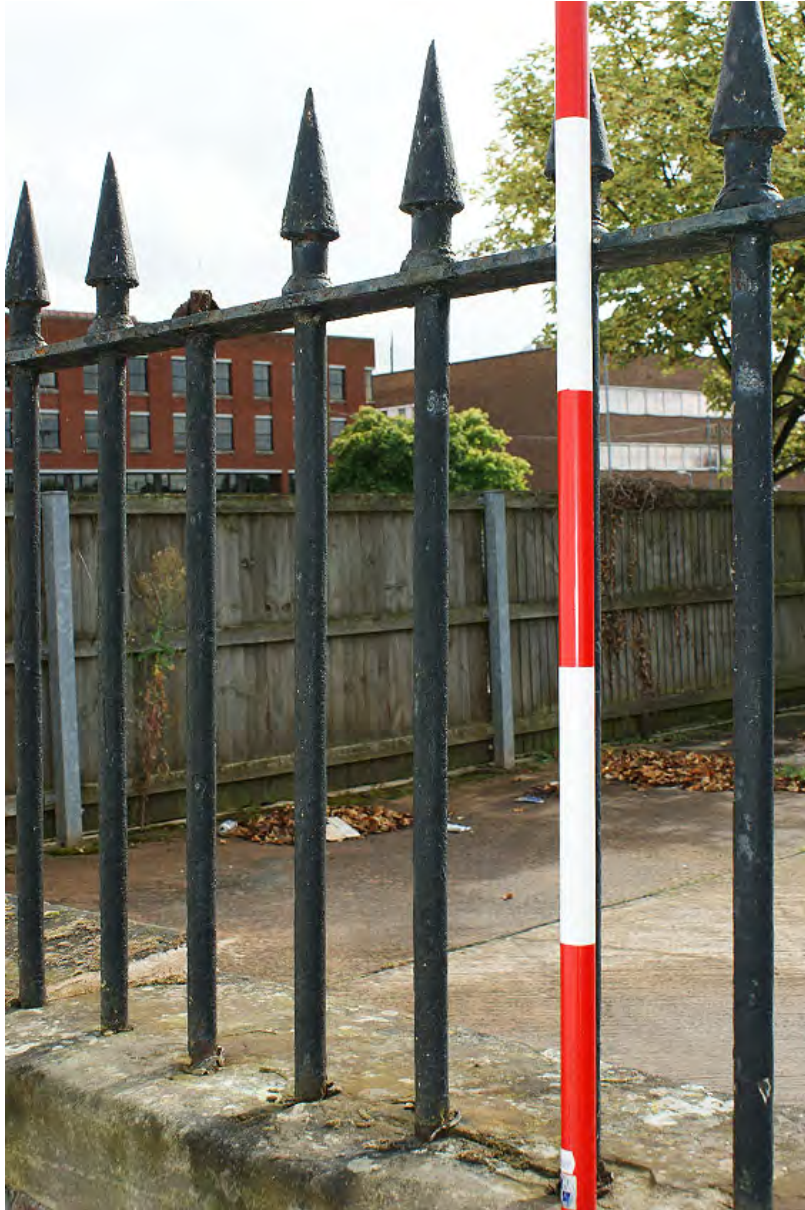
Plate 73: Tubular railing posts and spiked tops
