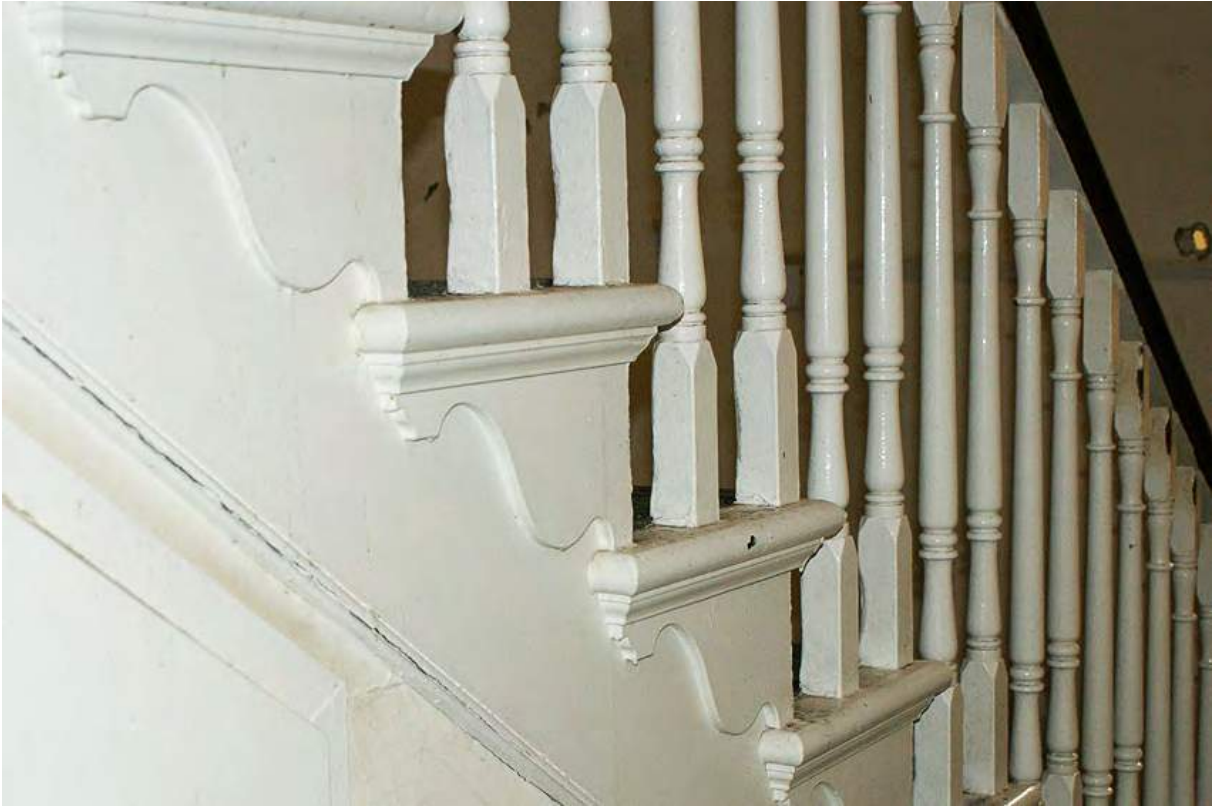
Plate 118: Open string with decorated scroll type brackets
