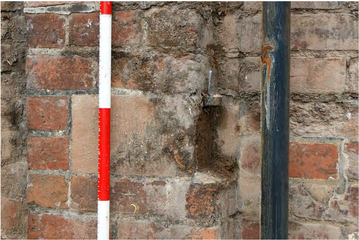
Plate 61: Hook for holding hinges of a gate
