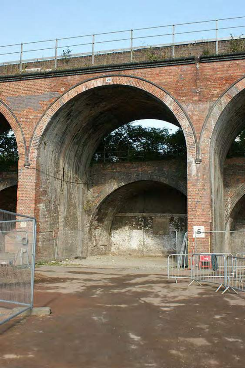
Plate 197: Viaduct arches showing arches of The Butts siding
