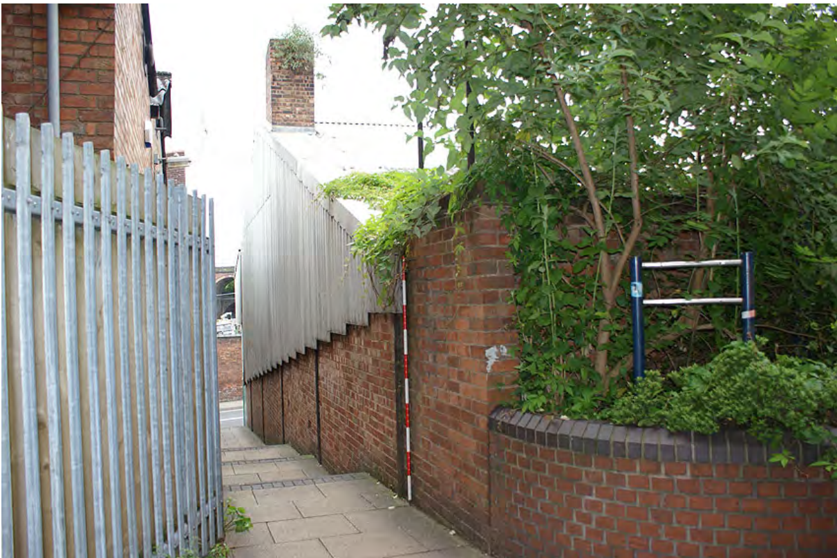
Plate 4: Transwipers building from the south-west
