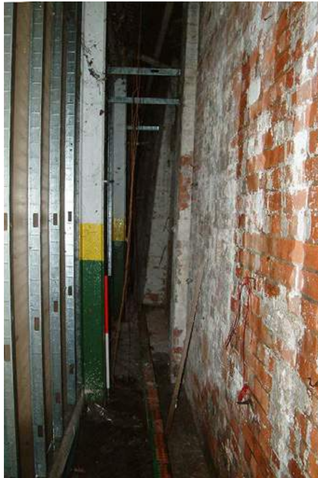
Plate 6 Transwipers interior stanchion structure from thh west
