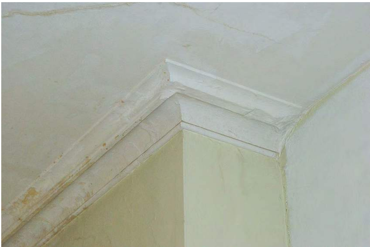
Plate 107: Moulded plaster cornicing within main building
