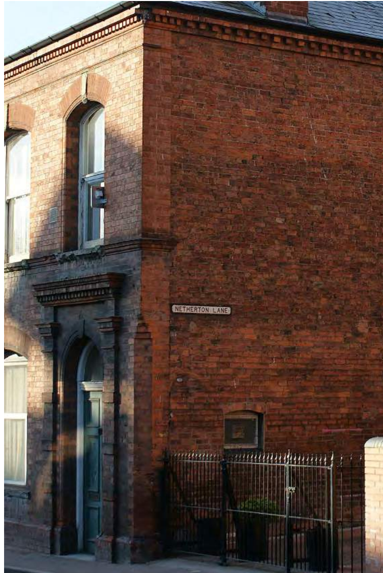
Plate 142: Clear building break between frontage and side elevations
