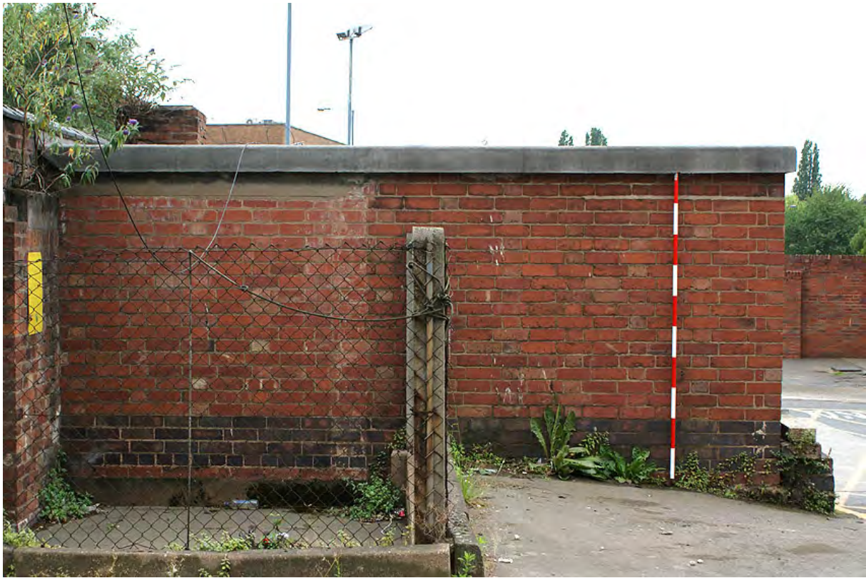
Plate 79: East elevation of air raid shelter
