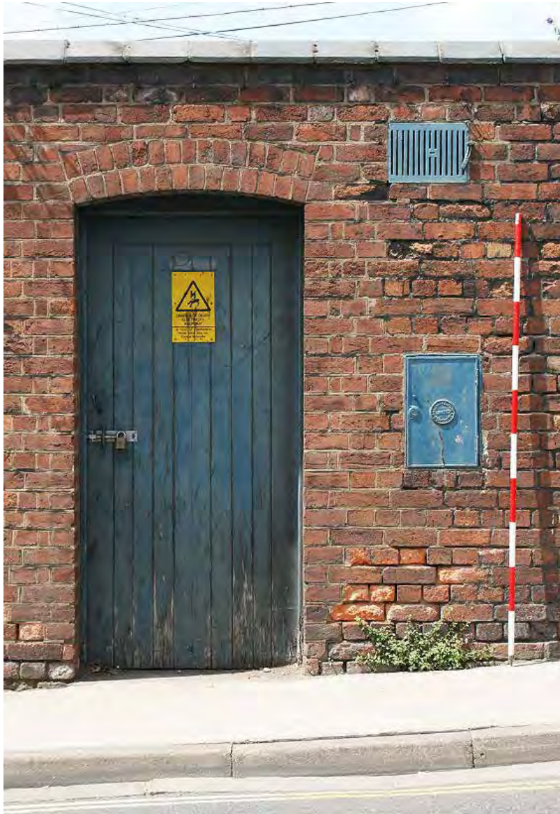
Plate 46: 1930s/40s inserted door, box and air vent
