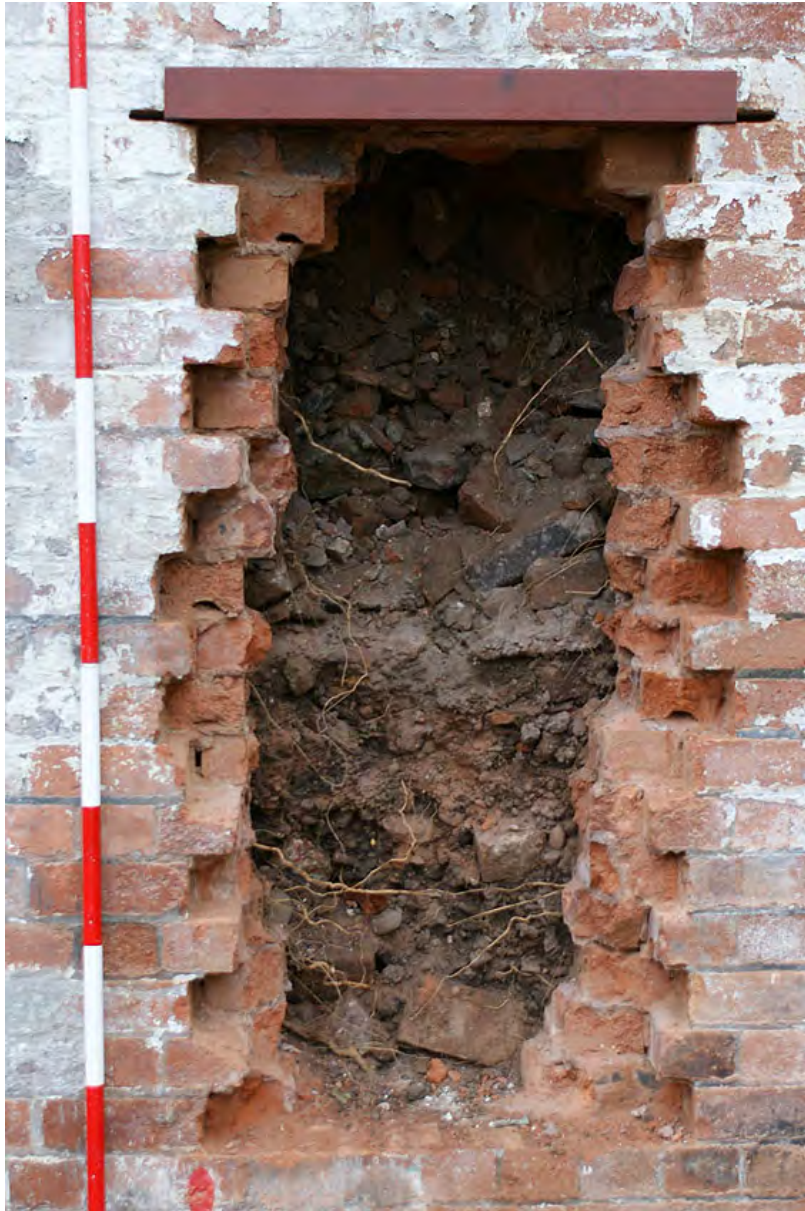
Plate 36: West side hole cut into city wall
