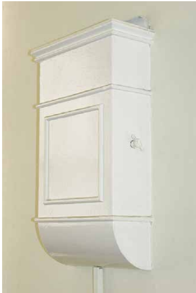
Plate 122: Unusual feature – example of ventilator with hand shaped handle
