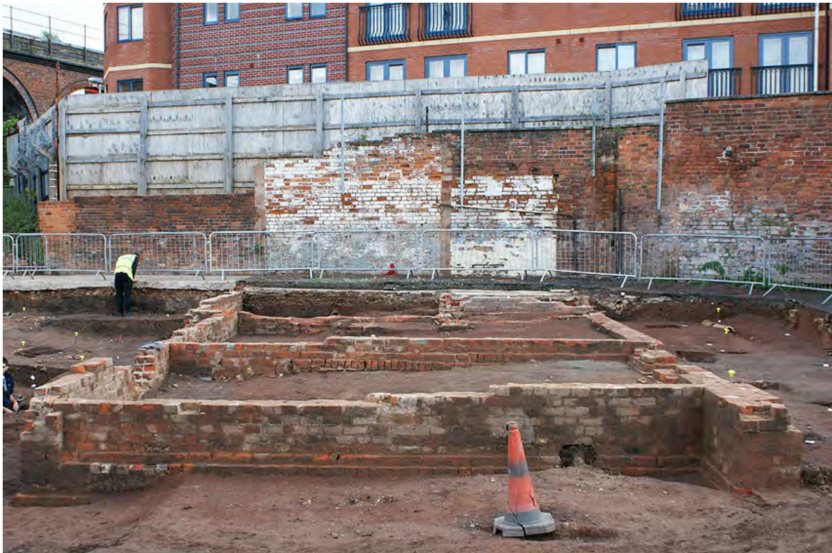
Plate 63: Foundations of range of buildings during excavation
