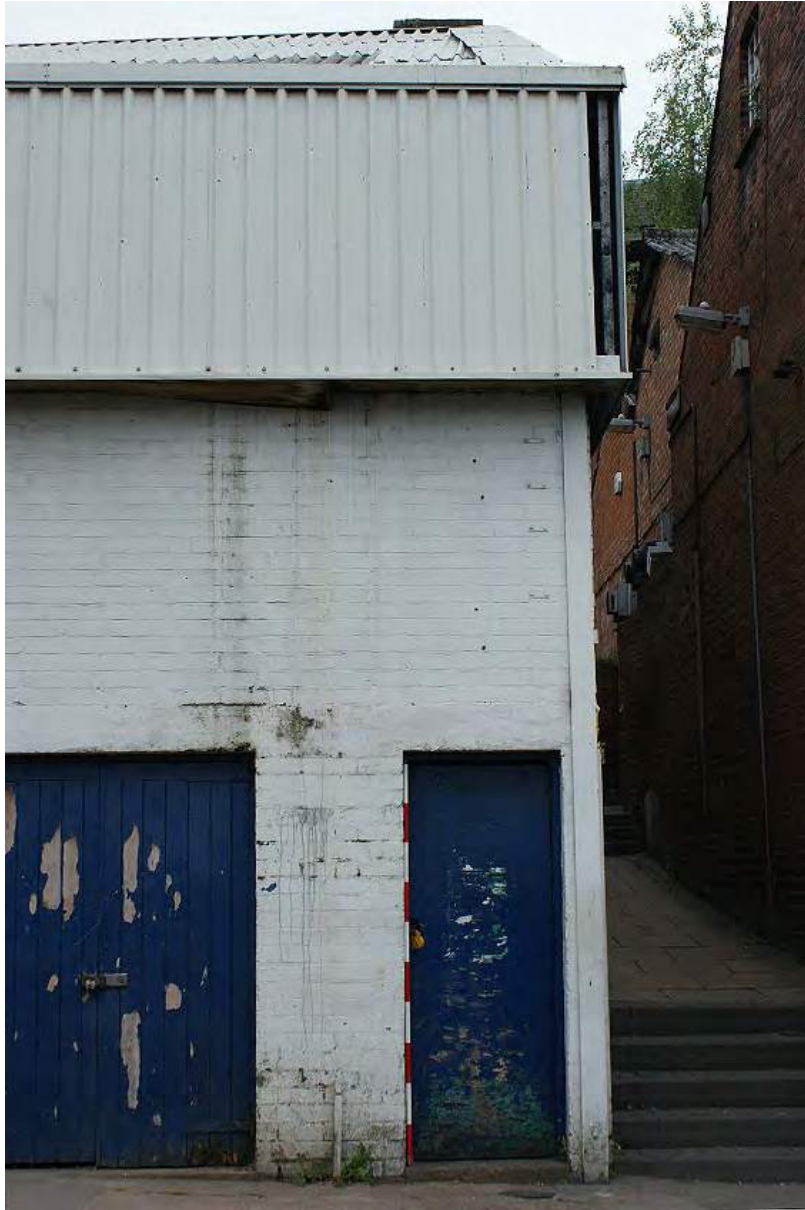
Plate 9: Entrance into cellar from The Butts
