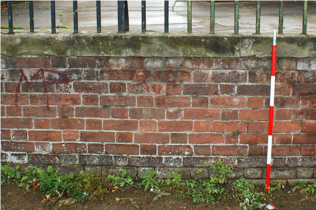
Plate 72: Coomber's boundary wall brickwork and sandstone top
