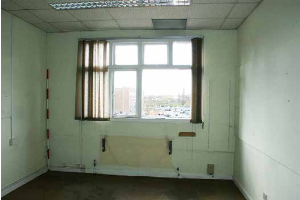
Plate 152: Office space of 1980s usage of middle section first floor
