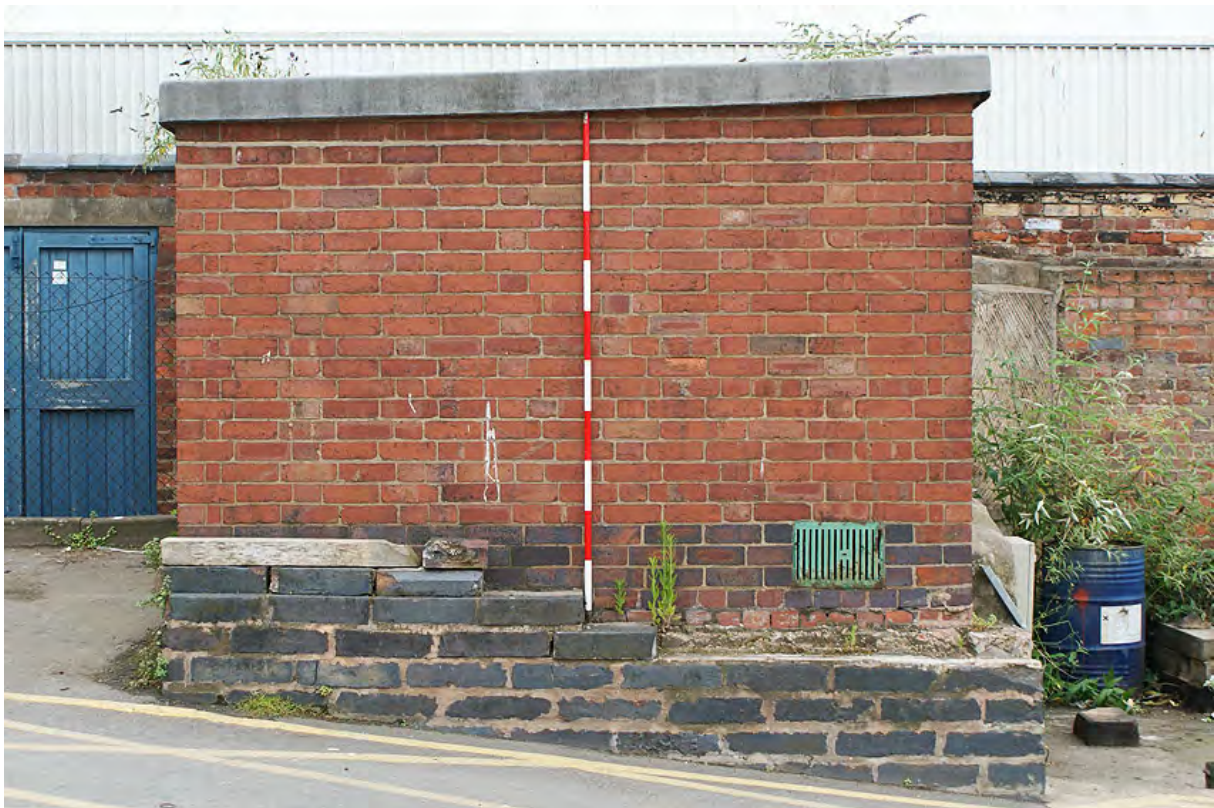
Plate 80: North elevation of air raid shelter
