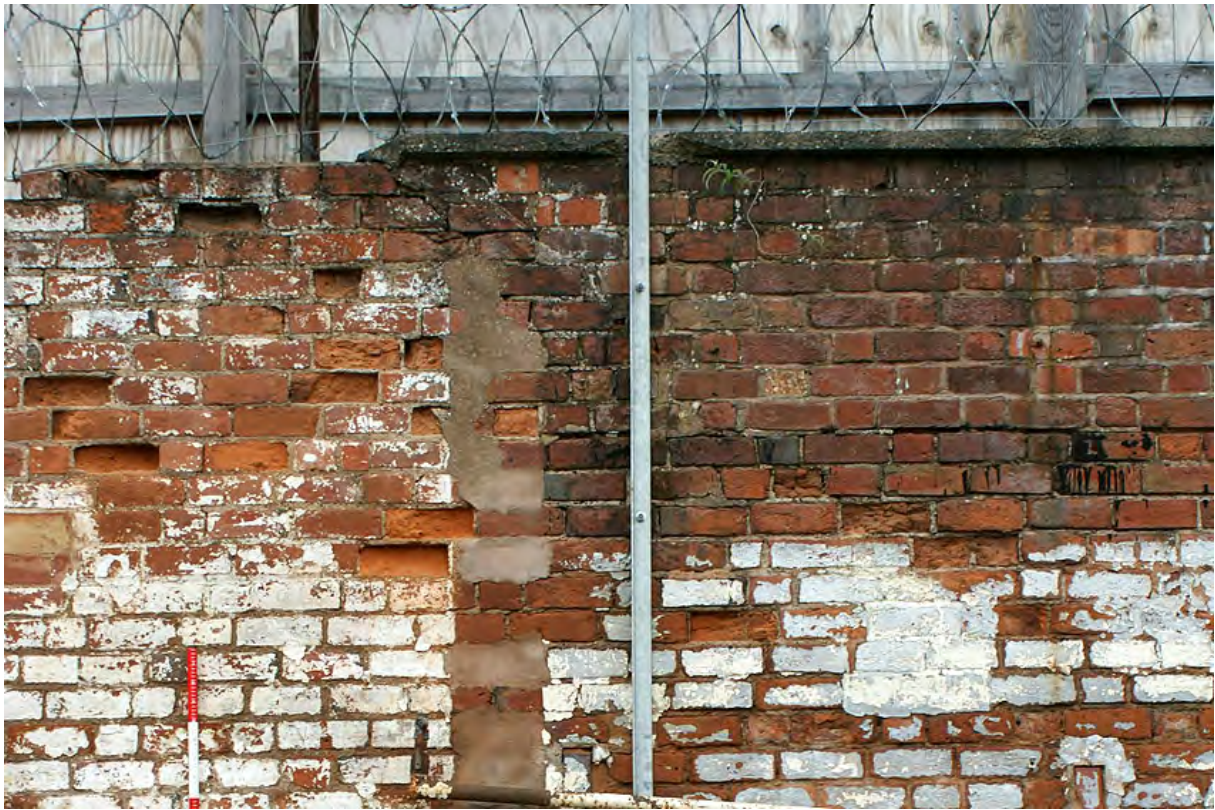
Plate 66: Roofline of former structure on wall section 5
