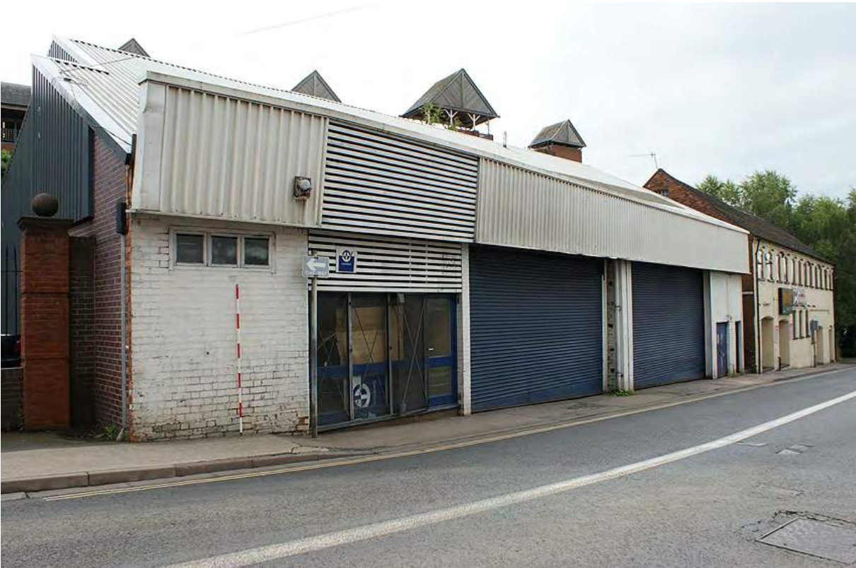
Plate 2: Transwipers building from the north-east
