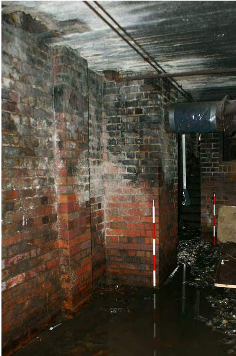
Plate 11: Base of chimney stack from the south
