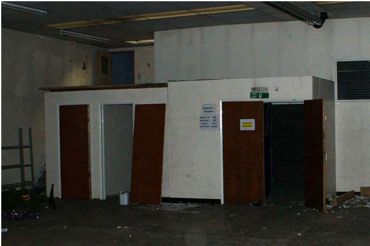
Plate 30: New breeze block utility rooms
