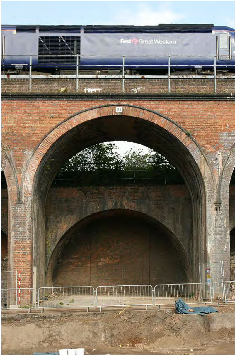
Plate 195: Viaduct arch showing stepped cornice and parapet
