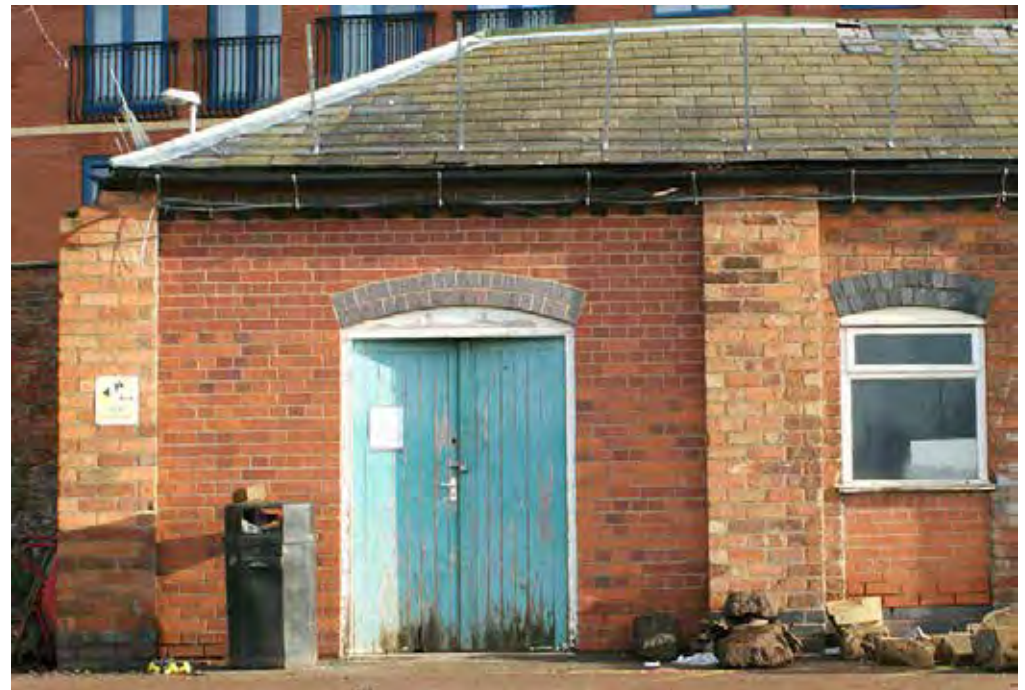
Plate 143: New wall and double-doored opening of 1970s date
