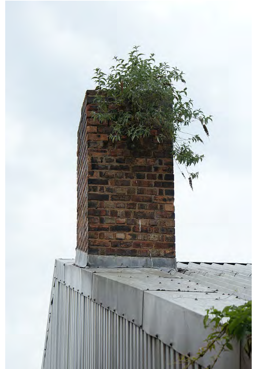
Plate 12: Chimneystack within Rack Alley elevation from the south
