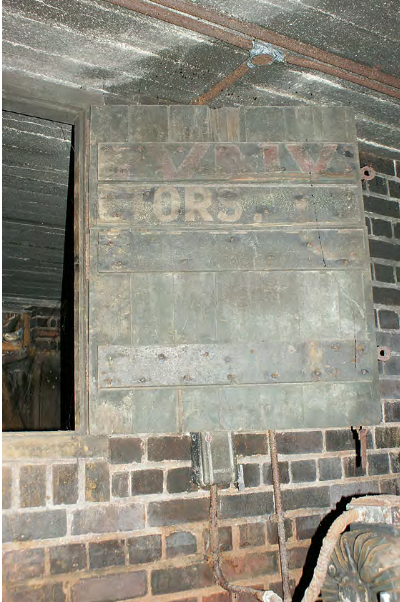
Plate 20: Coal cellar hatch from the south
