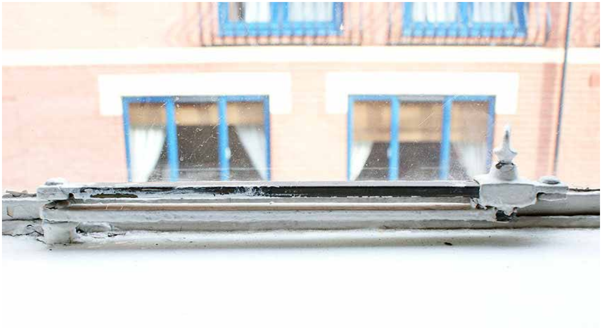
Plate 131: Slider quadrant window stay
