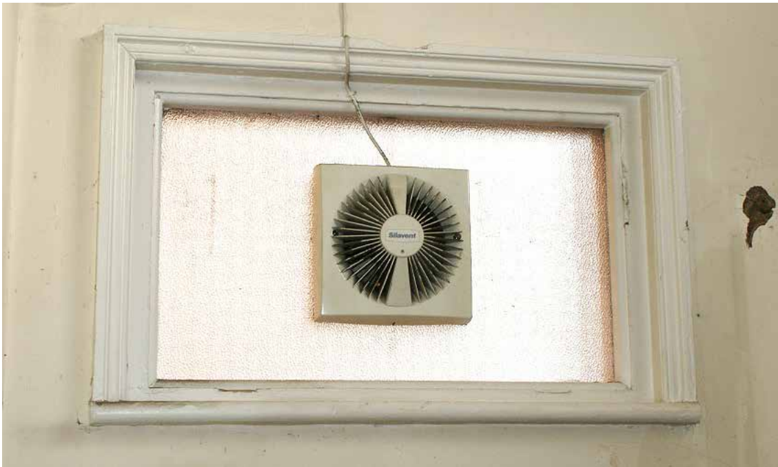
Plate 114: Example of bolection moulded window frame, Room G5
