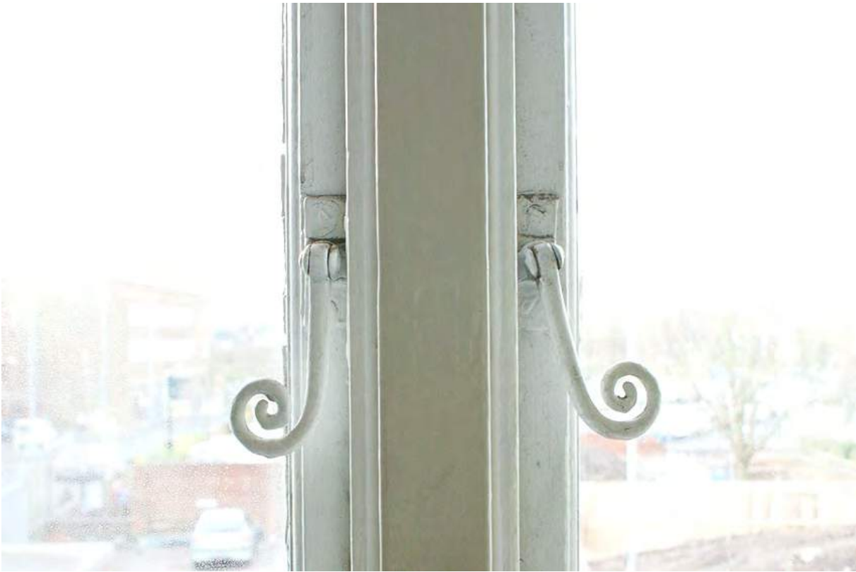
Plate 134: Spiral turnbuckle window catches
