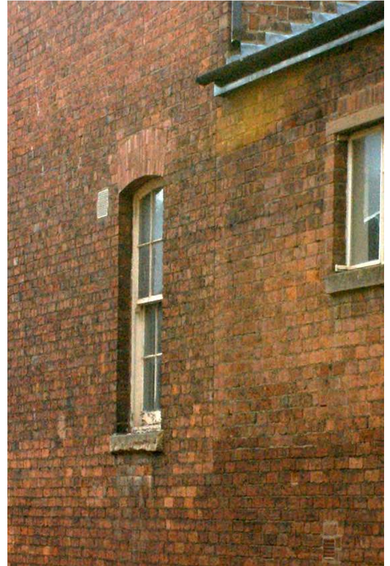
Plate 141: Building break between first floors of frontage and middle sections
