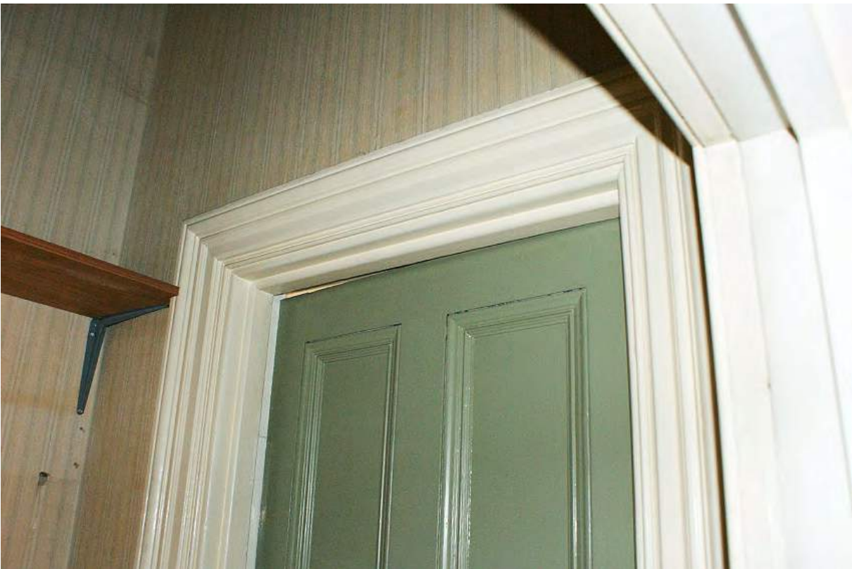
Plate 127: Surviving bolection moulded door surround, Room F4a
