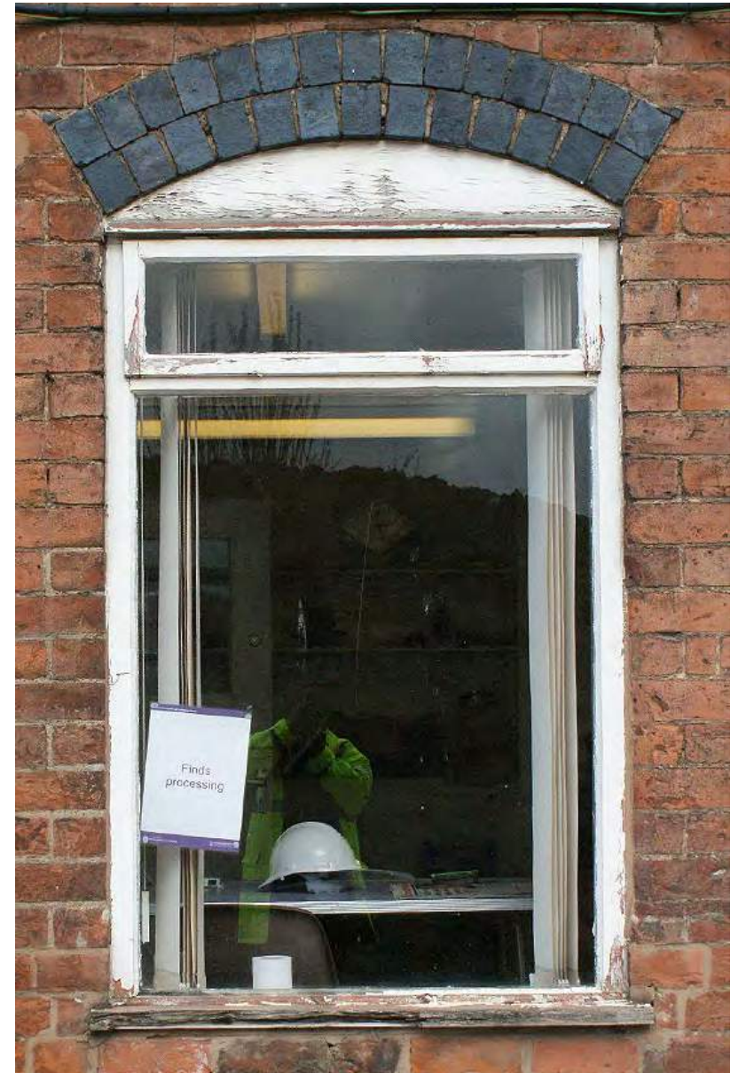
Plate 101: Blue brick window arch on two-storey range
