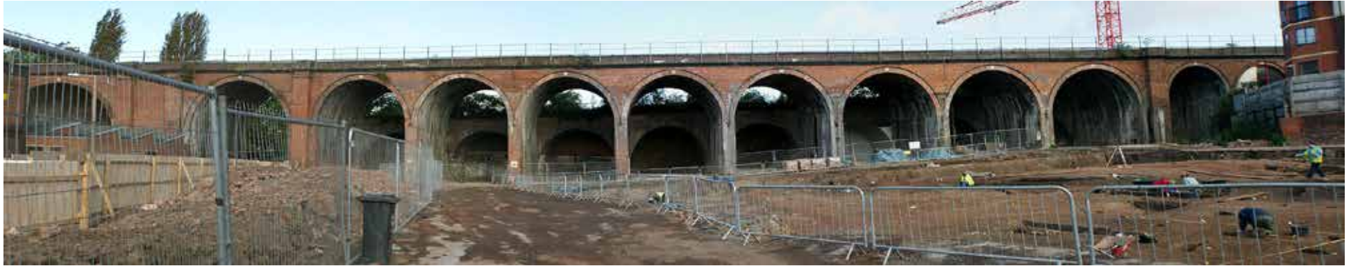
Plate 194: Viaduct arches 25 to 33 during excavation
