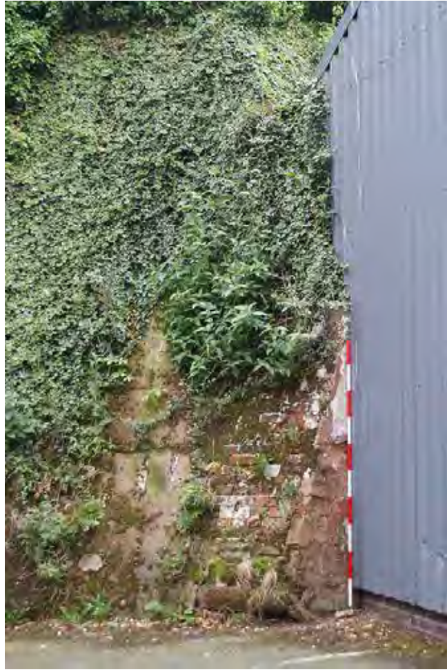
Plate 34: Tower or bastion remains on land adjacent to Transwipers
