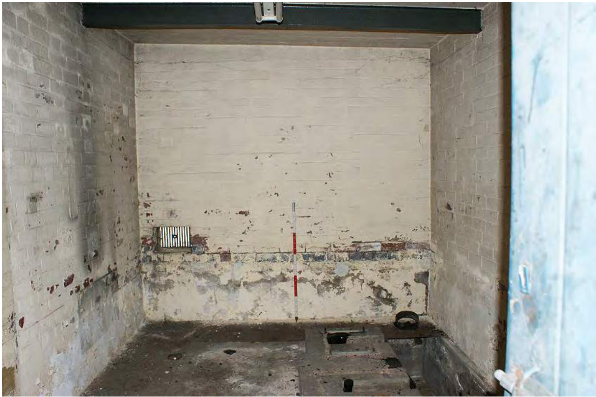
Plate 89: Interior of air raid shelter
