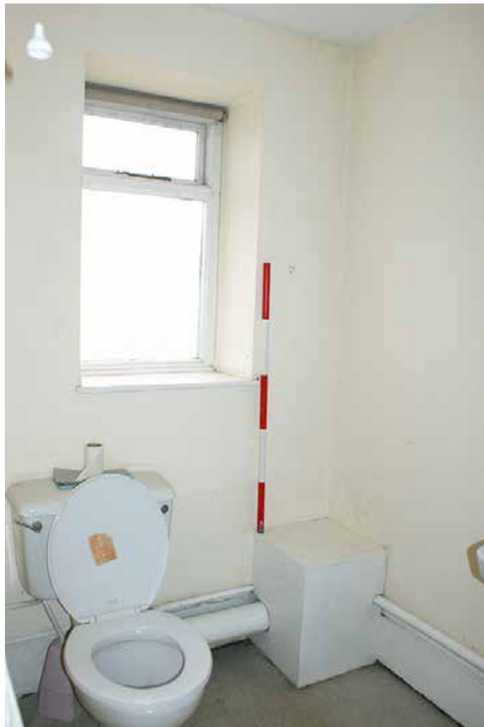
Plate 153: 1980s bathroom created on frontage section first floor
