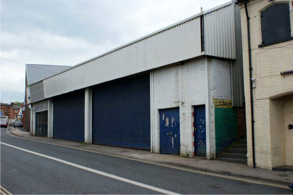
Plate 1: Transwipers building from the north-west
