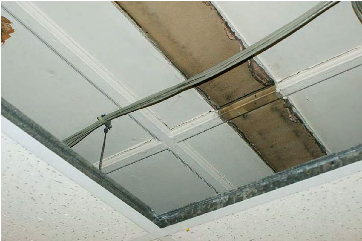
Plate 130: Ovolo moulded wood creating panelled ceiling, above later suspended ceiling, Room F10
