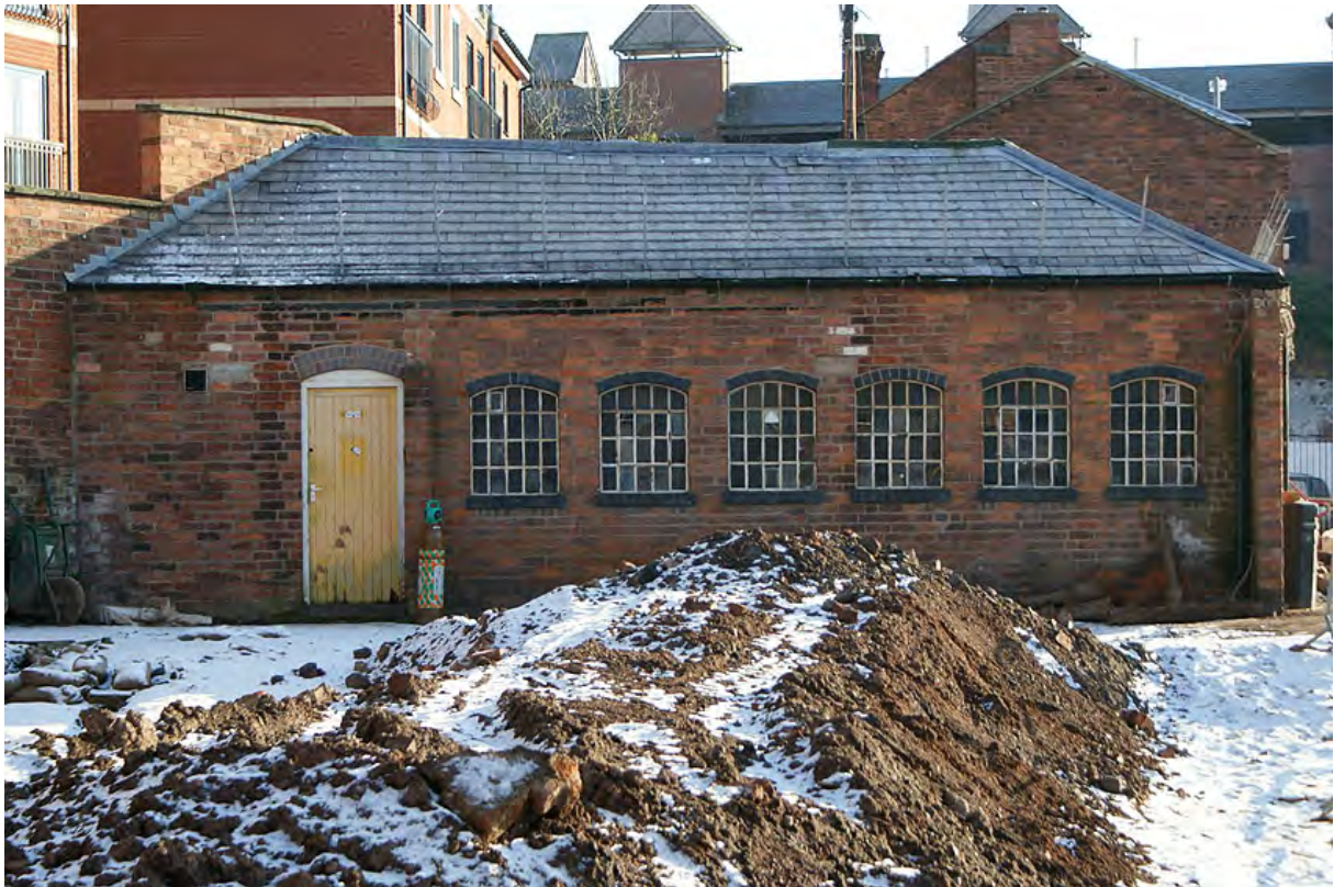
Plate 95: North elevation of single-storey range of Joseph Wood building
