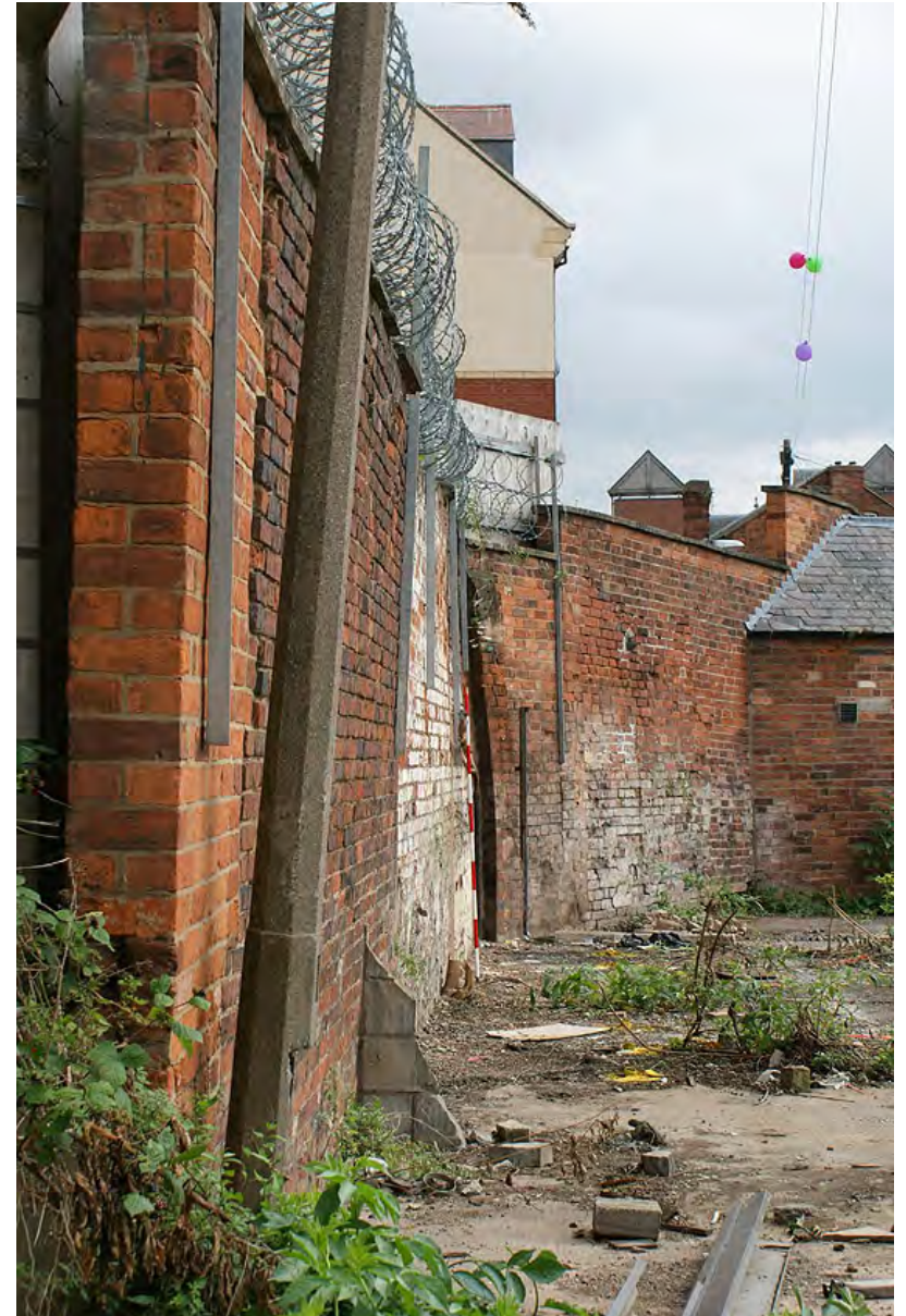
Plate 57: Depot side of Netherton Lane wall
