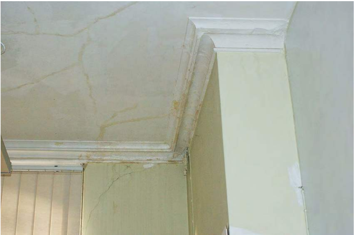
Plate 108: Moulded plaster corncicing within the main building
