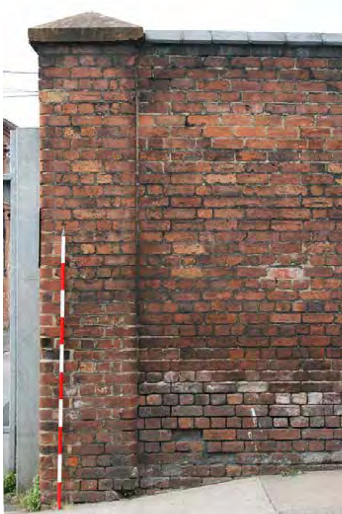
Plate 42: West end pier of The Butts boundary wall
