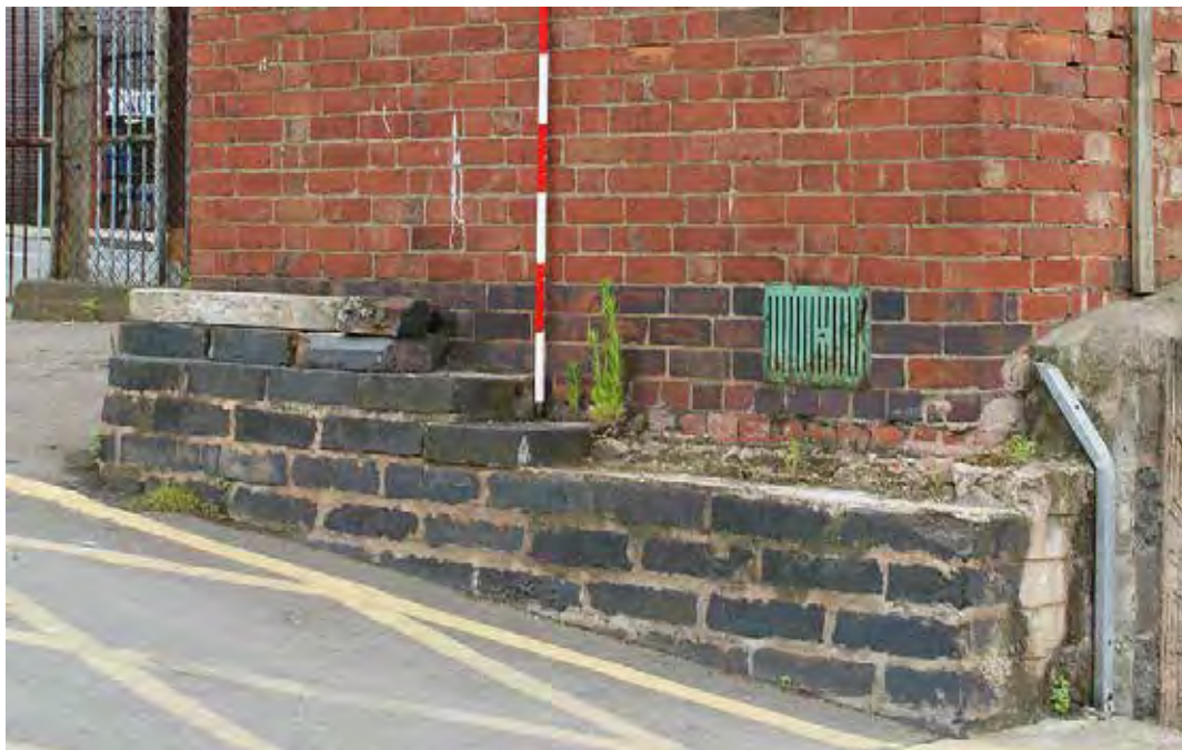
Plate 88: Low level wall constructed of engineering brick
