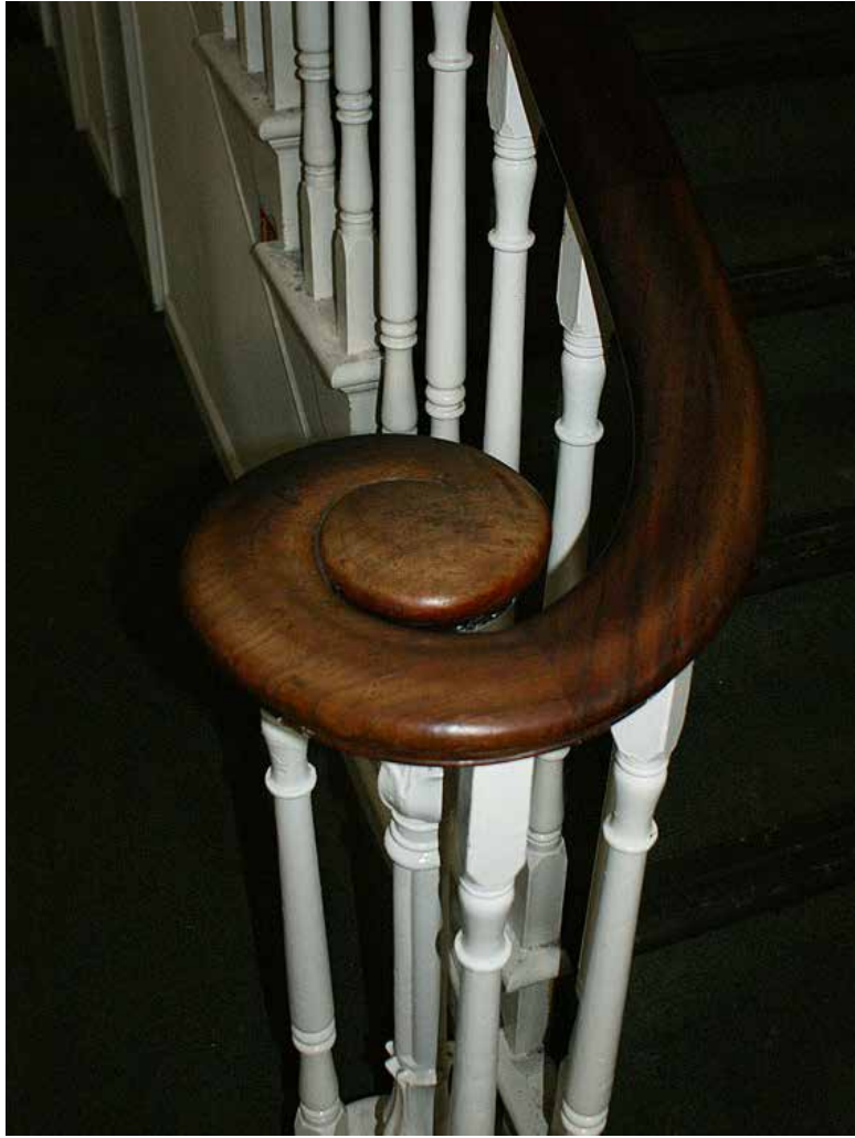
Plate 136: Gently curved flat top stair handrail
