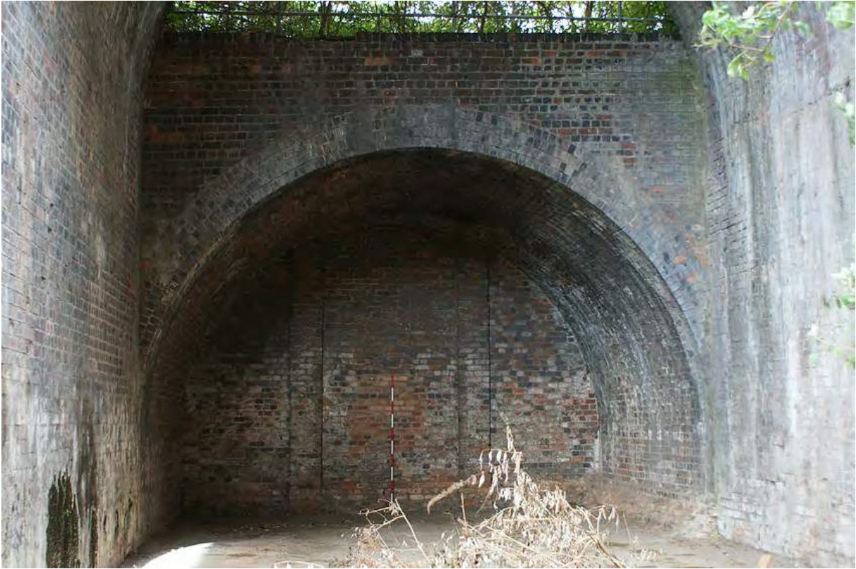
Plate 198: Arch of The Butts siding
