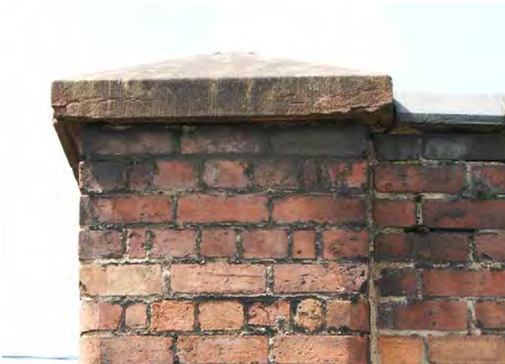
Plate 43: Sandstone capital to pier
