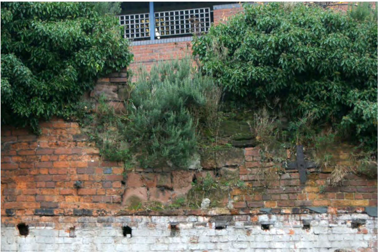
Plate 33: Stonework at top of the city wall
