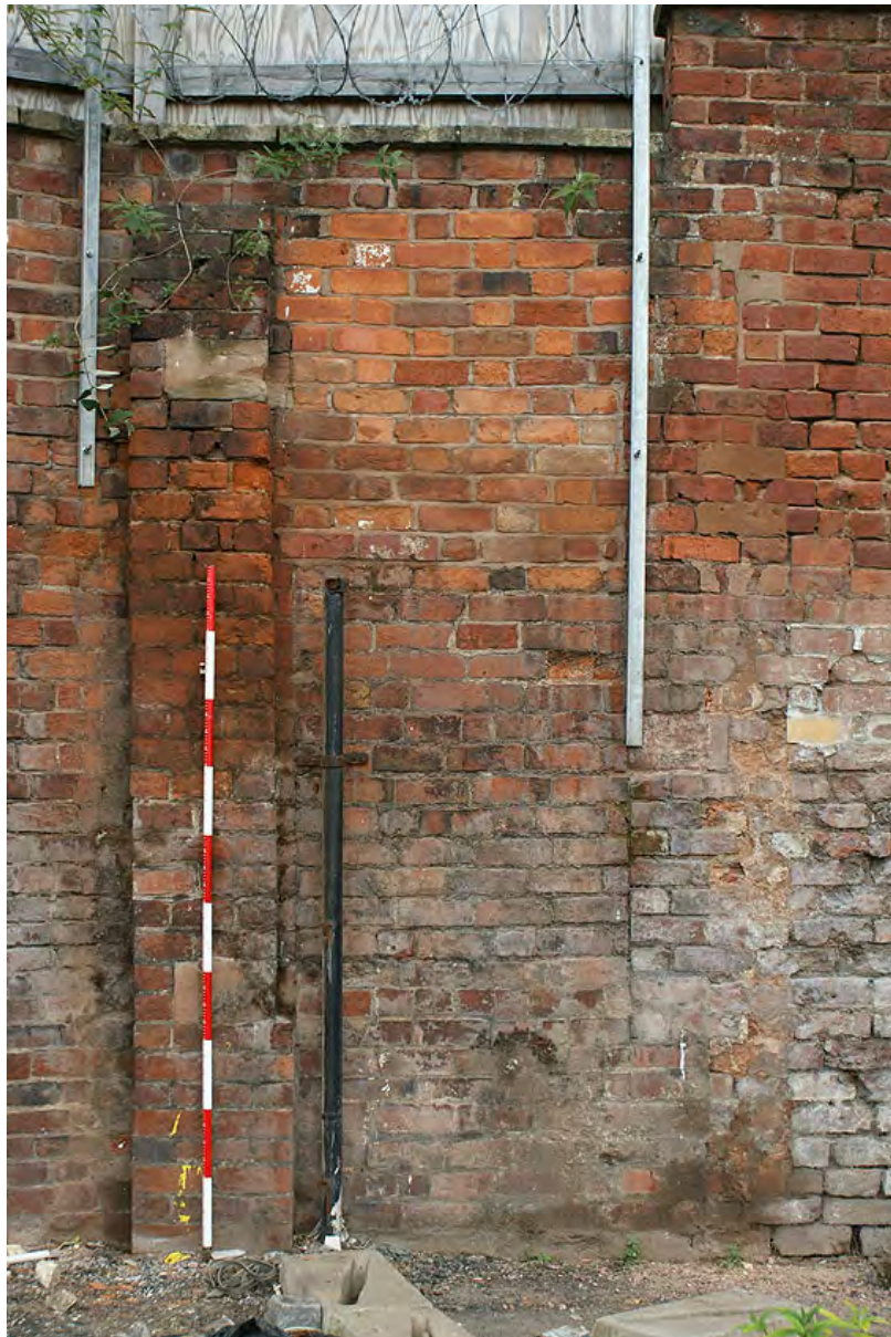
Plate 60: Wall section 4, blocked gateway
