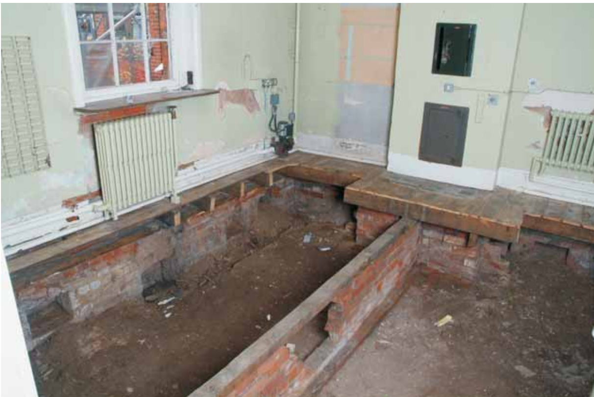
Plate 18.22: Building 18 – ground floor: east ward following removal of the floor showing traces of brick ducting, view to the northeast
