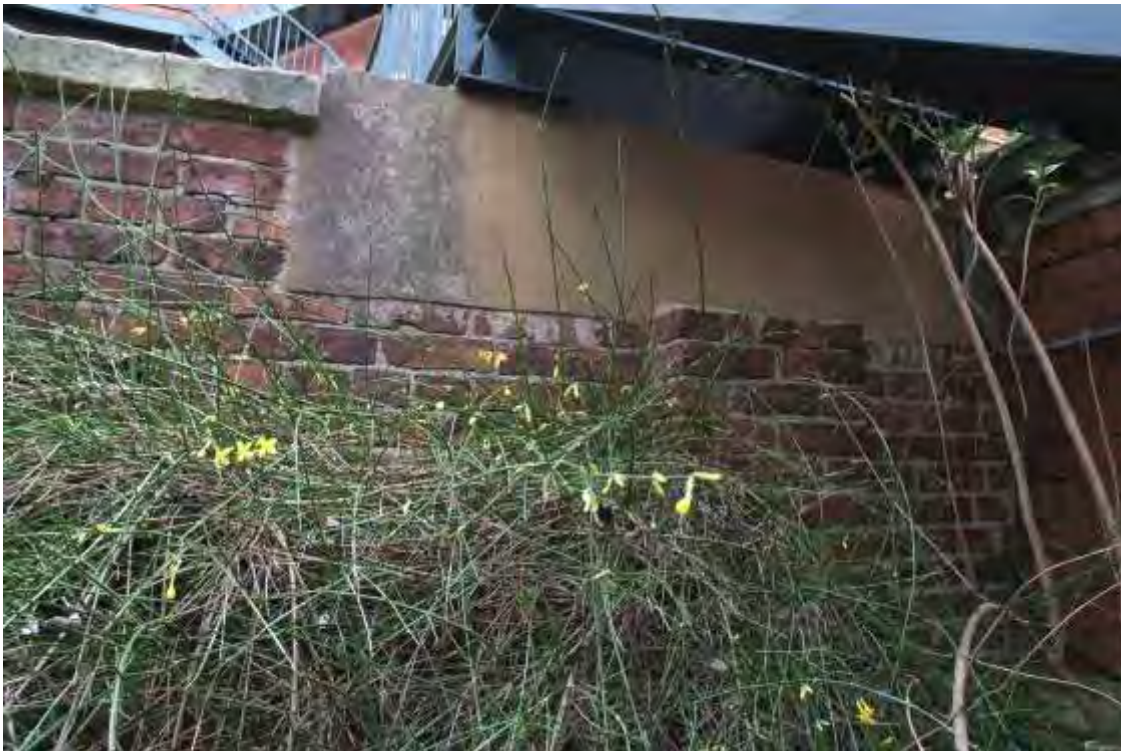
Plate 46.2: Building 46 –southern face to south of Building 36 showing concrete insert for fire escape, view to the northeast
