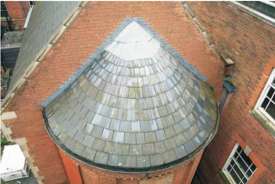
Plate 22.13: Building 22 – half conical roof of apse, view to the east
