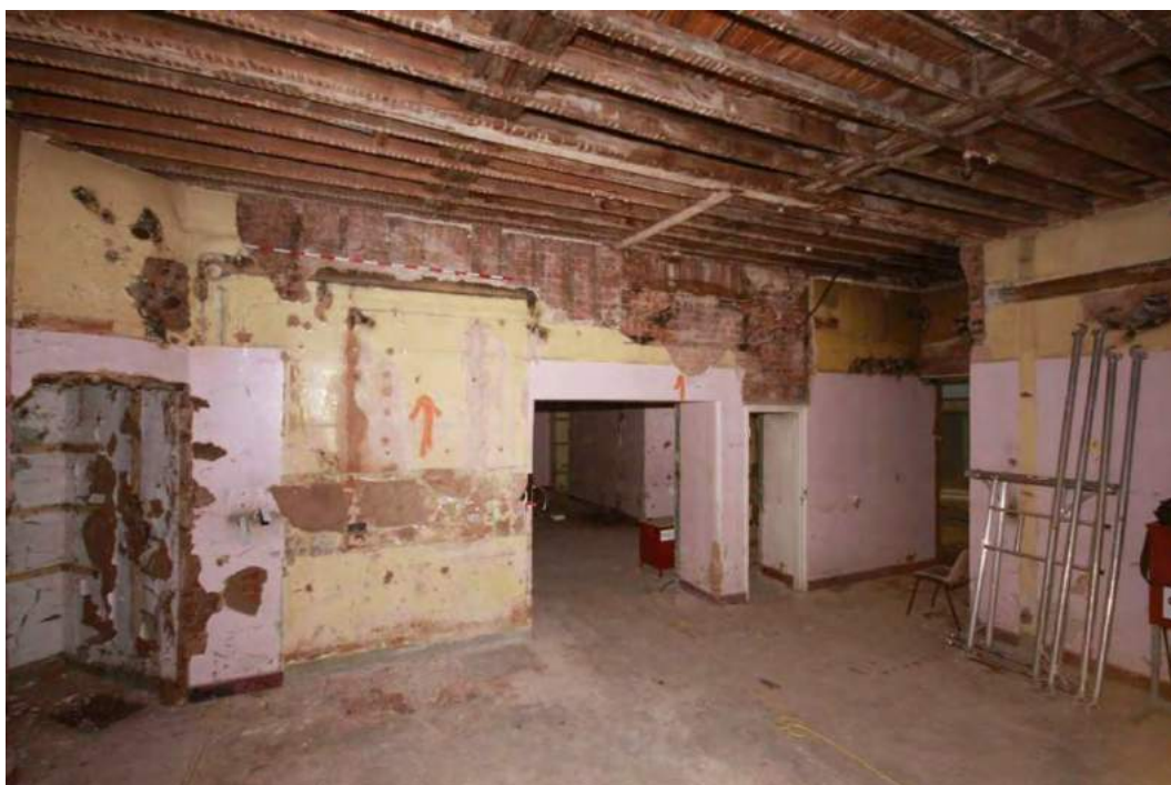
Plate 24.150: Building 24 (LGF): blocked openings in original western elevation of north wing (Building 24a) following soft strip, view to the southeast
