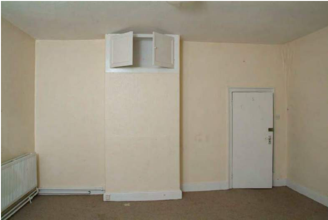
Plate 30.45: Building 30 (FF): bedroom in late 19th century extension to southwest wing showing inserted doorway through rear wall of original house, view to the north
