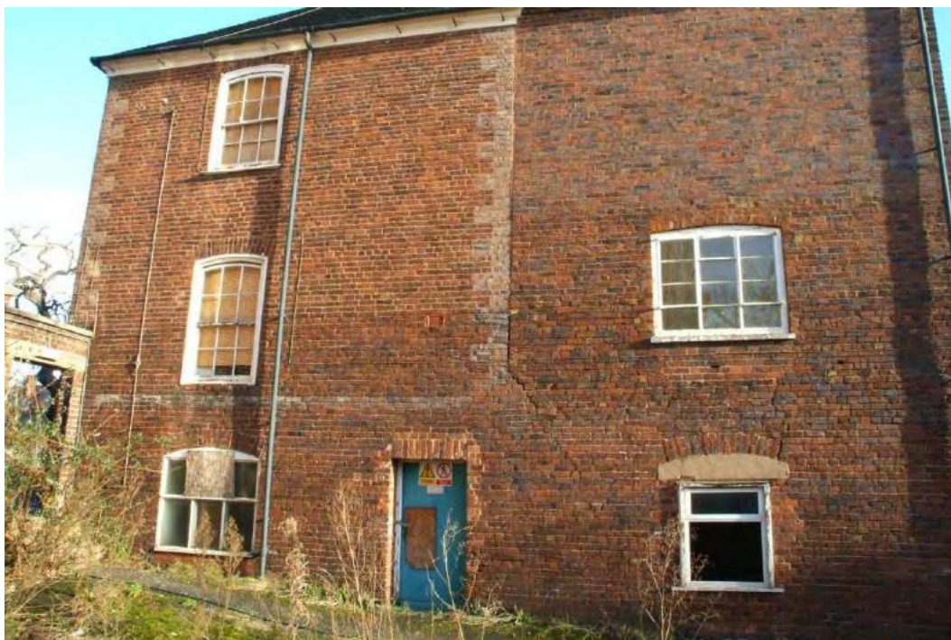
Plate 30.7: Building 30: detail of western elevation showing changes in brickwork, view to northwest
