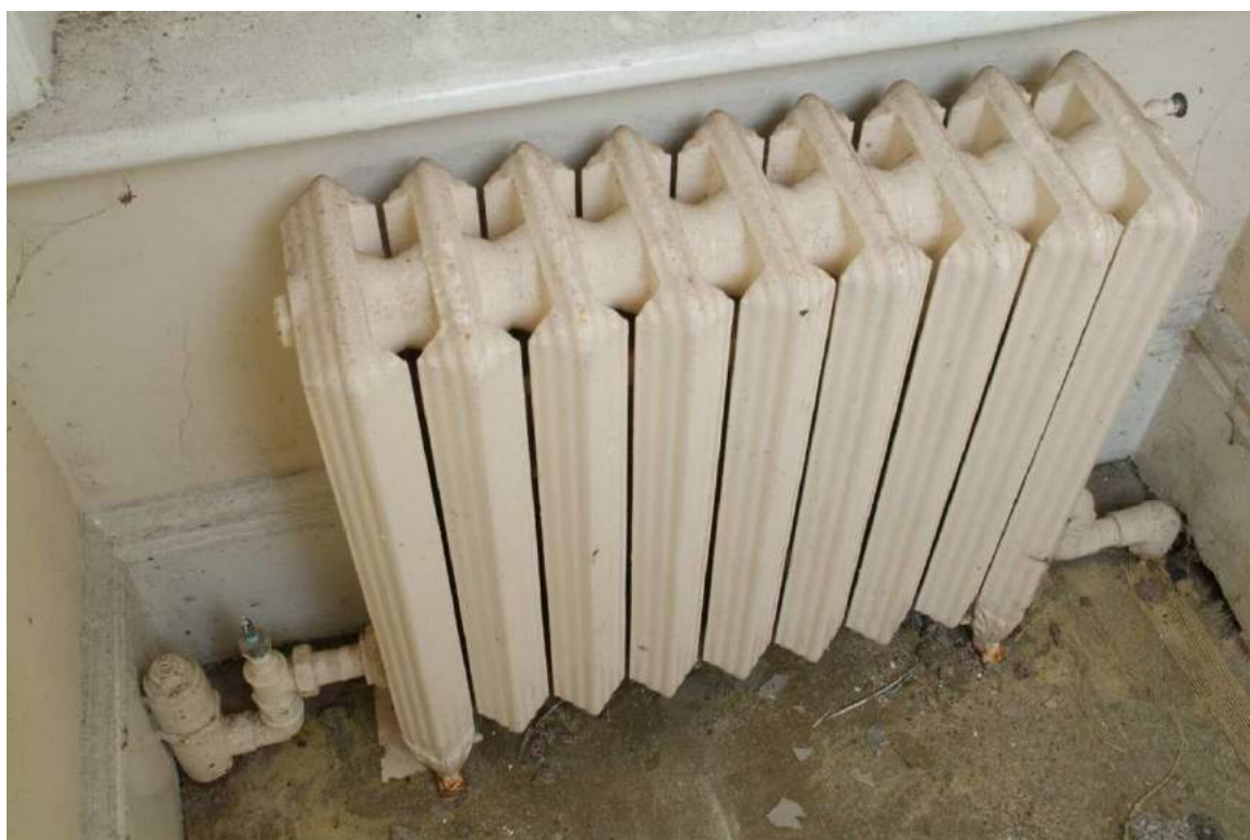
Plate 43.36: Building 43 – ground floor: detail of early 20 th century ideal radiator at west end of corridor, view to the south
