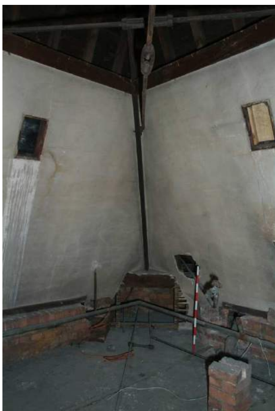
Plate 24.211: Building 24 (SF): lathe and plaster lining to roof of the southeast corner tower, view to the northwest
