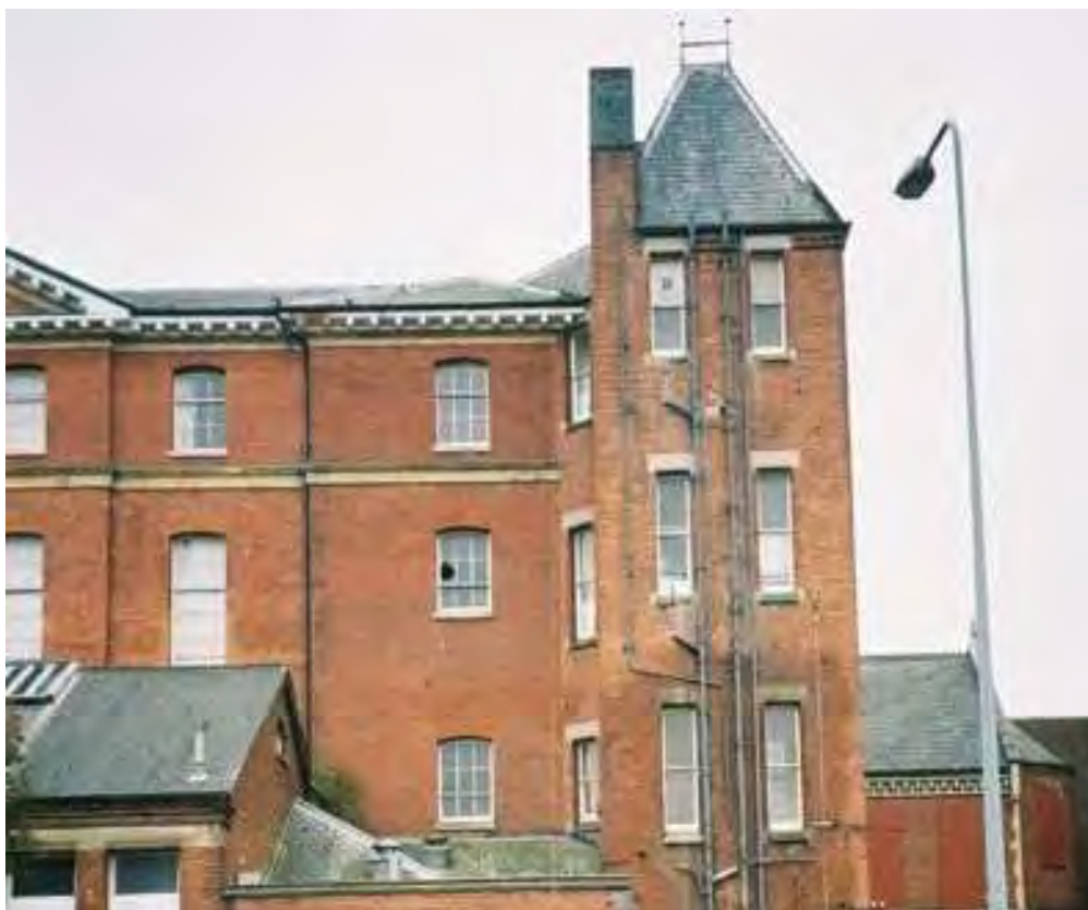
Plate 24.18: Building 24: detail of north western extension (Buildings 24b and 24g) showing vertical and horizontal changes in brickwork
