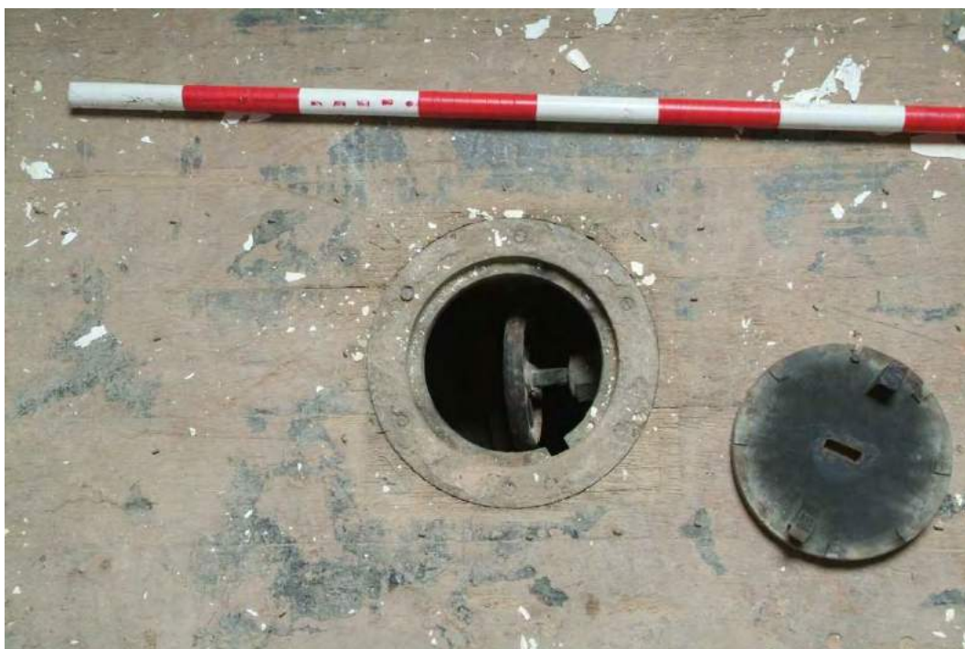
Plate 24.180: Building 24 (FF): detail showing brass stop cock opening in floor
