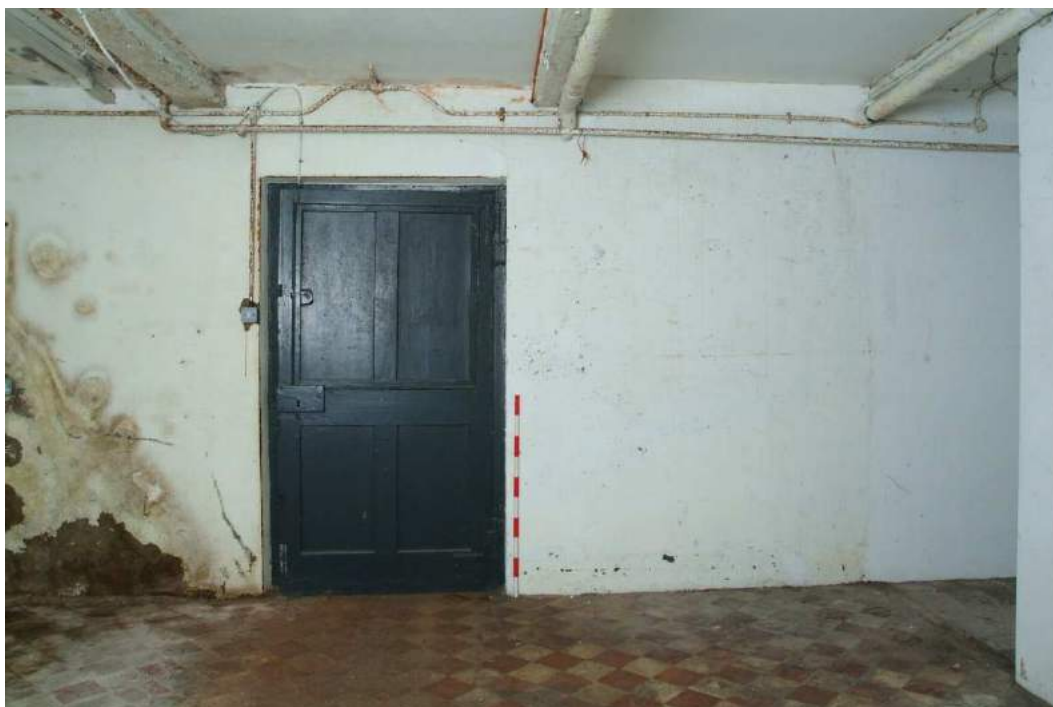
Plate 30.26: Building 30 (LGF): westernmost part of original basement showing inserted door and blocked fireplace, view to the south
