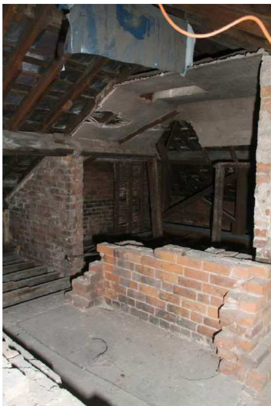
Plate 24.215: Building 24 (Roof Structure): former tank support structure in central part of roof, view to the southwest
