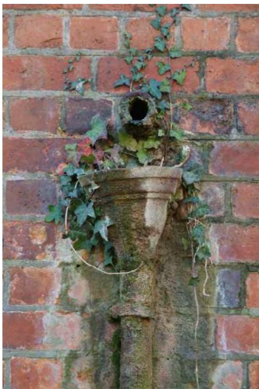
Plate 44.5: Building 44 – detail of rainwater hopper
