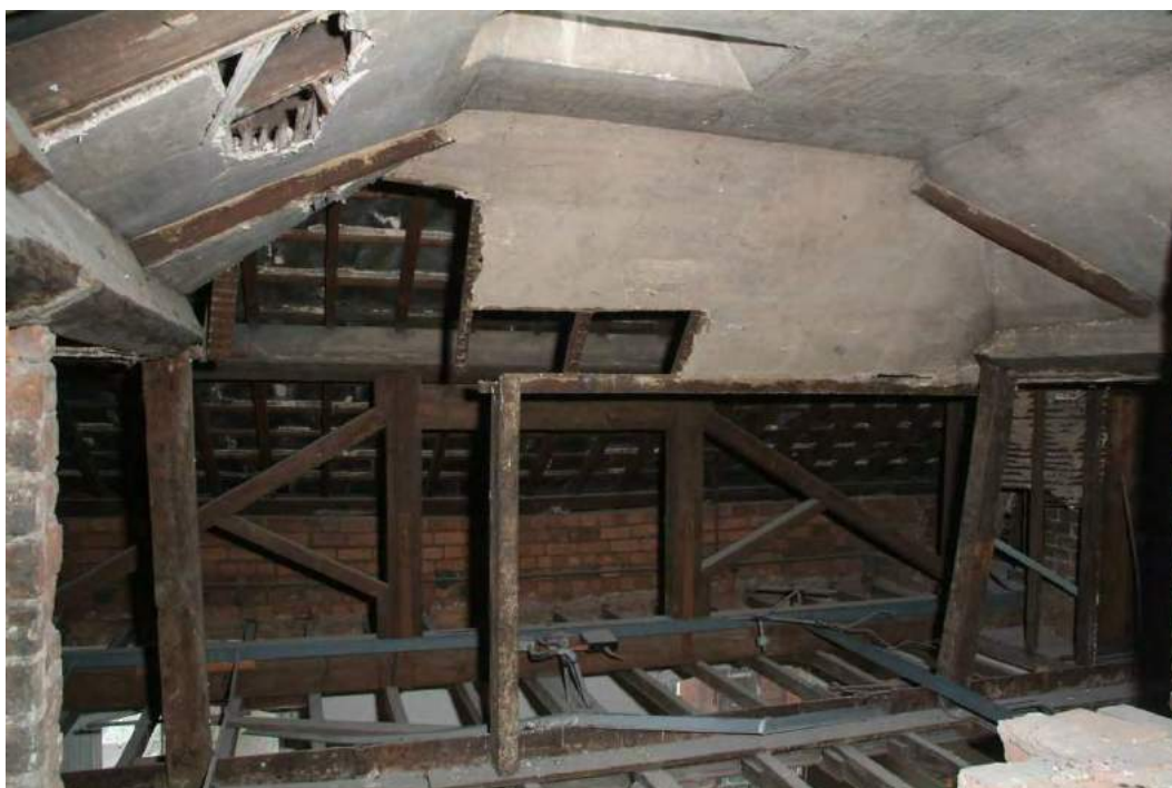
Plate 24.216: Building 24 (Roof Structure): lathe and plaster chamber in roof west of centre
