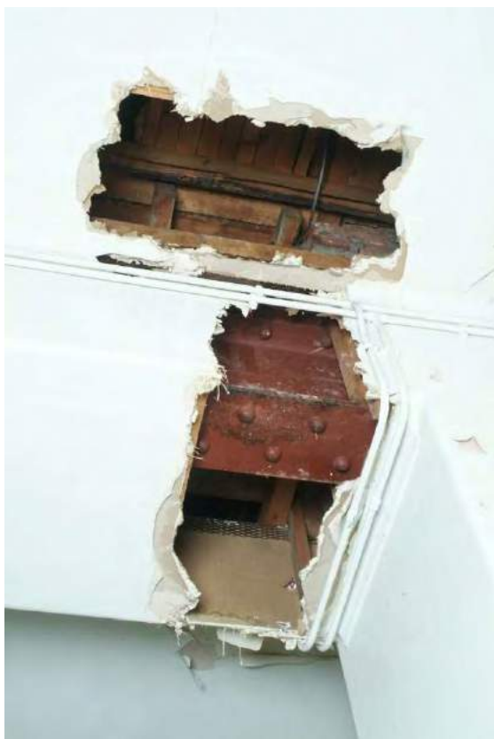
Plate 24.63: Building 24: Rushout Ward [Room 1.11] showing detail of riveted beam, view up and to the northwest
