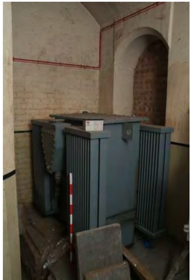
Plate 22.72: Building 22 (LGF): interior of the transformer room showing surviving transformer and brick lined sub floor ducting, view to the southwest
