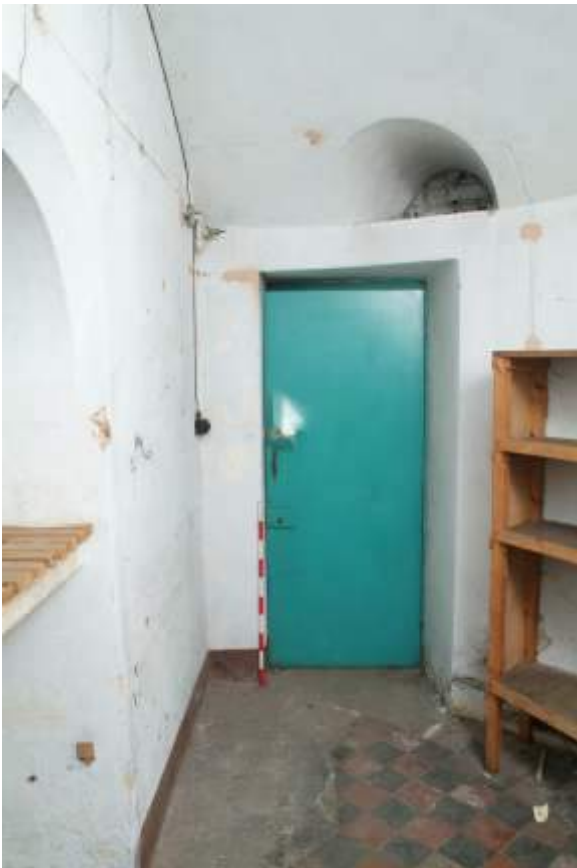
Plate 22.77: Building 22 (LGF): interior of apse showing inserted doorway, view to the south
