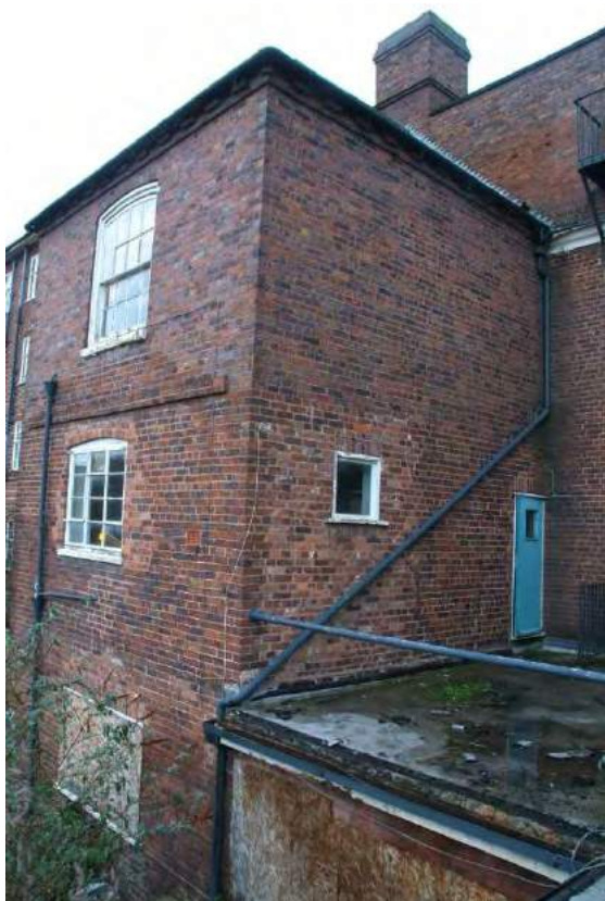
Plate 30.10: Building 30: detail of original southern elevation showing alterations to brickwork below stairlight, view to the north
