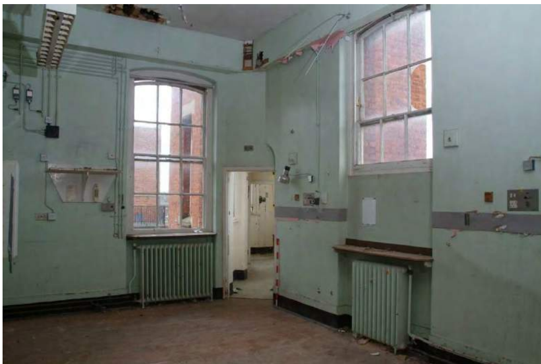
Plate 24.165: Building 24 (FF): west end of Garlick Ward showing short window (right), original window (left) and mis-aligned entrance to tower closet, view to the northwest
