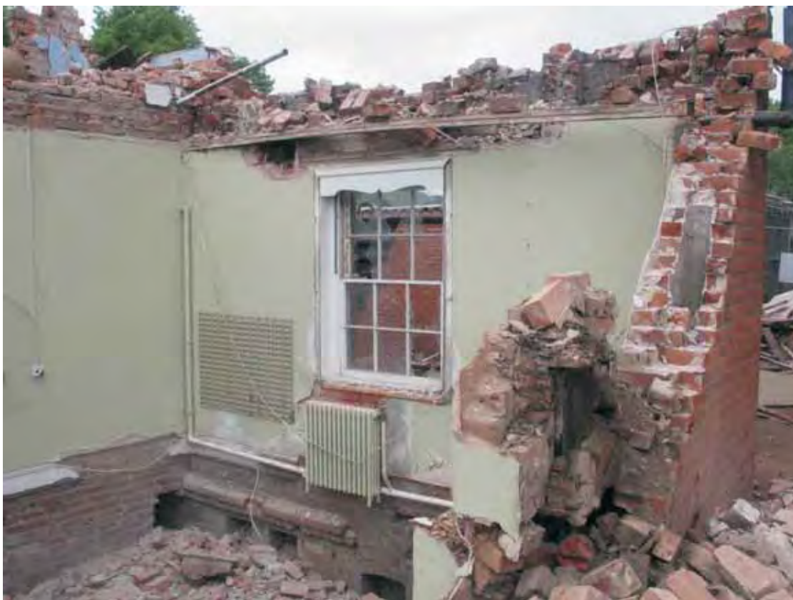
Plate 18.26: Building 18 – demolition of lower storey showing plaster lined shafts within the north and east walls, view to the northwest
