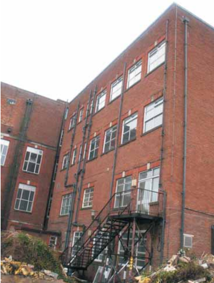
Plate 17.9: Building 17b – visible remnants of the VD Clinic showing western lavatory wing and change in brickwork above ground floor, view to the southeast
