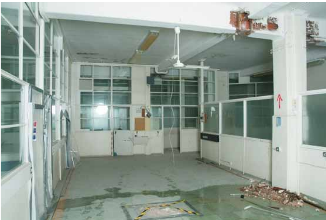
Plate 17.44: Building 17b – second floor: original metal partitions within the children's ward, view to the north
