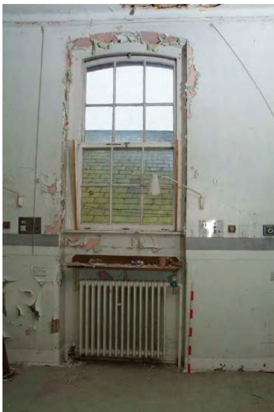
Plate 24.19: Building 24: detail of upper ground floor window in the northern elevation showing hopper light, view to the northwest
