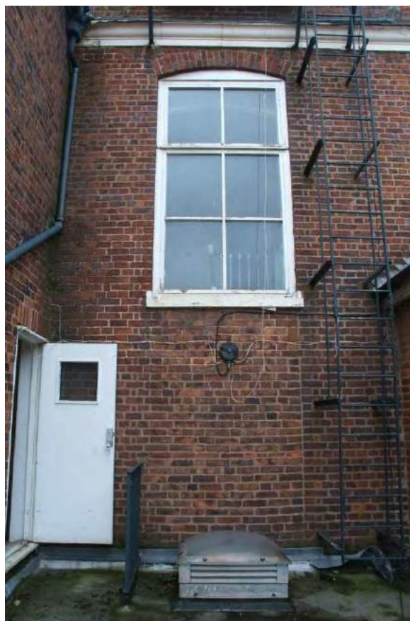
Plate 30.10: Building 30: detail of original southern elevation showing alterations to brickwork below stairlight, view to the north
