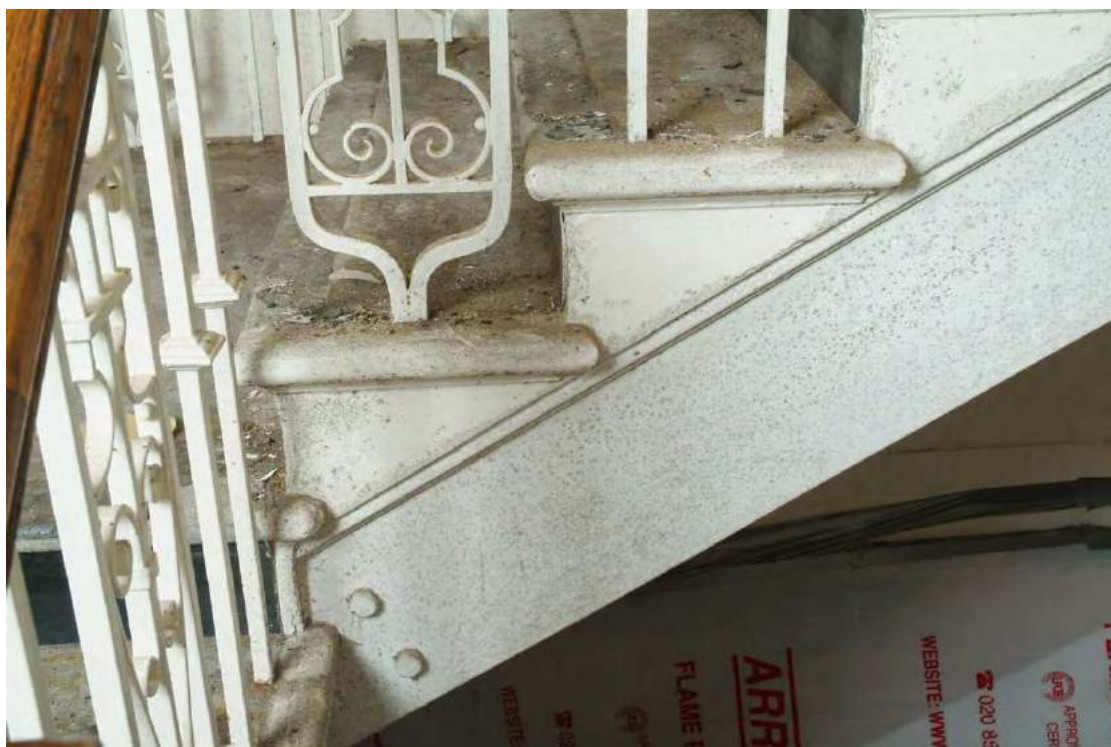
Plate 43.21: Building 43 – ground floor: detail of later strengthening to staircase
