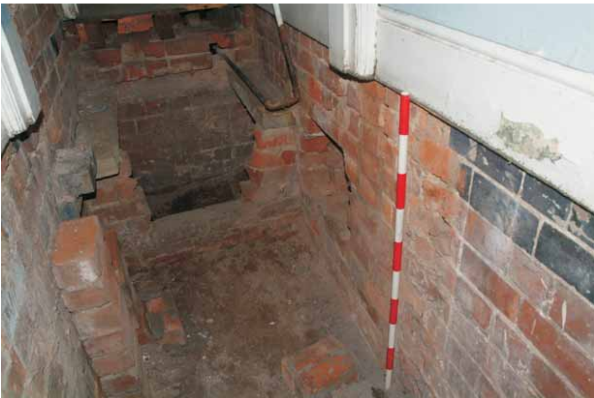
Plate 18.34: Building 18 – ground floor: foundation walls below floor in western closet wing showing truncated stub wall (left) and formerly external 'blue' brick, view to the northeast
