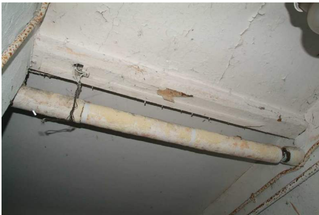
Plate 30.29: Building 30 (LGF): westernmost part of original basement showing remnants of service bell arrangement, view to the north
