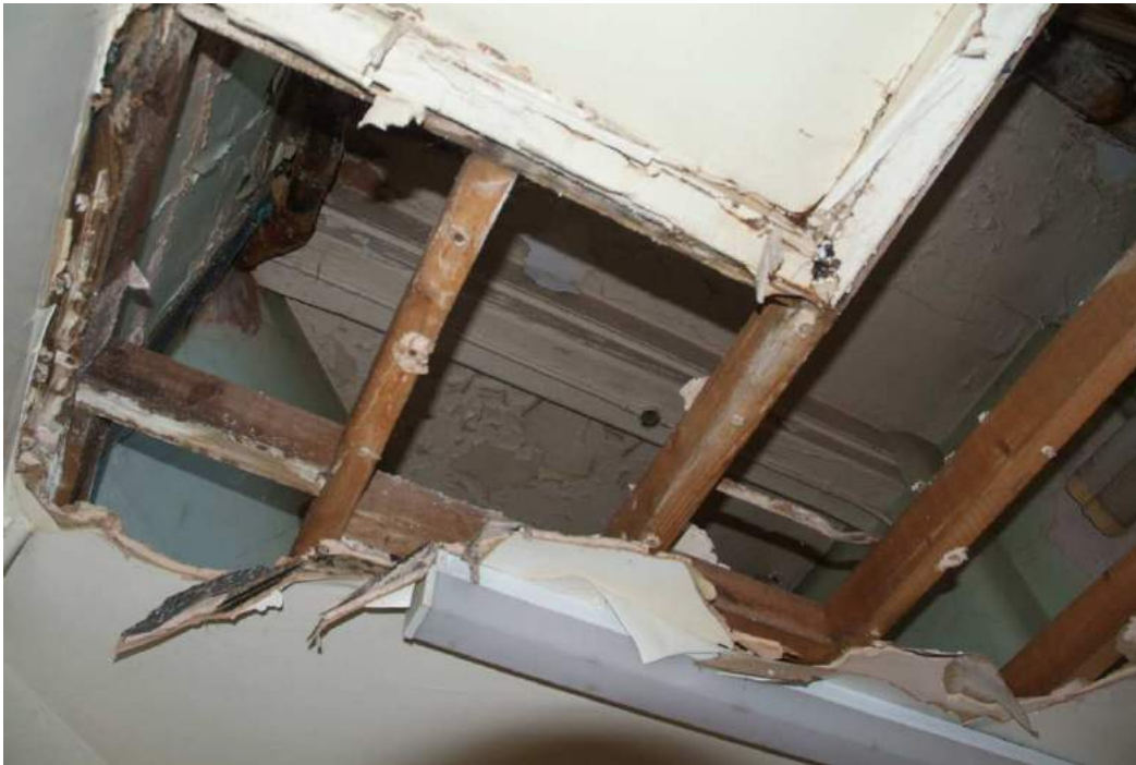
Plate 24.181: Building 24 (FF): exposed joist carrying 3rd floor over closet wing opening, view to the southwest
