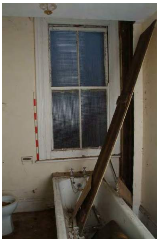
Plate 43.70: Building 43 - second floor: bathroom in central range showing original vertical pipe box, view to the east
