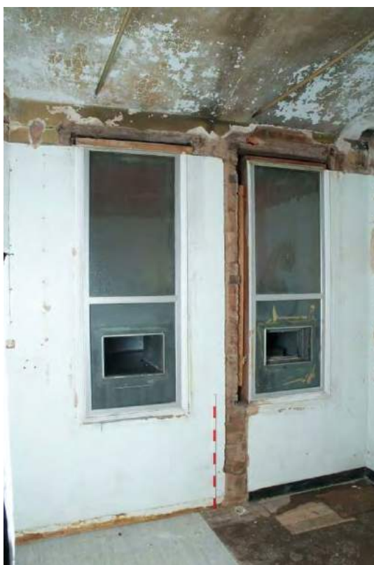
Plate 24.148: Building 24 (LGF): air ducts in modified original window openings, view to the southwest
