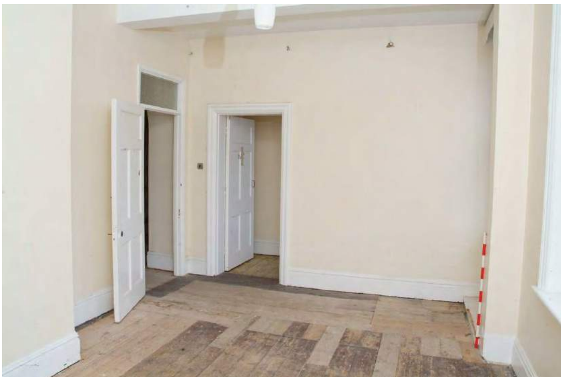
Plate 43.61: Building 43 - first floor: eastern bedroom showing line of former corridor and original communal entrance to the W.C., view to the north
