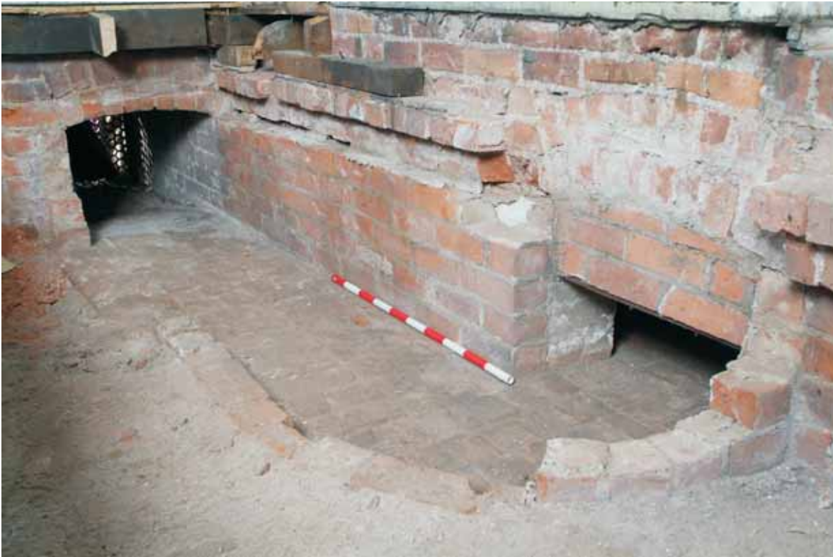
Plate 18.27: Building 18 – ground floor: main air inlet duct beneath duty room floor, view to the northwest
