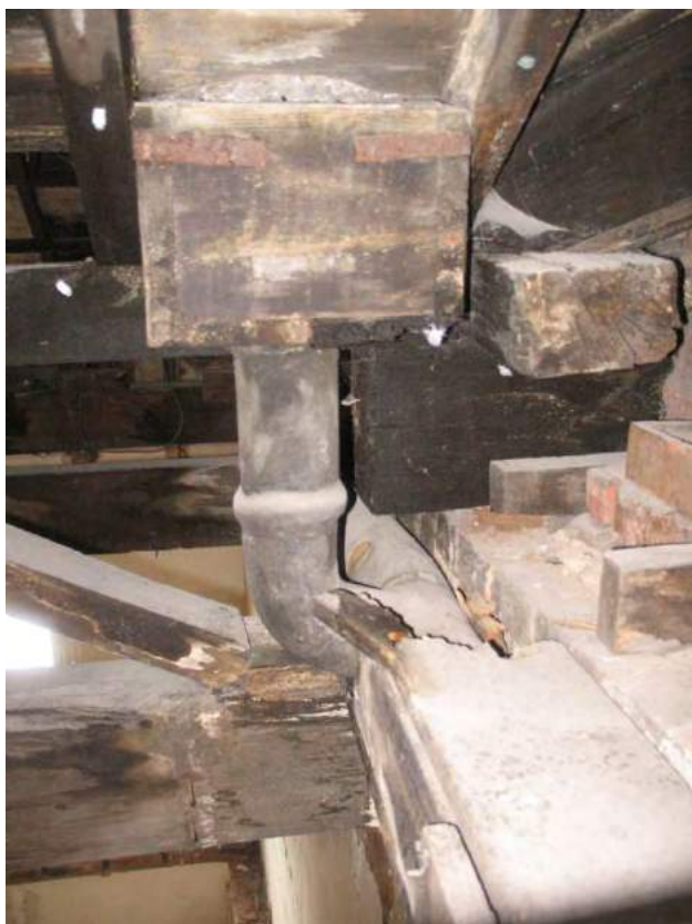
Plate 24.219: Building 24 (Roof Structure): internal lead rainwater hopper and pipe, view to the west
