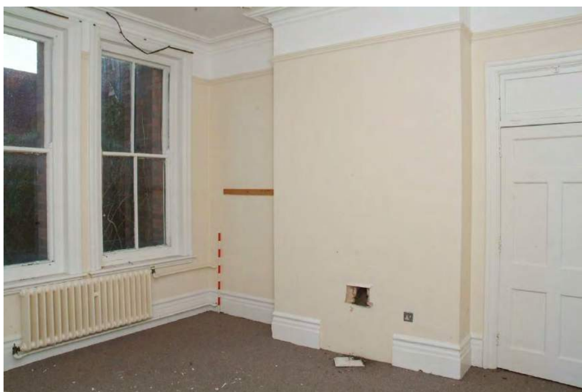
Plate 43.26: Building 43 – ground floor: living room showing blocked fireplace
