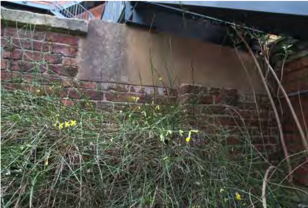
Plate 36.7: Building 36 – southern elevation showing 20 th century insertion of concrete foundation for fire escape, view to the northeast
