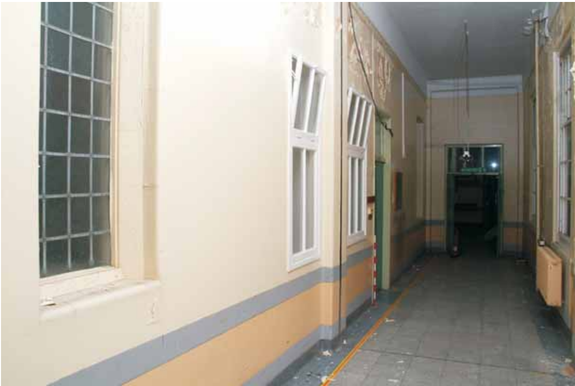
Plate 22.5: Building 22 – upper ground floor: later openings in former external southern elevation, view to the northeast
