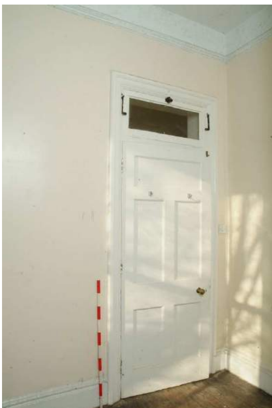
Plate 43.29: Building 43 – ground floor: typical original door and overhead to bedrooms in north and south ranges
