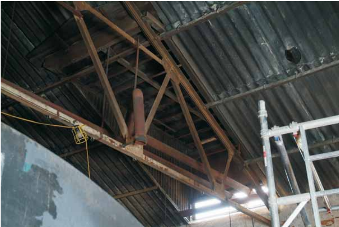
Plate 10.16: Building 10 – detail of roof trusses
