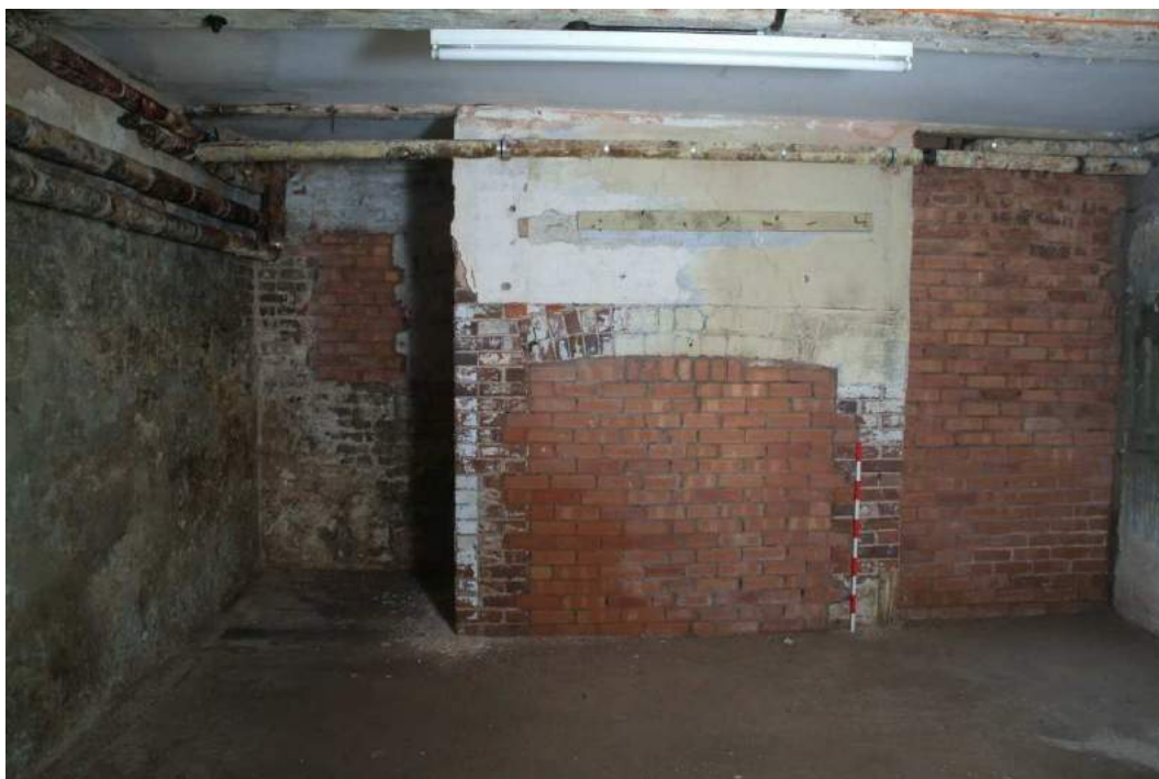
Plate 30.31: Building 30 (LGF): easternmost part of original basement showing blocked fireplace and window, view to the south
