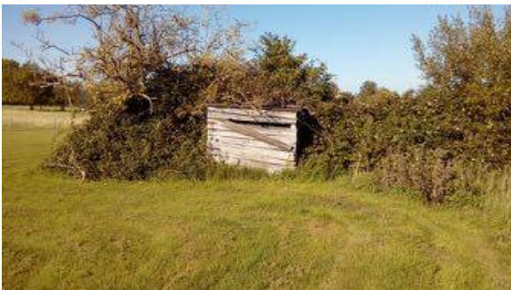
WSM 73457 South Elevation (all photos – Terry Woodfield)
