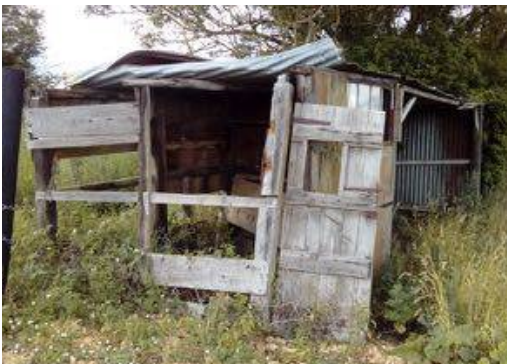
WSM 73085 East Elevation (all photos - Terry Woodfield)
