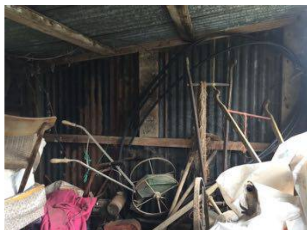
WSM 71080 Interior showing timber frame
