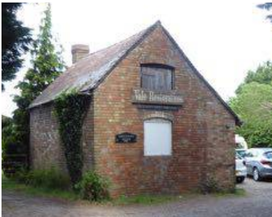
WSM 71729 South and East Elevations (all photos - Ken and Gill Pawson)
