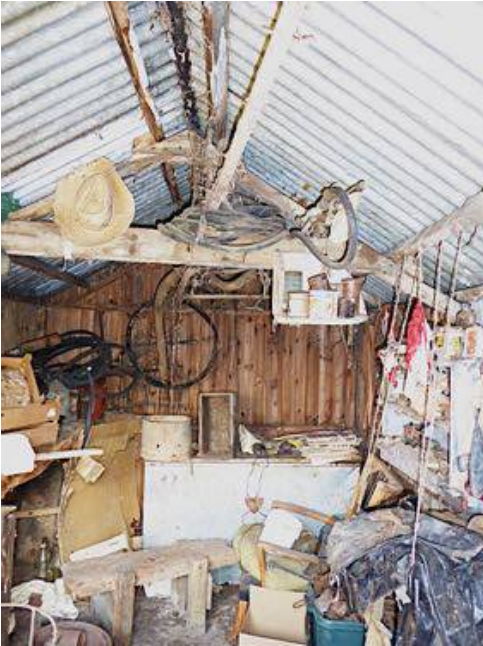
WSM 71124 Interior views, before restoration
