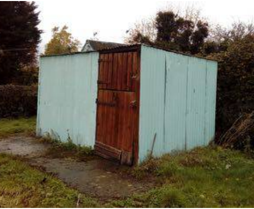
WSM 73551 South & East elevations (all photos – Terry Woodfield)
