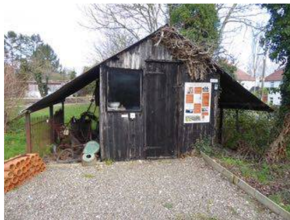
WSM 71124 After restoration
