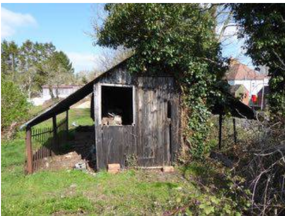
WSM 71124 Before restoration
