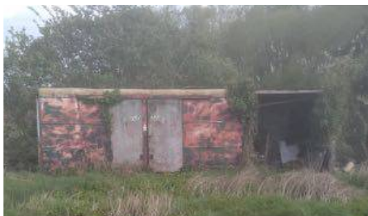
WSM 77576 South elevation (all photos - DA & JE Evans)
