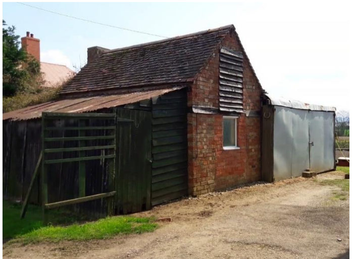
Photo 4: Brick construction with additional lean-tos
