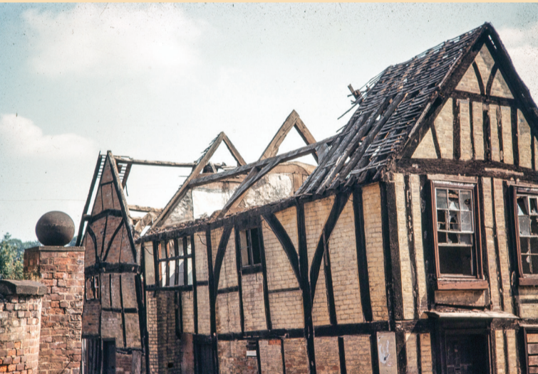
Below bottom: Chorley House roof detailing (© WCC Charles Archive)
