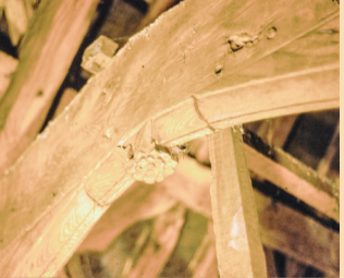
Left: Decorative timber mouldings and carvings inside the roof of 31-35 High Street (© WCC Charles Archive)
