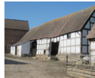
A mid 17th century, part timber-framed, part limestone rubble barn with four framed bays aligned east/west. There are cart entries on the south side only and a 19th century lean-to addition with a catslide roof adjoins the west elevation. Photo © Worcestershire County Council
