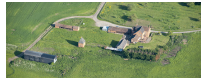
An estate farmstead, associated with Croome Court, with significant loss of traditional buildings. The 2nd Edition Ordnance Survey map records a large scale farm with three yard areas, two of which were covered. Photo © English Heritage. NMR.27699_20
