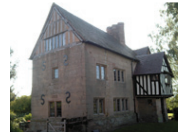
An early 17th century farmhouse in Stoke Prior. Timber-frame with painted brick and rendered infill, extended in painted sandstone ashlar. Photo © Worcestershire County Council
