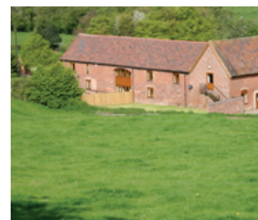
Brick early to mid 19th century buildings around a courtyard at Shelsley Walsh, looking towards a threshing barn built of weatherboarded timber frame. Photo © Worcestershire County Council
