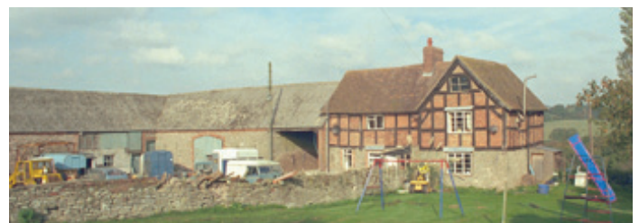
The farm buildings associated with this 17th century timber-framed house were rebuilt as a regular L-plan range in the early-mid 19th century. Adjoining the house is a throughway to allow covered access between the farmyard and paddocks to the rear; and attached to it on the left is a threshing barn and (in the left-hand range of the L-plan) a stable range. Photo © Worcestershire County Council
