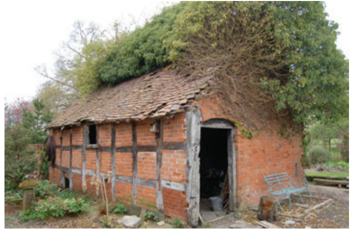
Single-storey cider house, Crowle. This is an extremely rare survival in timber frame. Photo © Worcestershire County Council
