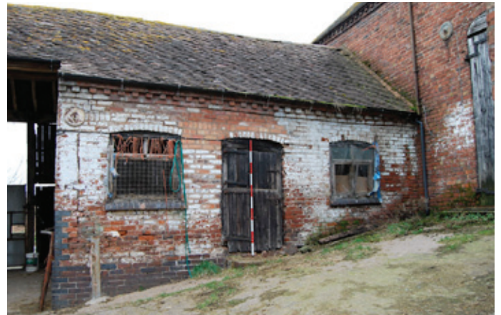
Mid 19th century brick stable with ventilated windows flanking the door, near Bewdley. Photo © Worcestershire County Council
