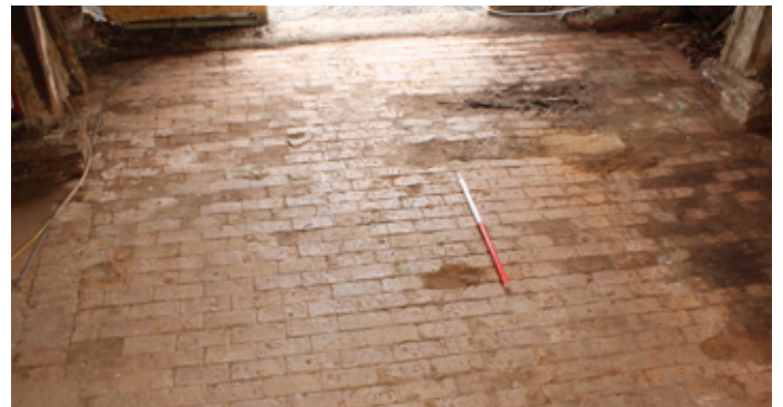
Threshing floors, either made of stone flags or brick (there are no records of timber floors), rarely survive. Photos © Worcestershire County Council
