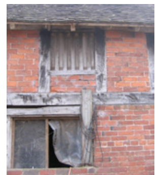
The ground floors of timber-framed cow houses were frequently replaced in brick, because cattle tended to kick out and damage walls. Note the pegs along the top of the horizontal timber but their absence along the bottom, indicating that the brick is original to this early-mid 18th century frame. Photo © Worcestershire County Council
