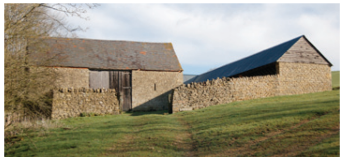
An outfarm near Conderton, comprising a threshing barn and a shelter shed facing a cattle yard. Photo © Worcestershire County Council
