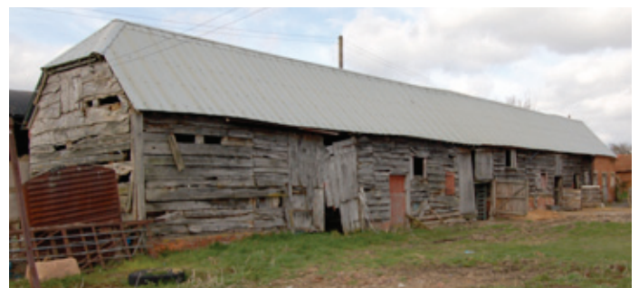
A combination barn in the Teme Valley, with integral cattle housing to the right. Photo © Worcestershire County Council
