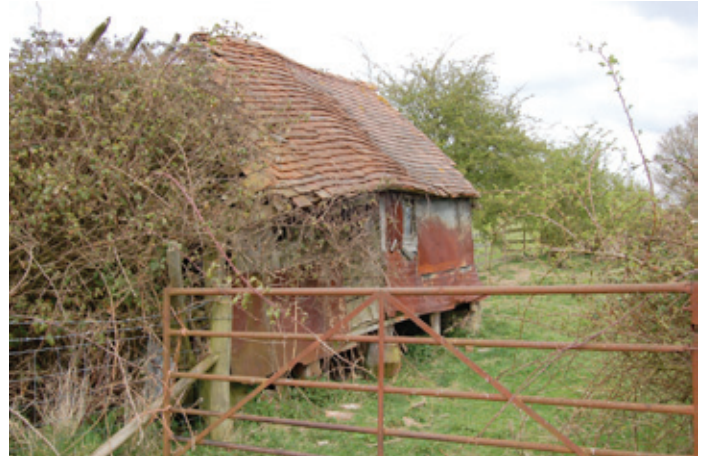
A fruit store at Crowle, raised above the ground to keep the crop dry. Photo © Worcestershire County Council
