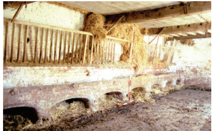
Stable interior showing a brick manger with tethering rings fixed to a wooden lip, the hay rack above tilted to enable hay to be forked into it through a gap along the side-wall from the loft above. Photo © Worcestershire County Council
