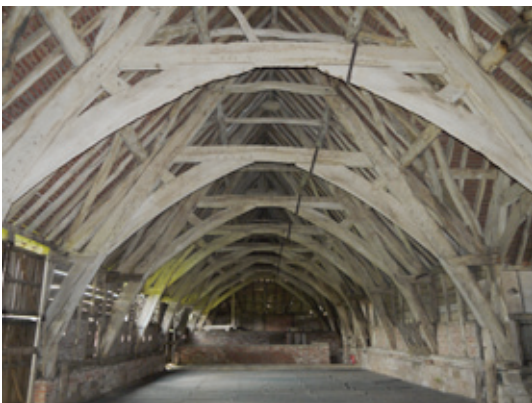
Leigh Court Barn at Leigh is listed at grade I. It was built in the 14th century to store produce for Pershore Abbey and is the largest cruck-framed structure in Britain. It has 18 cruck blades each made from a single tree. Photo © Worcestershire County Council
