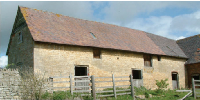
A two-storey cow house built of oolitic limestone. Note the typically broad doorways and openings to the hay loft. The doorway to the right is narrower and slightly taller, signifying that is the entrance to a stable. Photo © Worcestershire County Council
