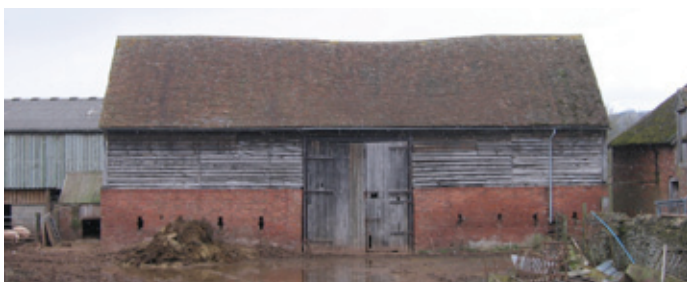
The use of timber frame set on a tall brick plinth is a common feature, as here on this mid 18th century five-bay barn near Stanford upon Teme. Photo © Worcestershire County Council
