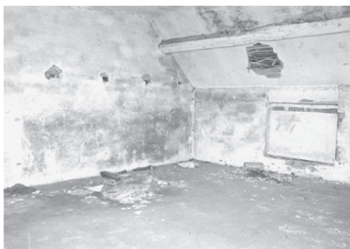
Plaster floor and walls to a cheese room at Birchensale Farm, Redditch. Photo © Worcestershire County Council
