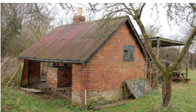
Old Ordnance Survey maps might show that orchards surround field barns which on inspection might reveal other functions. This open-fronted late 19th century building at Birlingham has a chimney stack which serves a copper. This was probably used to heat and soften withies for making baskets and in addition might have heated drink and food for orchard workers. Such modest structures are an integral and locally-important part of the county's historic orchards. Photo © Worcestershire County Council
