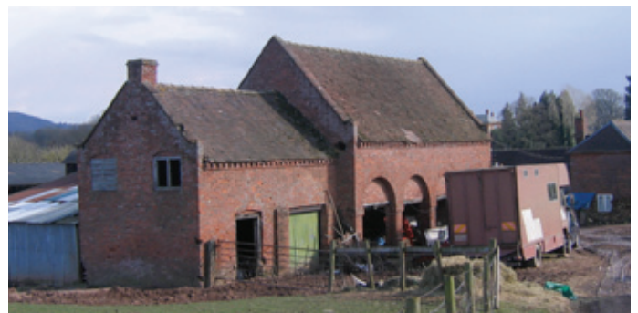
A mid-late 18th century brick cartshed with a first-floor granary. This is unusually decorative, and faces into a parkland landscape. Note the lower lofted building with a chimneystack to the left. Such buildings could have served as forges, but in this case the doorway is too narrow and it could have served as accommodation for farm workers. Photo © Worcestershire County Council
