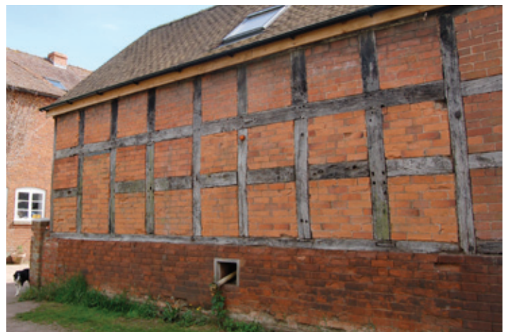
Square-panelling, as here at Suckley, is a characteristic feature of timber framing in western England. Photo © Worcestershire County Council
