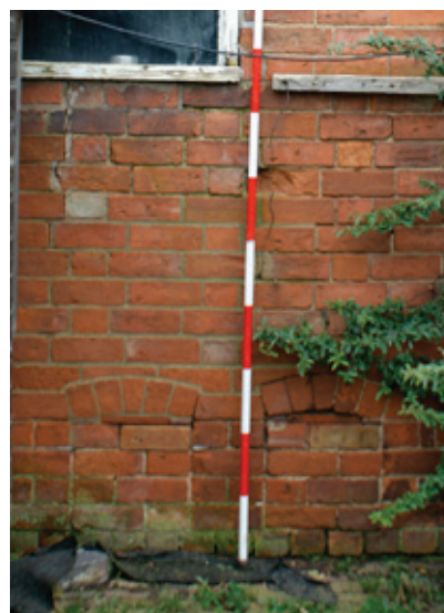
Blocked openings to a hen house. Photo © Worcestershire County Council
