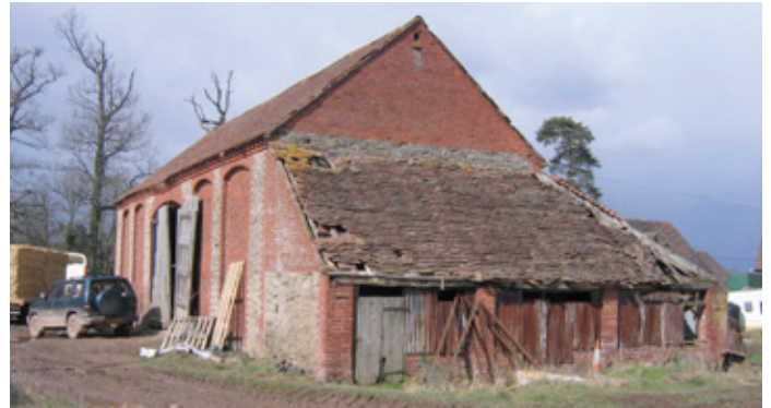
Looseboxes added to an early 19th century threshing barn. Photo © Worcestershire County Council
