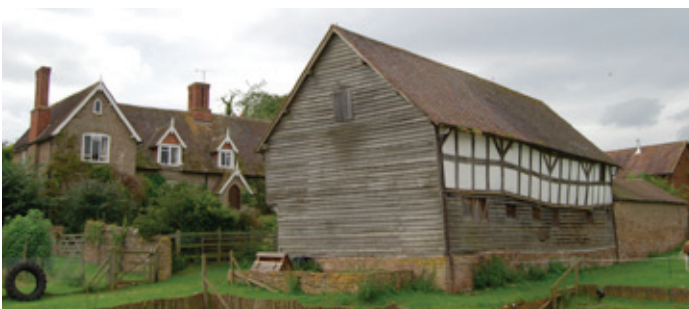
A cow house, possibly combined with a stable, at Stoke Bliss. This is an exceptionally rare example of an animal house of 18th century or earlier date – the use of square panel framing was used in the West Midlands into the 17th century. Photo © Worcestershire County Council
