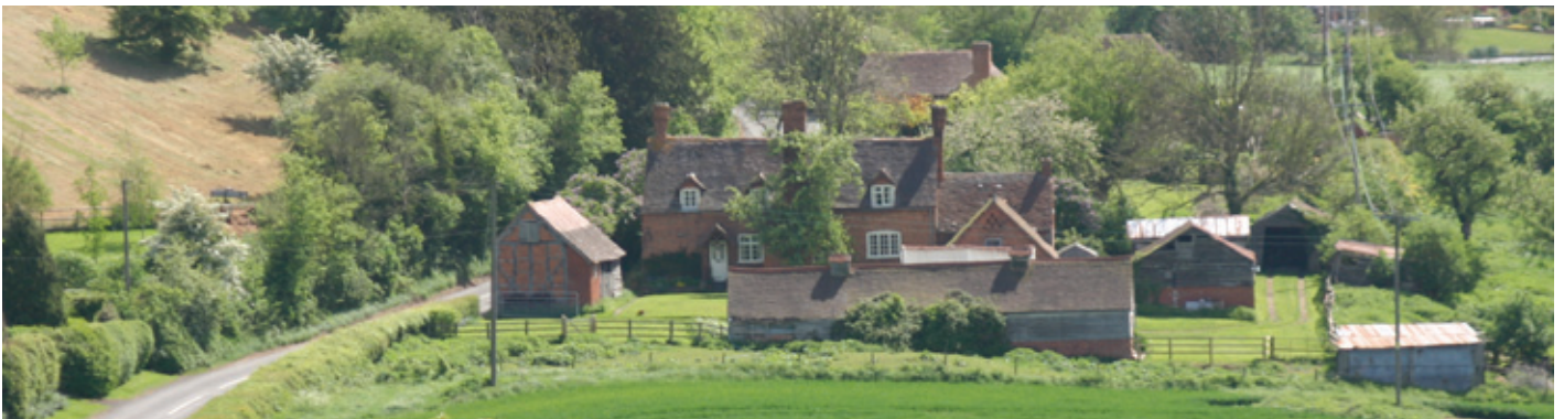
Loose courtyard plan with detached buildings to three side of the yard. Photo © Peter Gaskell
