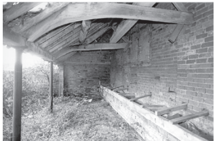
Shelter shed interior with rare surviving wooden manger. Photo © Worcestershire County Council
