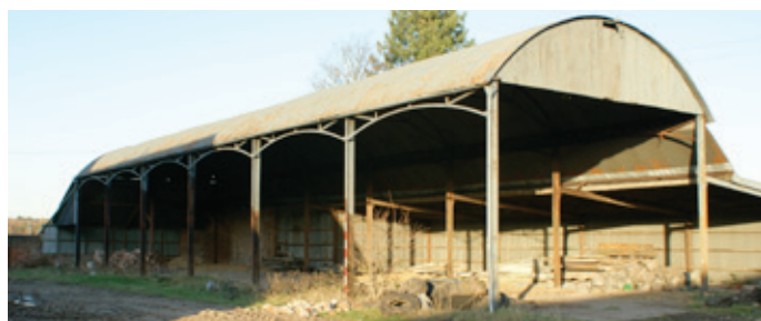
Dutch barn near Kidderminster. Metal-framed example. Photo © Worcestershire County Council
