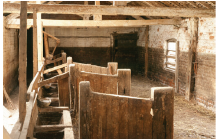
Traditional stalls of the type depicted here (note the feeding passage to the left) were replaced from the early 20th century in order to conform with hygiene regulations. They are increasingly rare. Photo © English Heritage/ Mike Williams
