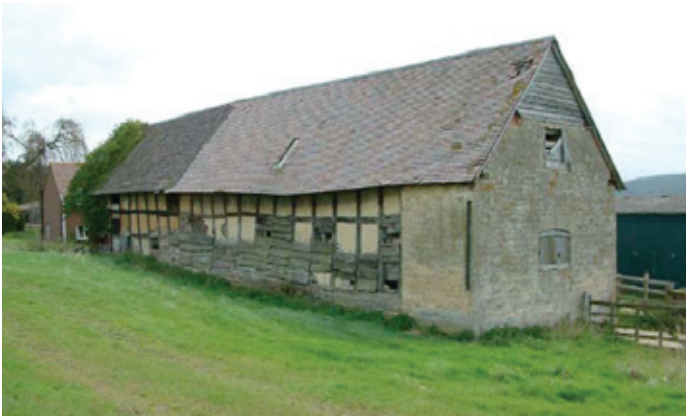
This timber-framed cow house with its hay loft at Grafton is an exceptionally rare example in a national context. It is attached to an L-shaped and cruck-framed house. Photo © Worcestershire County Council
