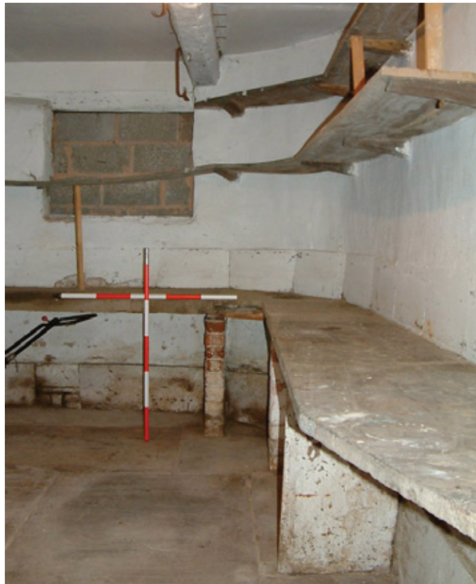
Cool storage and surfaces were provided in dairies by slate shelves supported on brick or stone piers or arches. Photo © Worcestershire County Council
