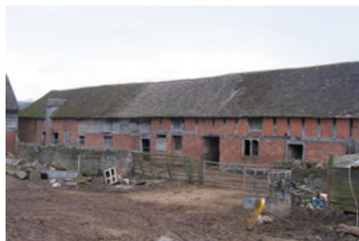
A very rare surviving example of an 18th century timber-framed cow house, with, to the left adjoining the barn, a stable with a gabled loading door to the loft. The ground floor was originally built in brick. Photo © Worcestershire County Council
