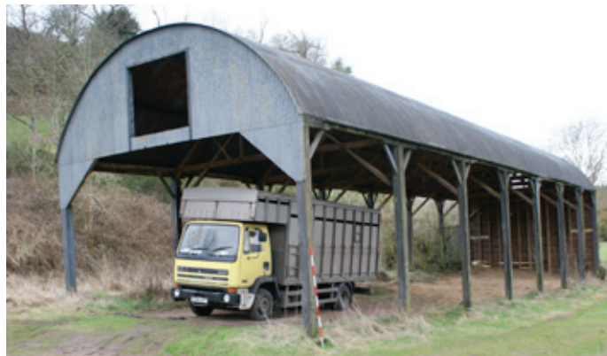
Dutch barn near Bewdley. Late 19th century example built of timber. Photo © Worcestershire County Council
