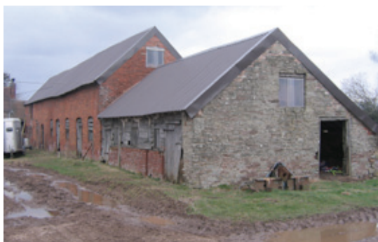
Cow houses were frequently extended and remodelled from earlier cores. At first sight this comprises an early to mid 19th century brick-built two-storey cow house with a hayloft, extended with a stone lias open-fronted shelter shed since infilled. It in fact has an 18th century or earlier timber-framed core. Photo © Worcestershire County Council
