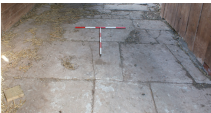
Threshing floors, either made of stone flags or brick (there are no records of timber floors), rarely survive. Photos © Worcestershire County Council
