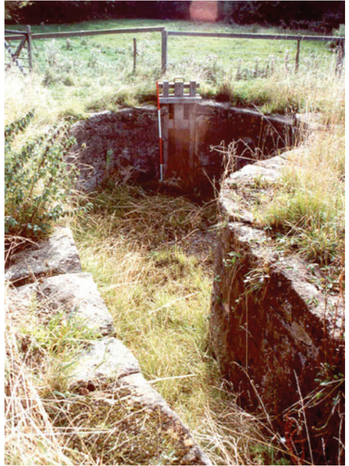
Sheepwashes typically incorporate a leat, a sluice with gate, a pool and usually a ramp to enable sheep to walk out of the pool. They can be teardrop-shaped, as here, circular or square: all were well-built of stone or brick. Examples are rare, as many have been filled in or completely lost after they went out of use. Photo © Worcestershire County Council
