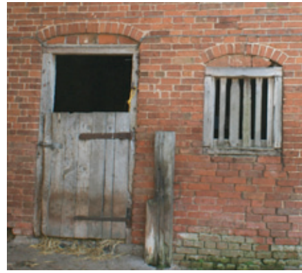
Stable door and ventilated window. Photo © Worcestershire County Council
