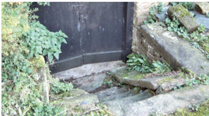
Steps to a cider cellar where the barrels would be stored. Stone ramps either side of the steps aided rolling the barrels in and out of the cellar. Photo © Joan Grundy
