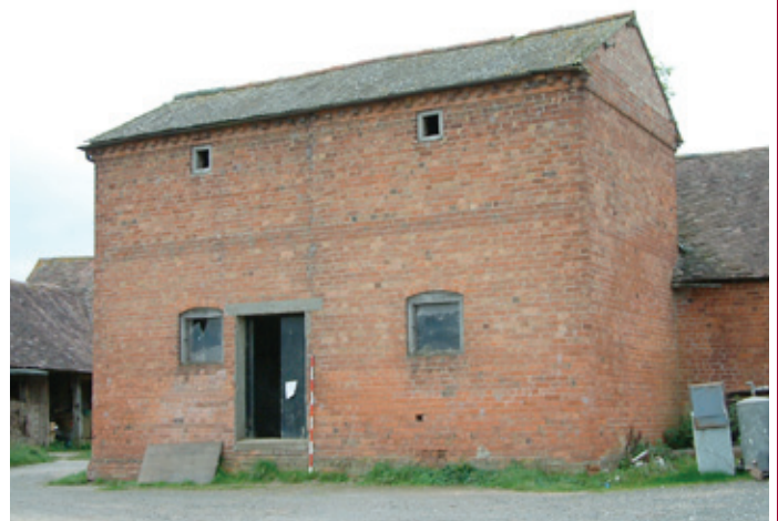
Stable, hayloft and granary (Building 3) from the north west. Photo © Worcestershire County Council
