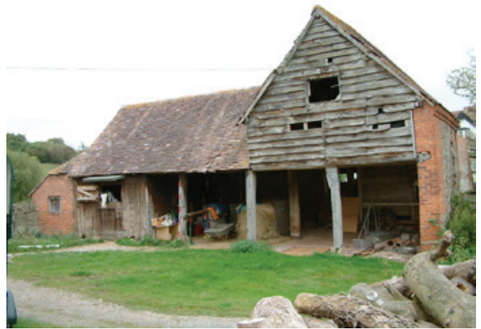
West elevation (Building 2) showing timber posts of shelter shed. Photo © Worcestershire County Council
