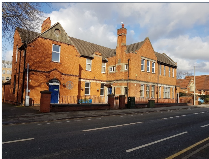
Image 6: Masonic Hall (former Unionist Club) 21 Easmore Road
