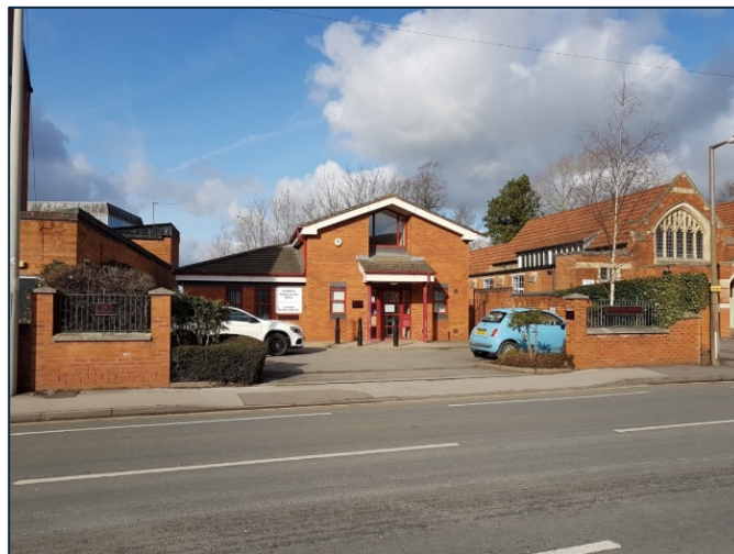
Image 49: Redditch Registration Office, 29 Easemore Road
