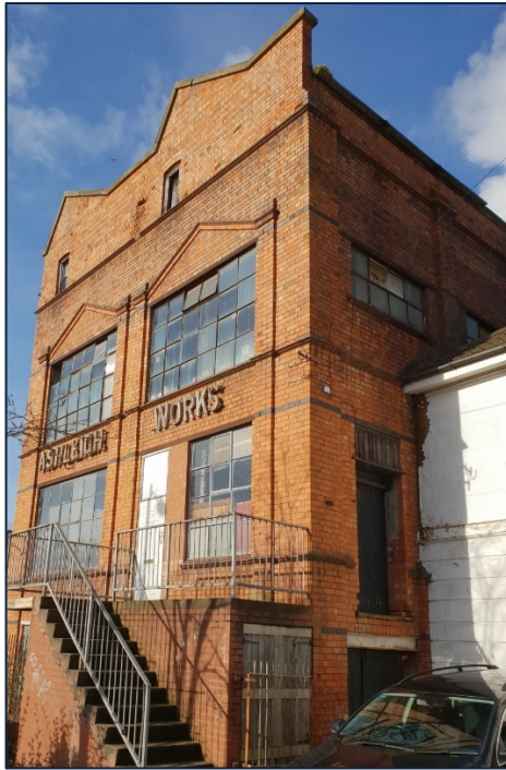
Image 3: Ashleigh Works, Bromsgrove Road
