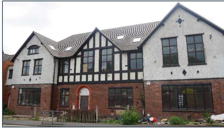
Image 52: The former St. Stephen's Church Institute and Redditch Central Mosque, Easemore Lane
