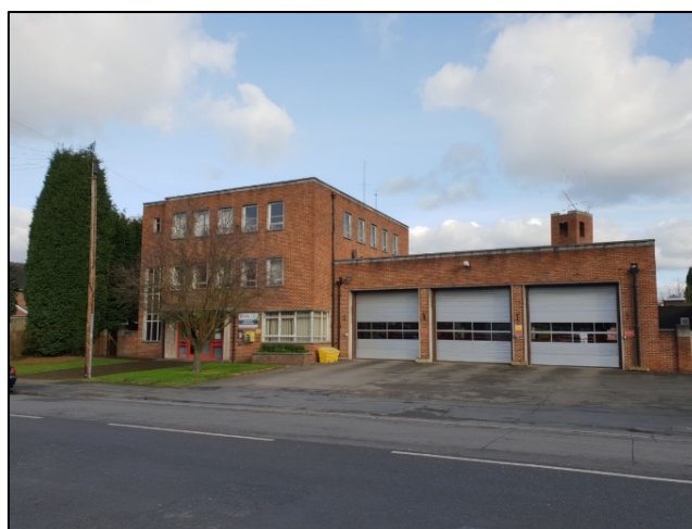
Image 41: Fire Station, Redditch
