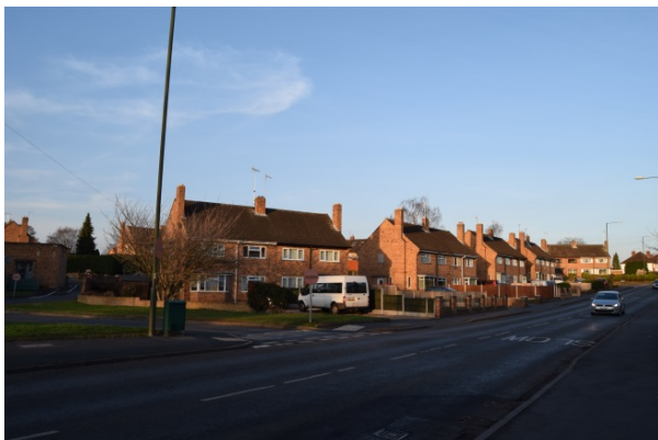
The south facing aspect of the former police houses.
