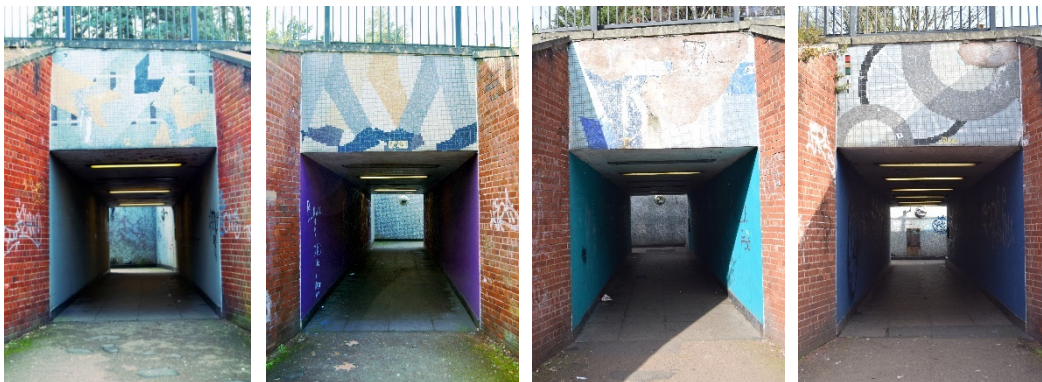
The four panels now in a poor state of repair.
