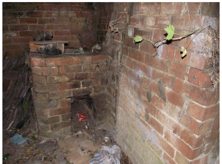
Brick fireplace with metal bowl above for heating water
