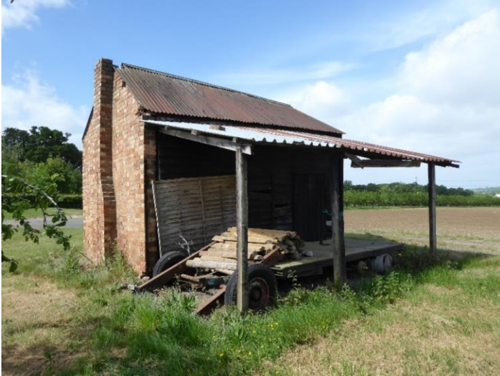
Wooden hovel with brick end wall, chimney and covered side
