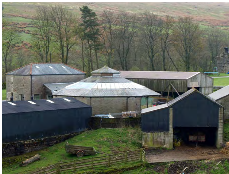
An unusually innovative example of an inter-war cowhouse in the Yorkshire Dales, its circular plan enabling cattle to be centrally milked by machine. © Jeremy Lake
