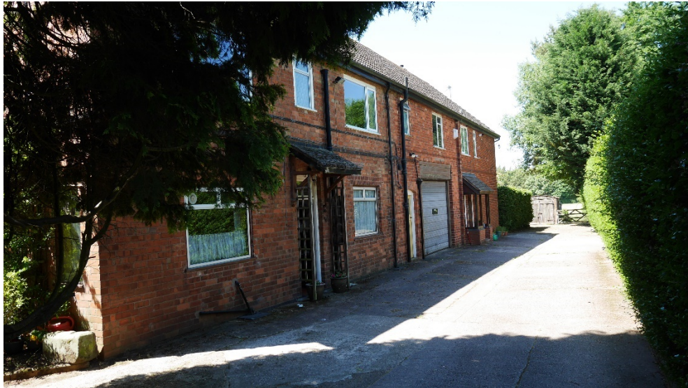
Extended cottage residence at Plot 7 of the Woodrow Farm Small Holdings Estate.
