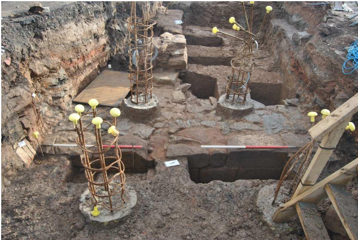
Figure 6: Remains of the early 17 th century bridge disturbed by modern piles, Upton-upon-Severn
