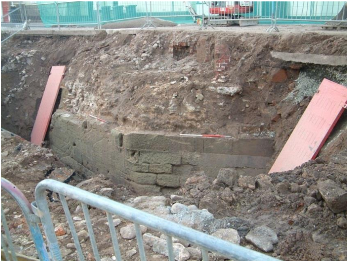
Figure 8: 15 th century bridge abutment, Bewdley
