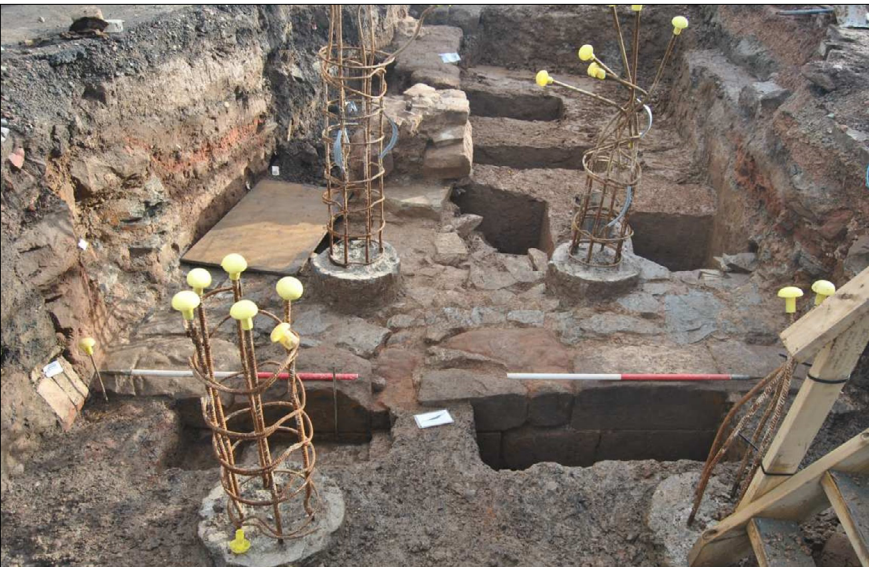
Figure 22: Post-medieval stone bridge with wall 8106 in the foreground; 1m scales; view east
