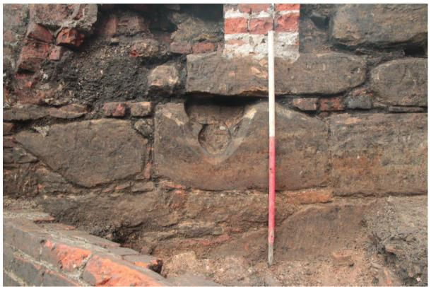
Plate 15: Detail of the late medieval tracery stonework reused in the curtain wall extension. Looking south, 1m scale
