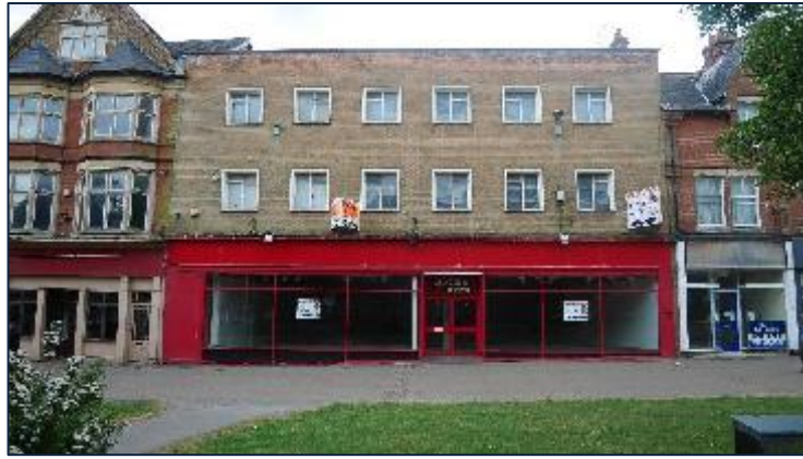
Image 18: Former Woolworths, Market Place
