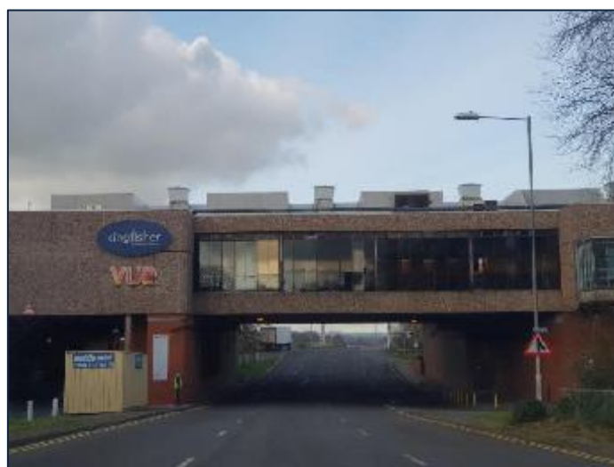
Image 31: Kingfisher Centre car park bridge
