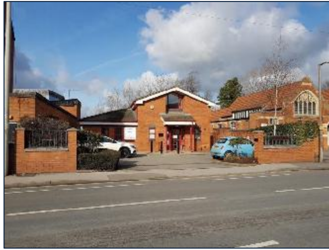
Image 49: Redditch Registration Office, 29 Easemore Road
