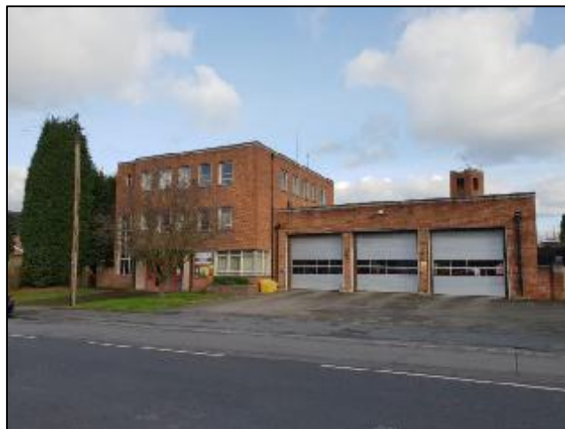
Image 41: Fire Station, Redditch
