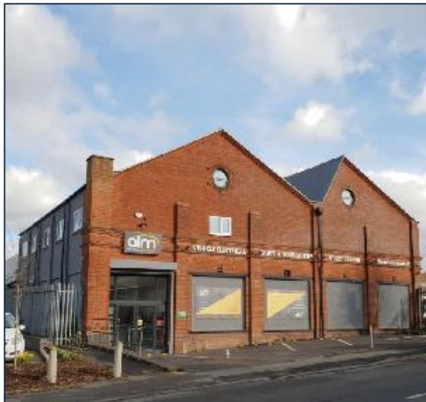
Image 1: Royal Enfield Building, Hewell Road (now ALM)
