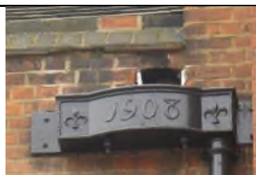
On a gutter head
