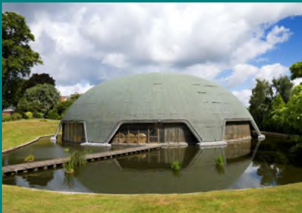
Left: The Edinburgh Dome at St. James Girls College in Malvern was listed at Grade II in 2009 for its innovative method of concrete construction. The dome was designed by Michael Godwin and is a 'parashell' concrete structure. John Faber of Oscar Faber acted as the engineer. The construction company Norwest Holst bought the sole rights to market the system in England but only two were ever constructed. © Historic England Archive DP138177
